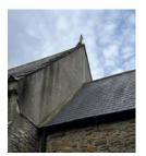
As recorded in the previous QI, the stone cross on the chancel/nave gable is damaged. Consideration should be given to repairing/replacing it.
