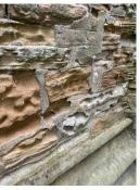
External walls are sandstone masonry. There is evidence of 'pocket' erosion to individual stones: very typical of stone sourced in Durham. This rate of erosion can be slow and it is likely the stone has appeared in this state for some time. There is evidence of indented stonework repairs. Earlier re-pointing at lower levels was carried out using a hard cement mortar which has caused serious erosion. In the upper levels where cement pointing has not been used the stonework is surviving better.
