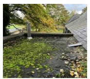
The Community room/boiler room roof is finished in built up felt. Vegetation growth has colonised part of the roof. In time, this can degrade the felt. This should be removed and the surface kept clear in the future. As noted previously, the felt could be nearing the end of its useful and should be monitored.
