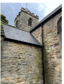
Where the pointing has a high cement content it stands proud of the stonework which erodes behind. There is abundant evidence of this. The hard cement mortar should be removed and the stone work repointed using a lime mortar.
