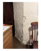
The vestry adjacent to the Chancel is in a reasonable state of repair apart from the north wall return at the door opening where rising and penetrating damp is affecting plasterwork.
