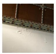
As noted in previous inspection there is evidence of blistering plaster/paintwork at high level north wall of Chancel. Check flashings/gutter joints, etc. externally at the change in roof pitch from Chancel to Vestry roofs.
