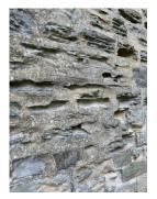
Full repairs of the stonework in a single project may be a daunting task. However, consideration should be given to a phased approach beginning with repointing near ground level, removing the hard mortar which is standing proud and indenting seriously eroded stonework. The phasing could be done to suit funding, eg a project in each year of the next quinquennial.
