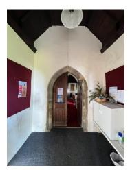
The north and west wall within the porch has loose C friable plaster. The defective plaster should be hacked off and replastered with a lime plaster.
