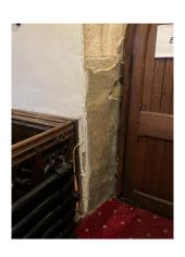
The surface of the stonework to the surround to the south porch door both within the nave and porch is losing its surface. This was noted in the previous inspection. Historically this has been partially repaired with a thin render smear, but this is coming away in part. Loose render surfaces should be removed and friable stone brushed back to allow the stone to dry out and breath.
