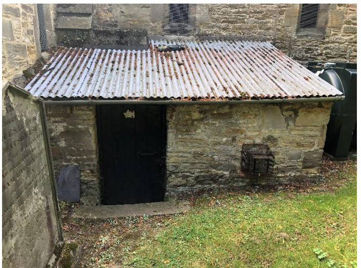
Fig. 5 (IMG 8321) Boiler house lean-to
