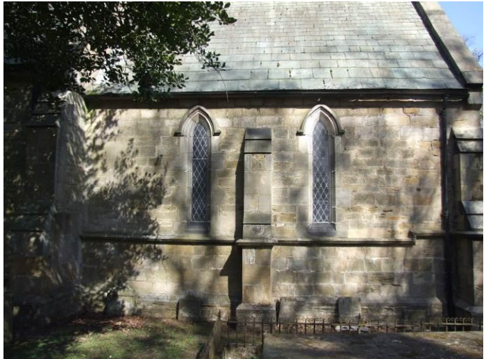
Fig. 8 (IMG 1307) Note some stone face erosion to left hand side of eastern buttress, may relate to gutter overflow
