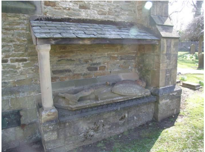
Fig. 14 (IMG 1323) Figure with roof protection and new stone column (west end of Church): some slate damage
