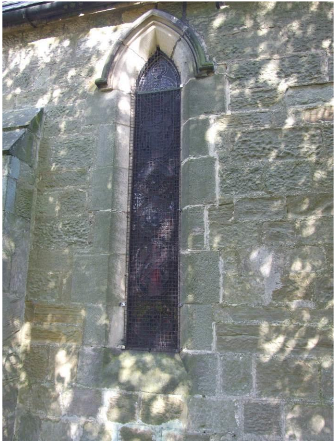
Fig. 7 (IMG 1304) Corroding but not yet pattern staining window guards
