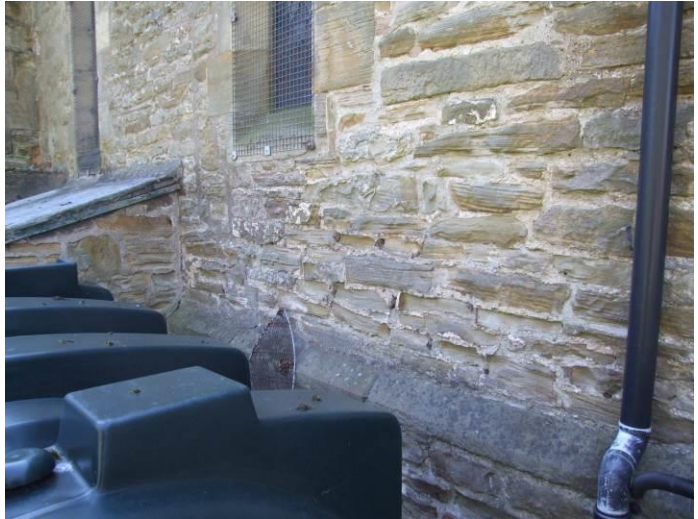
Fig. 12 (IMG 1320) Eroded stone faces and residual pointing to north elevation of chancel
