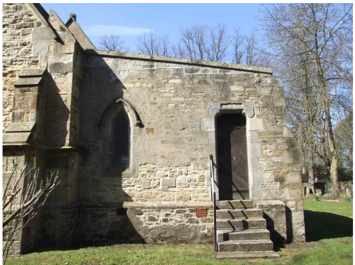
Fig. 9 (IMG 1311) Varied pointing character to east wall of vestry
