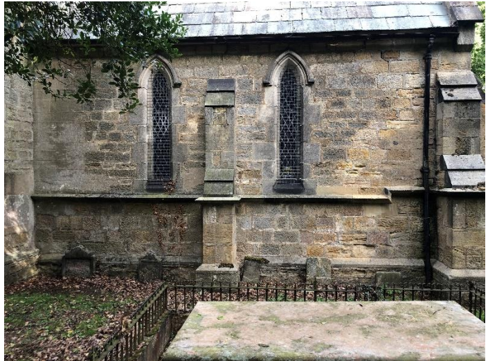
Fig. 3 (IMG 8299) Pattern cracking/face erosion from eaves to drip course
