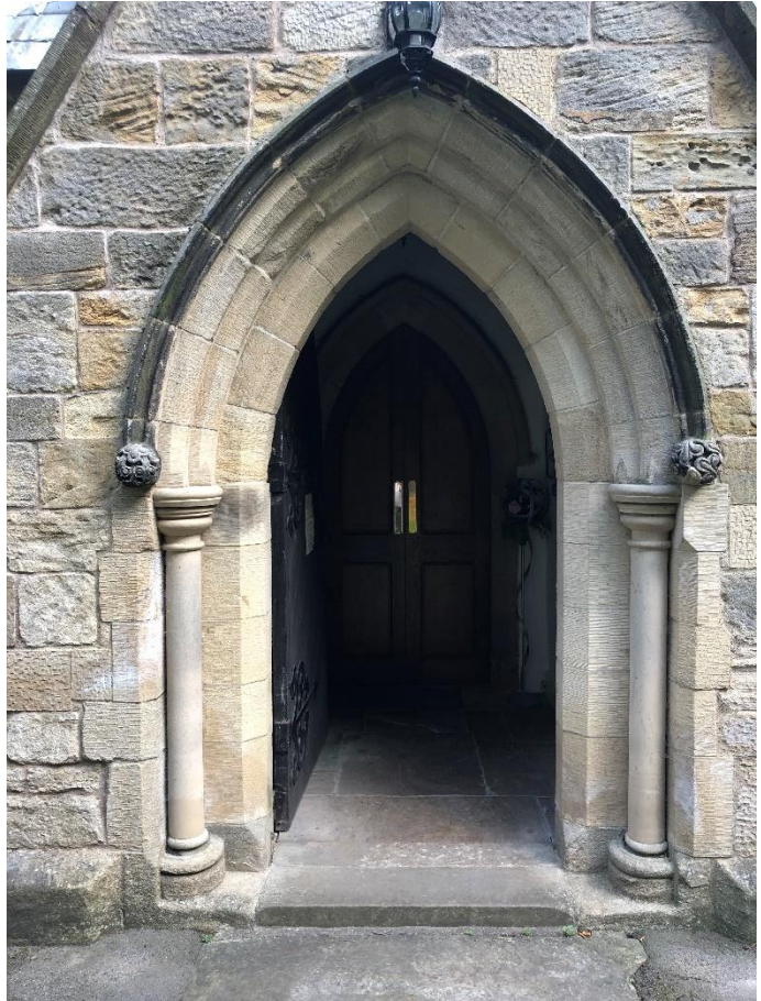
Fig. 6 (IMG 8285) Step access to porch (accessibility issues)
