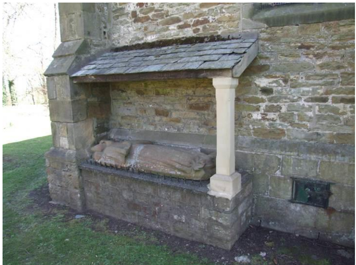
Fig. 13 (IMG 1322) Figure with roof protection and new stone column (west end of Church): some slate damage
