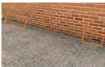
Figure 11- Floor vents to N elevation
