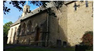
**West side** – Repoint same as the S nave, watertable has had water markings in the past running down but they are old, walling is generally sound with a bit of erosion above the plinth and this is evident right around the building. Clasp corner buttress with erosion to its lower stage.
