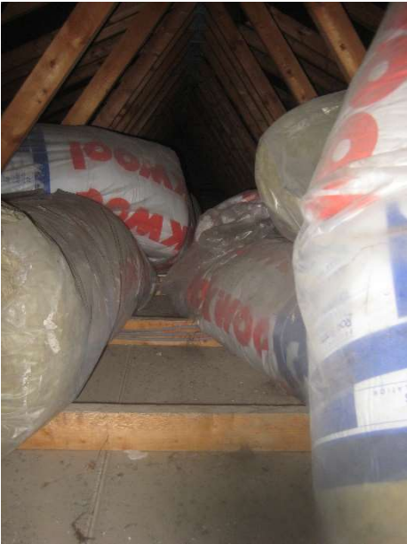
over centre of hall - mostly uninsulated despite unused rolls lying in the void
