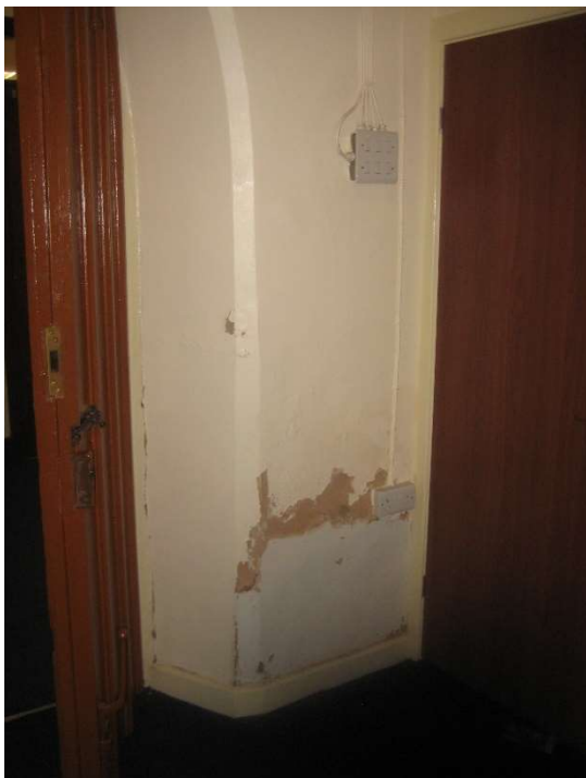
Church side of Nave doors
