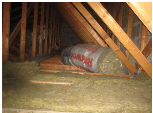
over N side of Hall – mostly uninsulated despite unused rolls lying in the void
