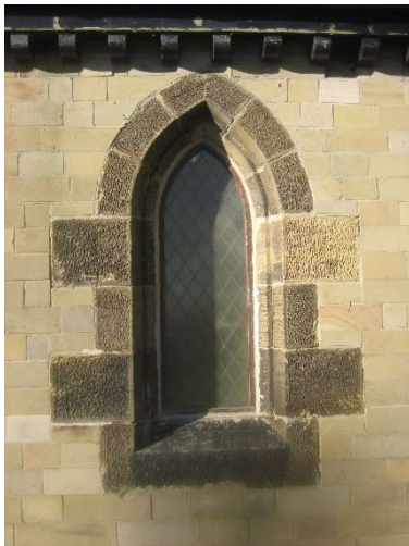
Reused window in Hall
