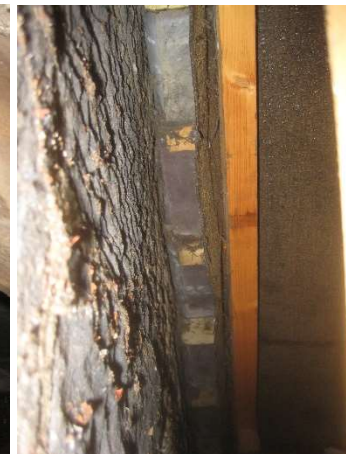
Hall felt not reaching the Nave wall
