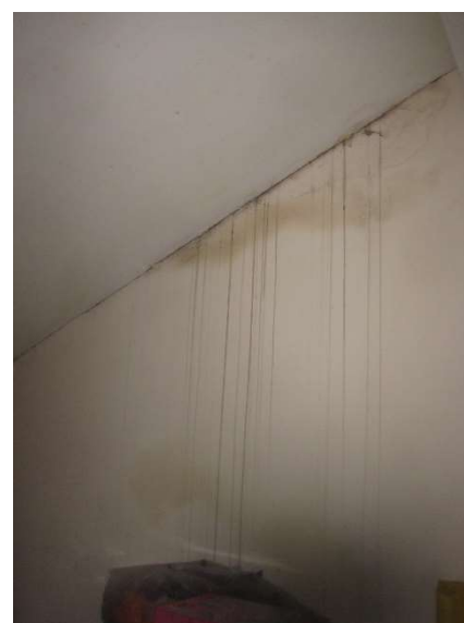
upper store wall where Hall felt does not reach the Nave wall
