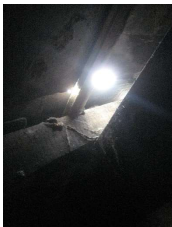
Daylight at missing slate Nave SW
