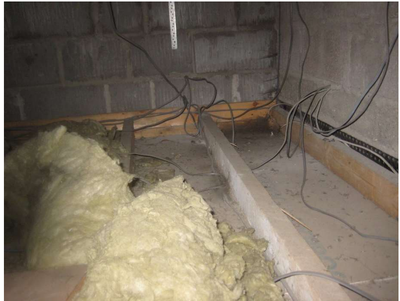
over centre of hall - mostly uninsulated despite unused rolls lying in the void
