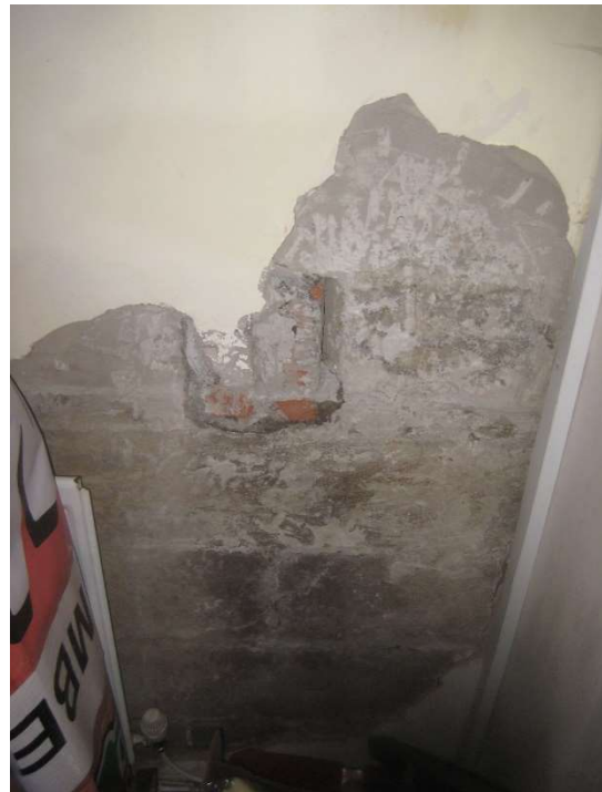
ladies wc after removal of damaged plaster
