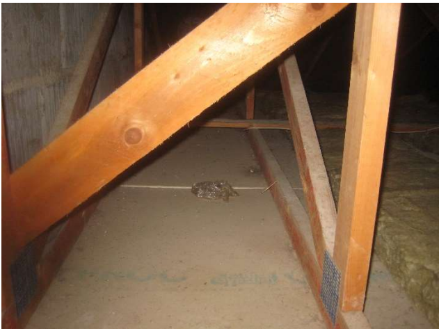
over N side of Hall – mostly uninsulated despite unused rolls lying in the void
