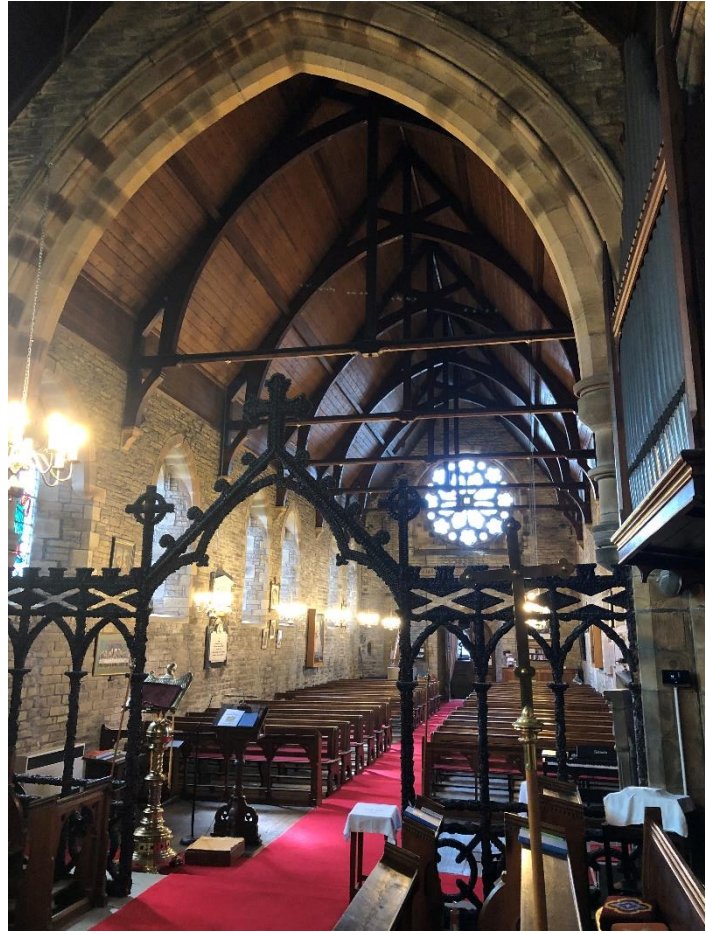
P3 (4819): Screen and roof structure, looking west
