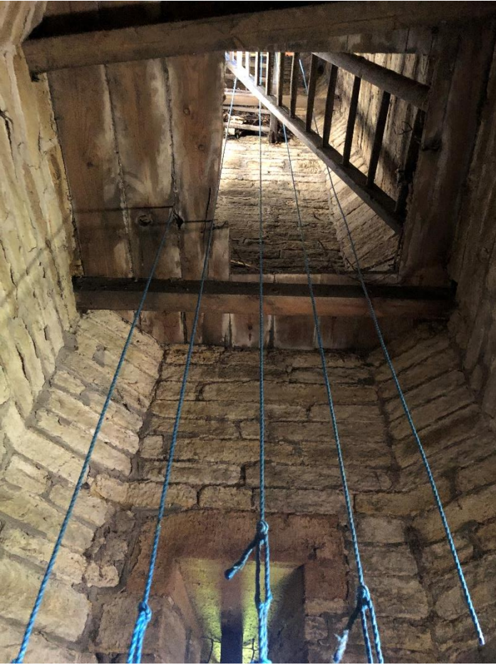
P8 (4852): Tower access
