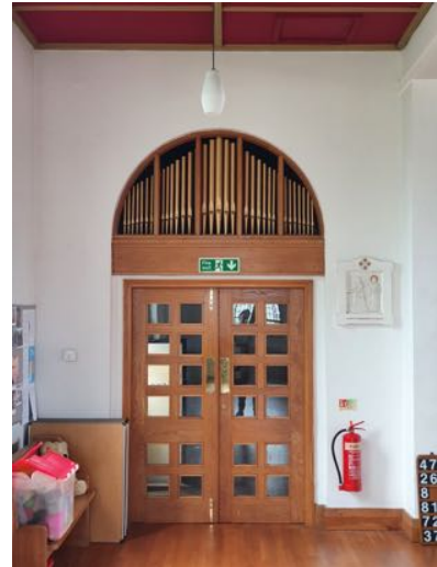
b) Doors to the lobby with decorative pipes above
