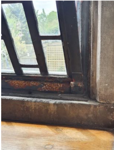
a) Ventilation hoppers have corroded
