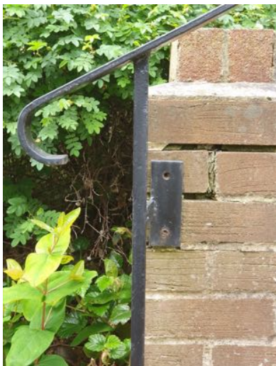
a) Repoint wall.
