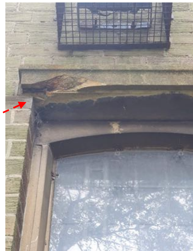
b) North Aisle window to be repaired.
