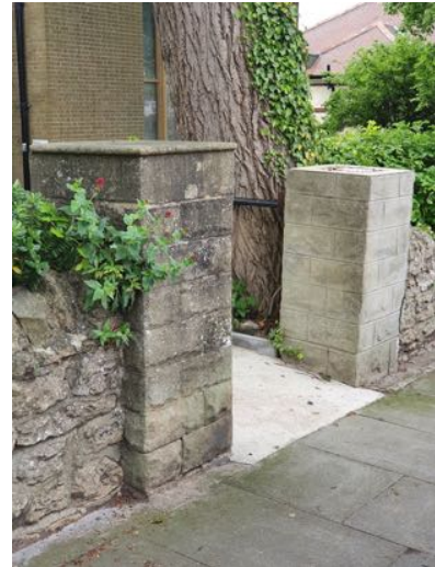
b) Pier to the south side of the pedestrian access is being pushed over by the tree.
