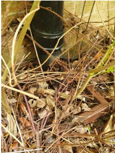
a) Downpipe is blocked with debris that has been washed down from the gutter.
