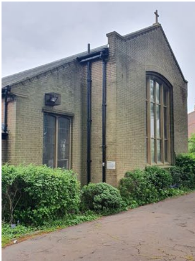
a) View from the NW
