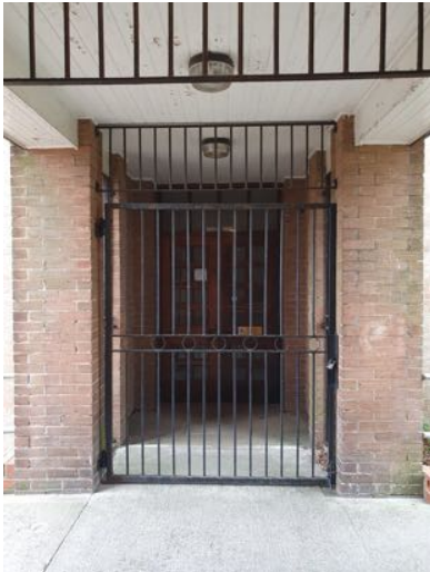
a) Secondary entrance and security gates
