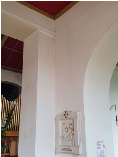
a) Settlement cracks to be monitored.
