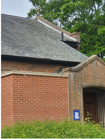
a) West end abutment flashing in good order.
