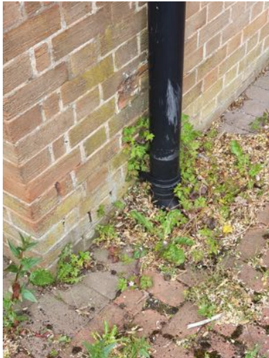
a) Gully infested with vegetation.
