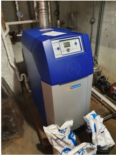
a) New boiler installed in 2020.
