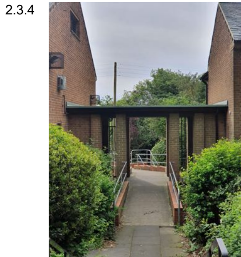
a) Covered walkway connects the Church and Hall
