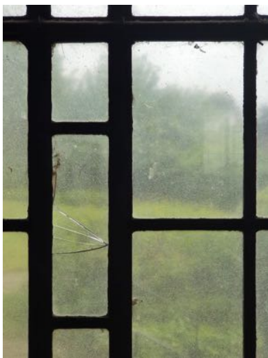
a) Minor cracks
