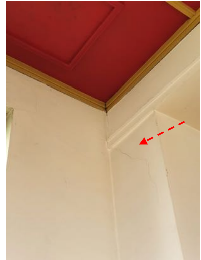
b) Settlement crack and note ceiling hatch.
