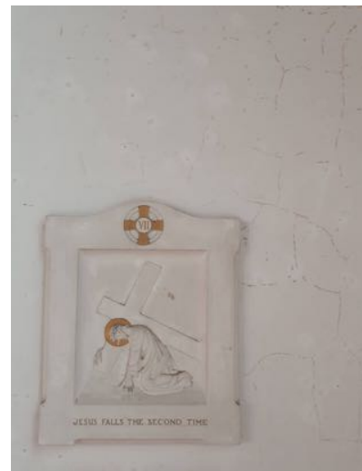
b) Wall monuments appear stable and unaffected by the cracked plaster.
