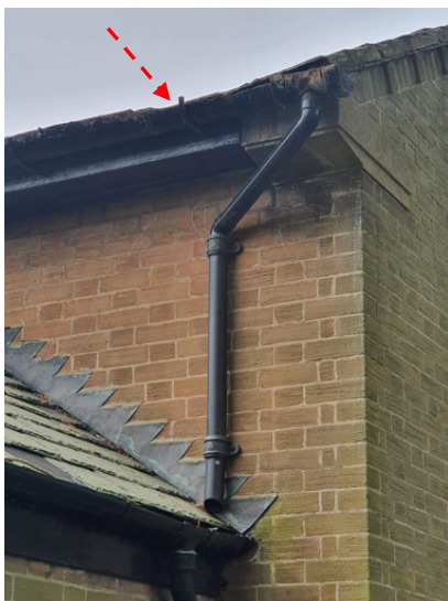
a) Cast iron gutter to be repaired
