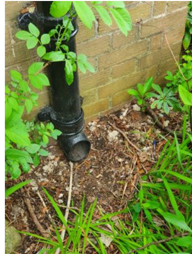
b) Gully is total concealed with debris
