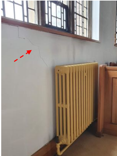
a) Cracked plaster below cill.
