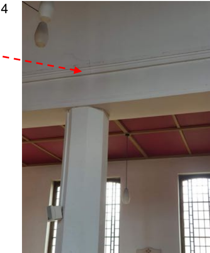
a) Probable settlement cracks to be monitored
