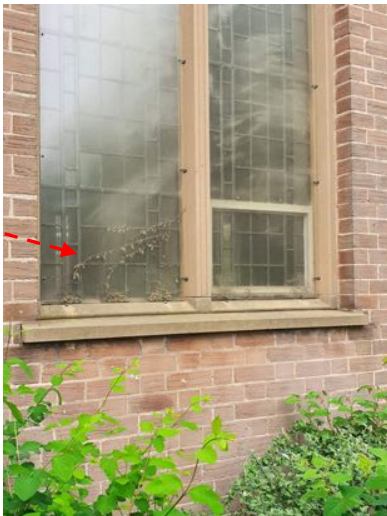
a) Debris trapped behind Perspex security sheet to be removed
