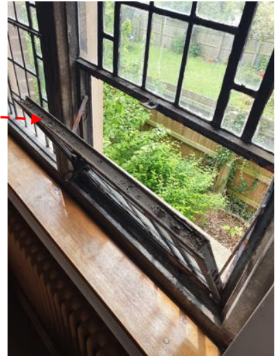
b) Previous decorative coating is breaking down.
