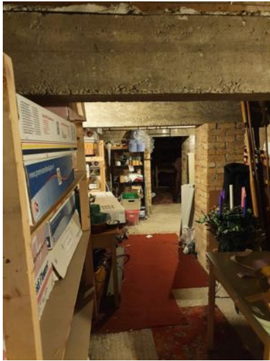
a) Undercroft is used for casual storage.
