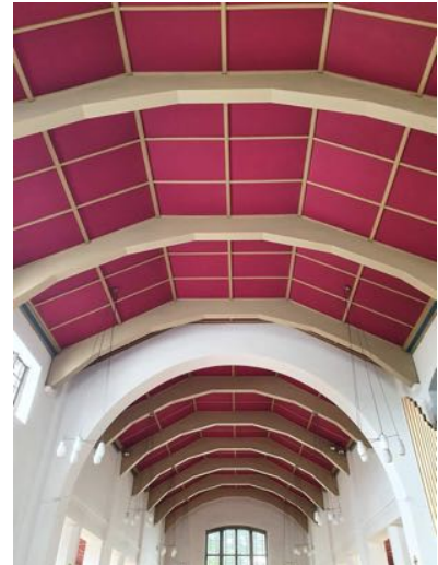
b) Continuous ceiling detail over the Chancel and Nave.
