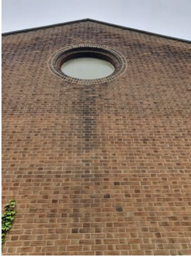
a) Staining below circular window
