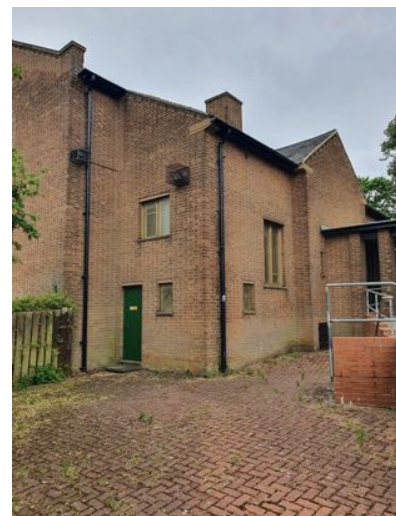
b) The building is 2 storeys in height at the east end due to the slope of the site.
