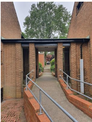
a) Covered walkway viewed from the east.
