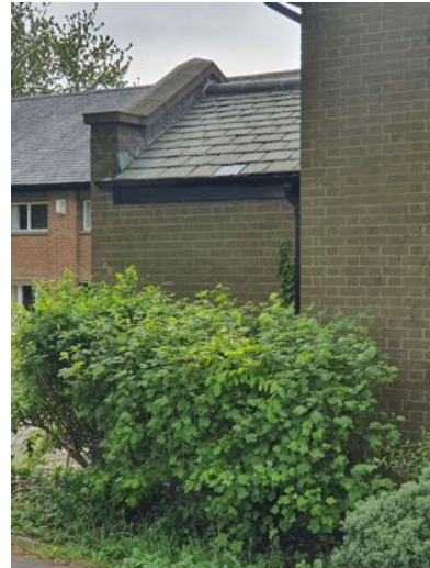
b) Lead flashing to brick parapet
