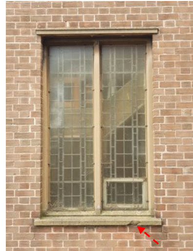
b) Damaged cill to stairwell window.
