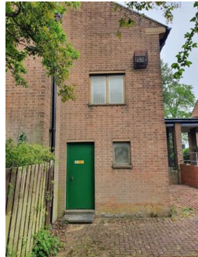
b) East return end with escape door and windows to the WC and Vestry.
