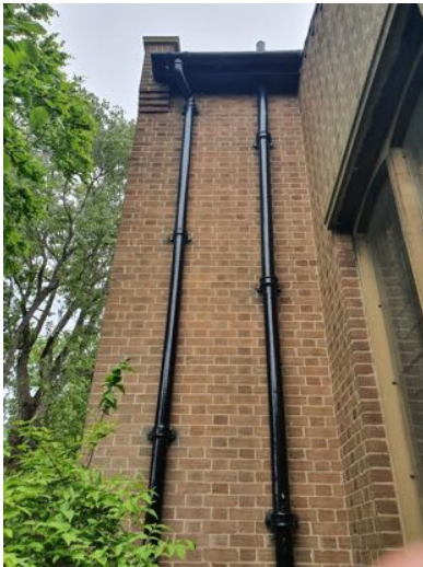
a) Fall pipe and from the Lady Chapel roof to the south. Right of that is a soil and vent pipe.
