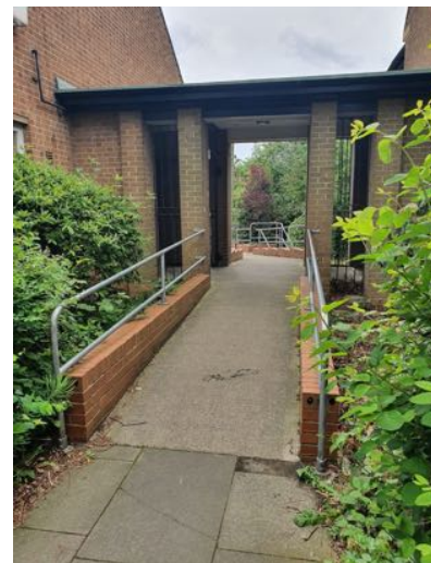
b) Ramp access to covered walkway
