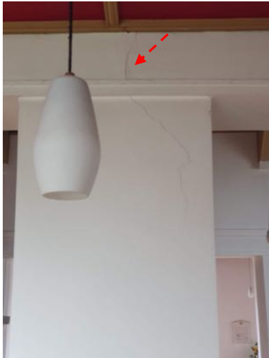
a) Cracked plaster finishes – to be monitored.
