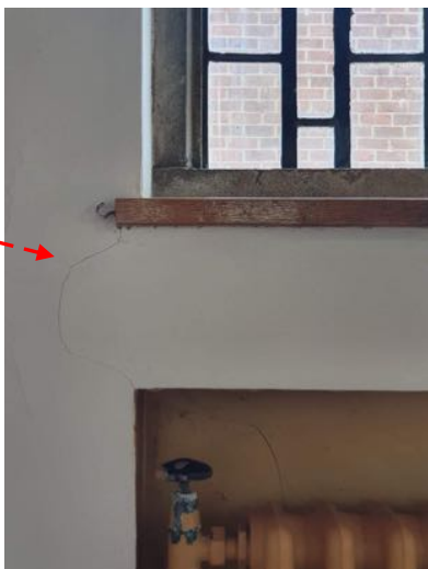
a) Minor plaster cracks
