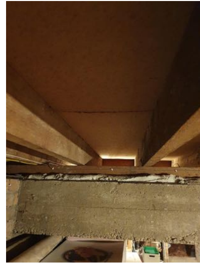
b) Exposed floor structure.
