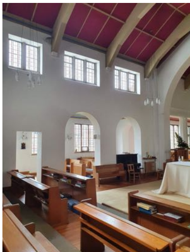
a) Clerestory windows to the south side of the Chancel
