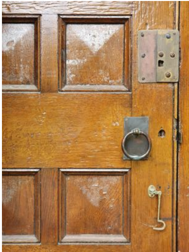
a) Lacquered finish starting to flake
