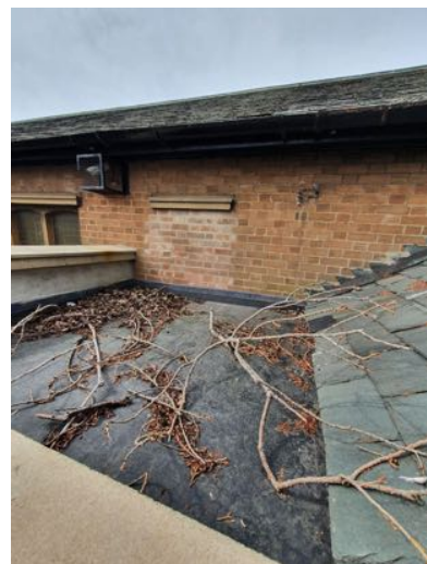
b) Ensure debris is cleared regularly from the flat roof.
