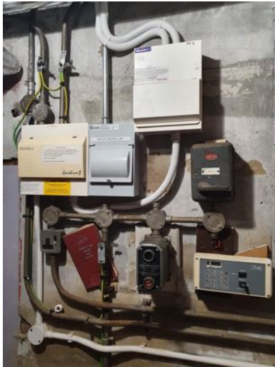
a) Electrical distribution boards
