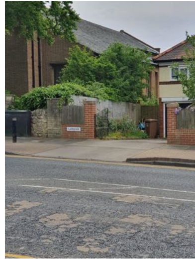
b) South slope viewed from Durham Road.
