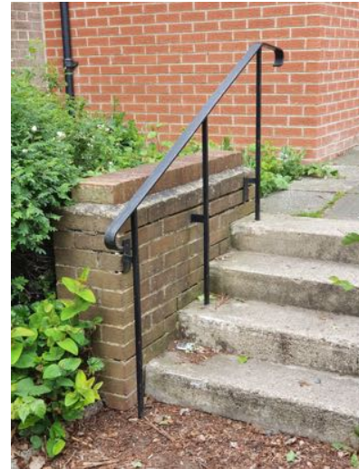
b) Resecure handrail
