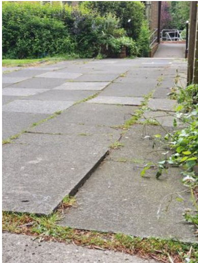
a) Uneven flagstones could present a trip hazard.
