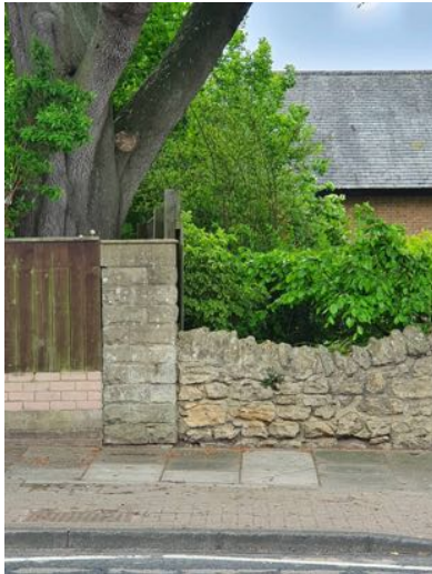
a) Boundary wall.
