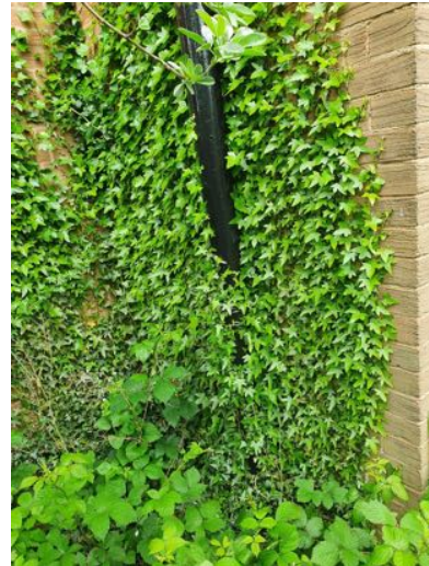
b) The base of the downpipe and gully are total inaccessible due to vegetation.
