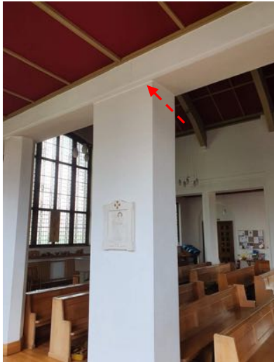
a) Settlement crack
