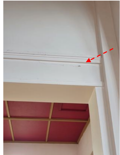
b) Probable settlement cracks to be monitored
