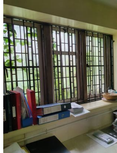
b) Vegetation can be seen growing over the east window fitted with internal security bars.
