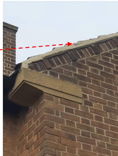
b) Minor cracking to verge pointing.
