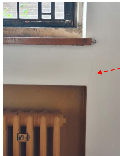
b) Minor plaster cracks
