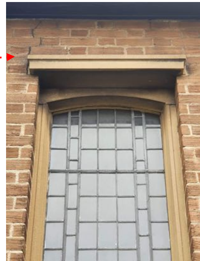
b) Minor settlement crack is reflected in the internal plaster finishes
