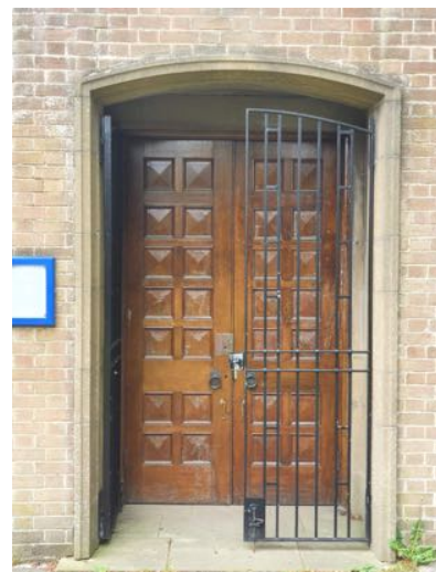
b) Entrance doors recessed with metal security gates set in front.
