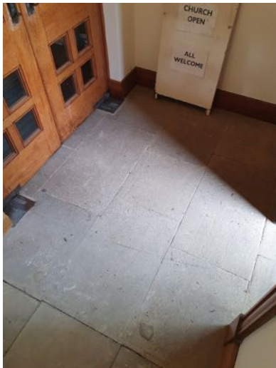
a) Stone paving provides a suitably durable surface
