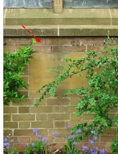
b) Open joint above foundation stone
