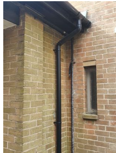
b) Plastic guttering and downpipes
