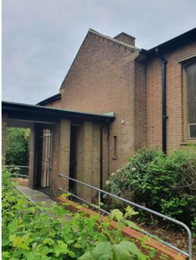
a) Covered walkway and gable end to the Organ Loft above
