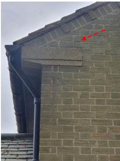
a) Minor crack above kneeler
