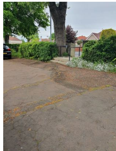
b) Tarmac drive undulates due to tree roots
