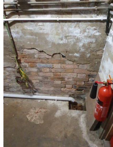
b) Missing render from the lower section of wall and drainage outlet.
