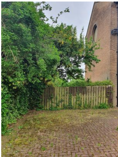
a) Gateway in fencing to be refurbished and made operational
