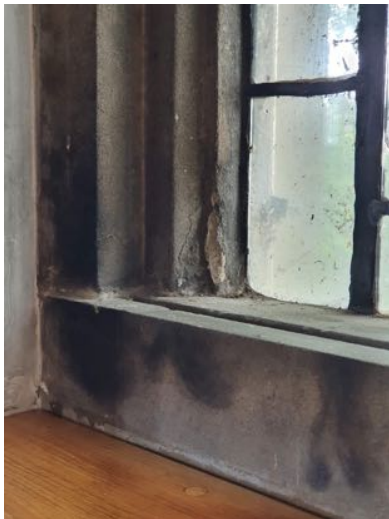
a) Minor decay to the stone window surrounds
