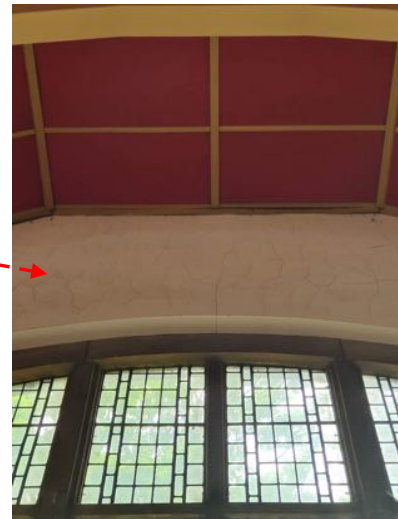
b) Crazed cracked plaster above west window
