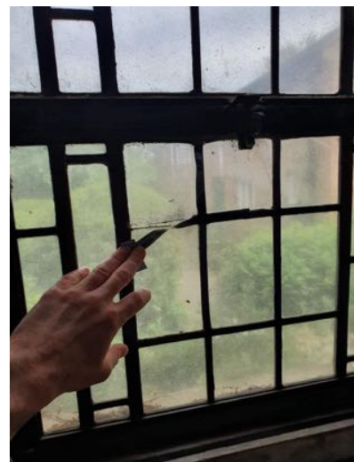
b) Missing section of lead came to be replaced.
