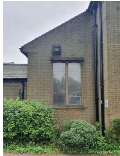
b) West elevation of North Aisle
