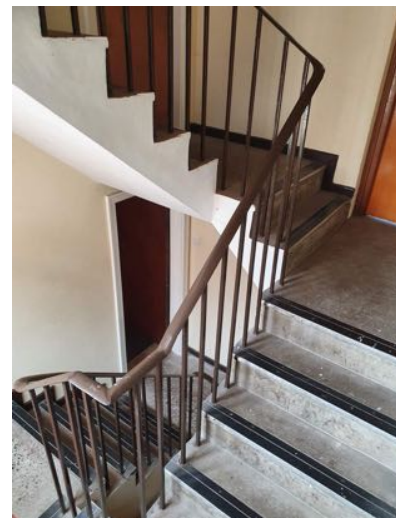
b) Concrete stair and landings.
