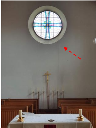
a) Runnel marks at the cill of the circular window.
