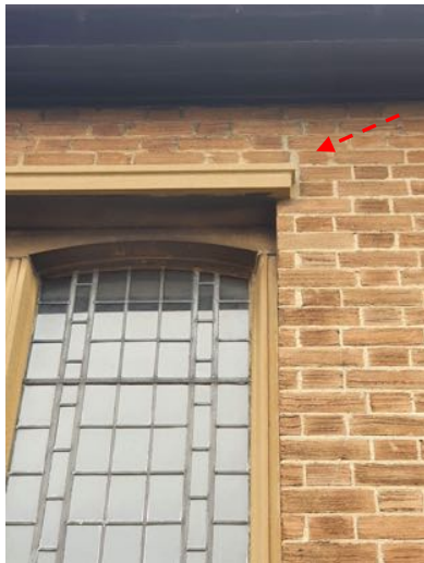
a) Settlement crack previously repointed.
