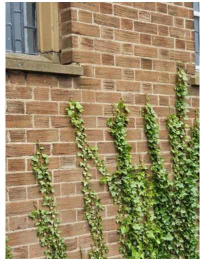
b) Ivy needs to be removed from the base of the walls.
