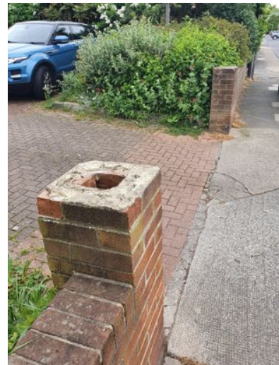
b) Caps missing from gate posts
