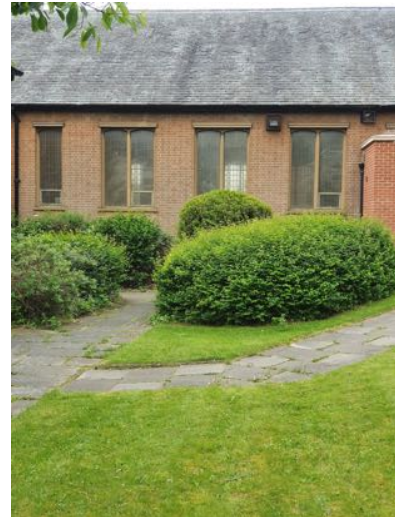
b) North Aisle windows.
