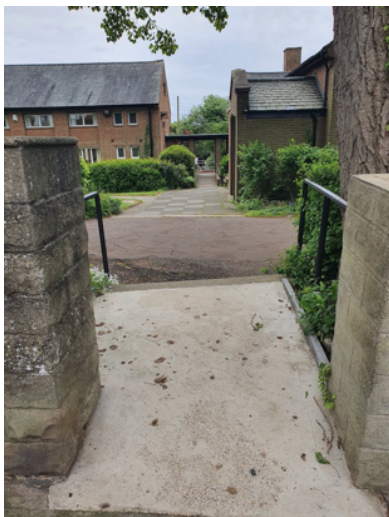
a) Concrete shuttering to replace displaced flagstones
