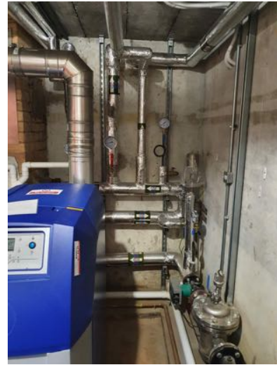
b) Well insulated pipework
