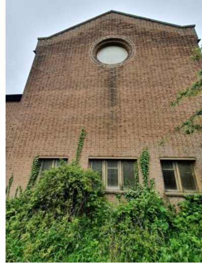
b) Overgrown vegetation obscures the base of the wall and is encroaching on the lower windows.
