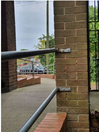
a) Galvanised tubular handrails showing some signs of corrosion.
