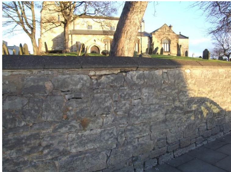
Fig 29. Tree growth, potentially compromising wall condition
