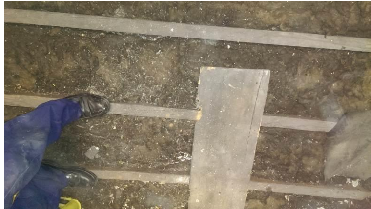
Fig 12. Evidence of woodworm, north aisle loft
