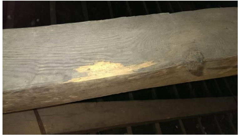
Fig 11. Evidence of woodworm, north aisle loft
