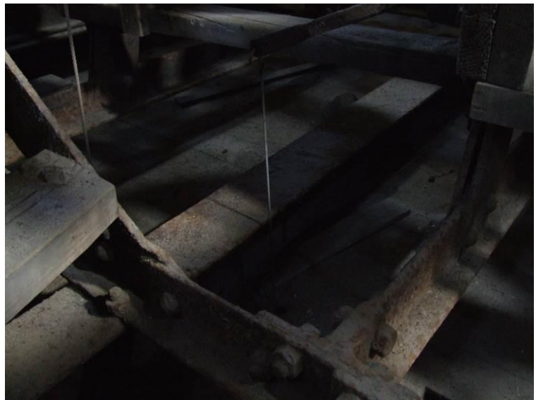
Fig 4. Corrosion to bell frame
