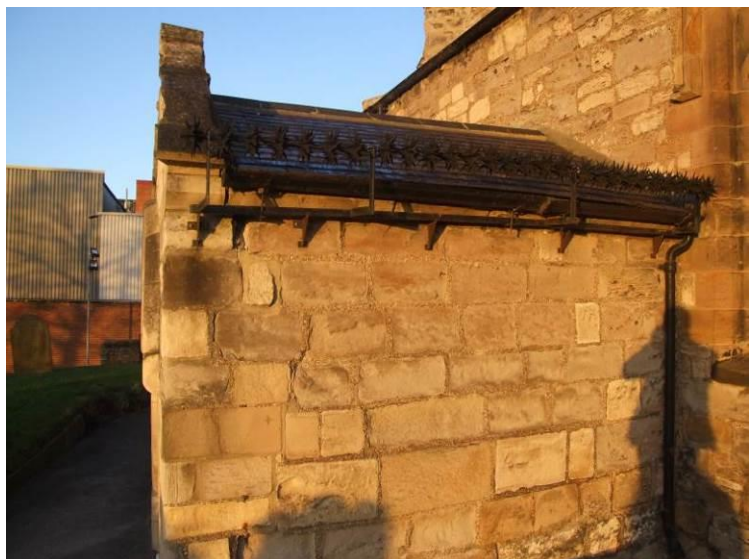
Fig 20. Localised cracking to Porch east gable
