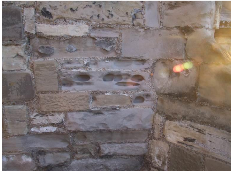
Fig 18. Localised area of extreme erosion to Tower
