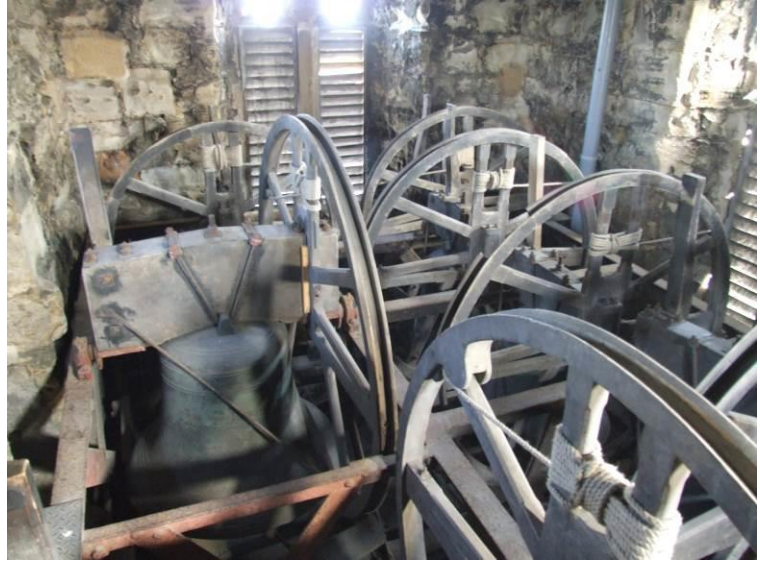
Fig 3. Corrosion to bell frame
