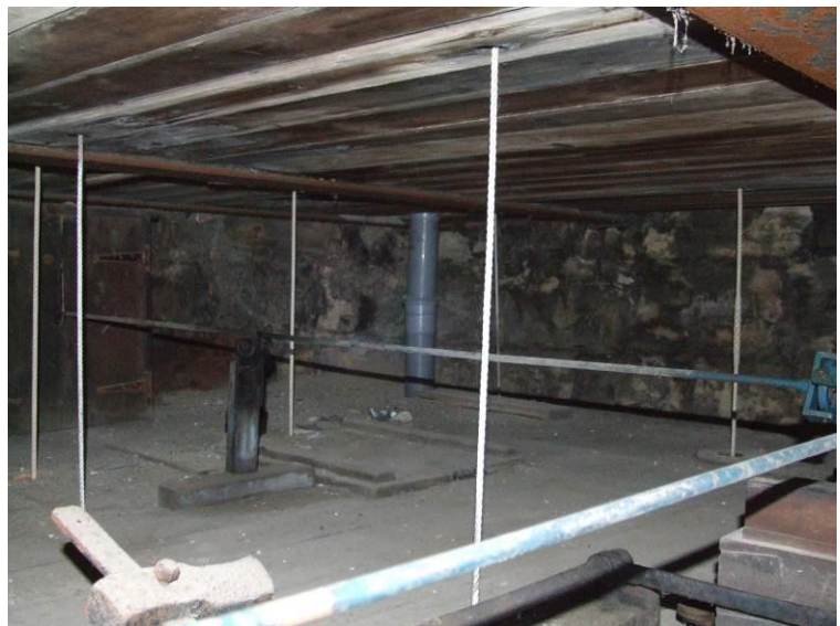
Fig 5. Steelwork, Belfry floor void
