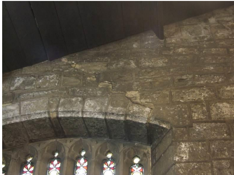
Fig 8. East gable wall above window, Fulthorpe Chapel
