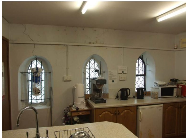
Fig 9. East gable wall above northernmost window, Kitchen area
