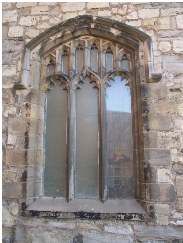
Fig 17. Stained glass protection, some tightly pointed in, latter with recommended air gap to perimeter
