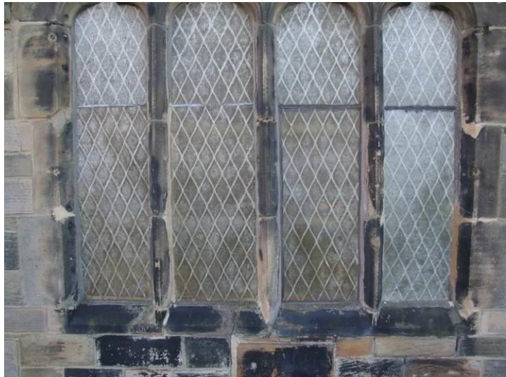
Fig 25. Window detail showing glazing and repointing, Choir Vestry
