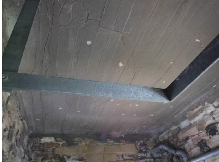
Fig 6. Tower roof structure
