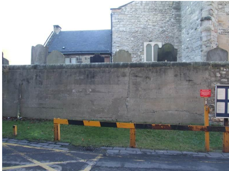
Fig 28. Mass concrete retaining wall to Brewery access road
