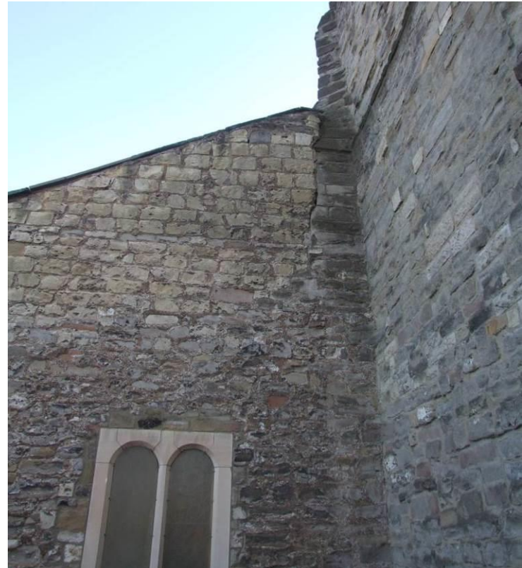
Fig 27. Detail of Choir/north aisle junction; likely area of water ingress
