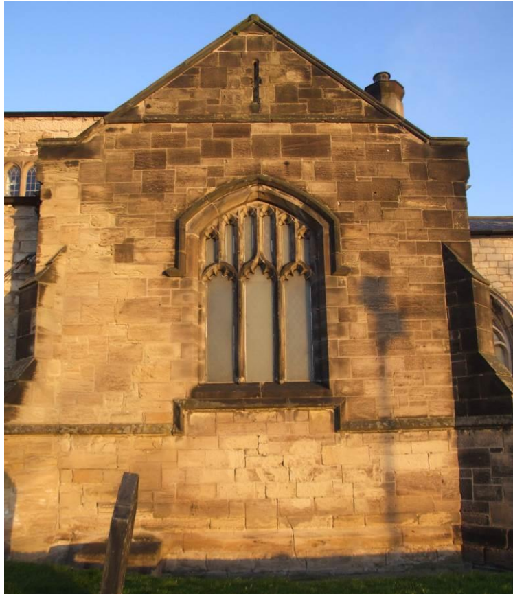
Fig 21. Central vertical cracking below Organ Chamber, south window
