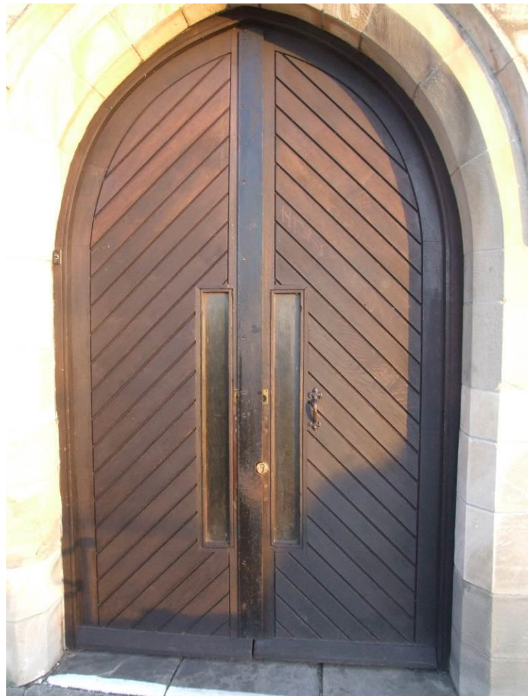
Fig 15. Main entrance door, suggested re-glazing of view panels; redecoration of metalwork/timber
