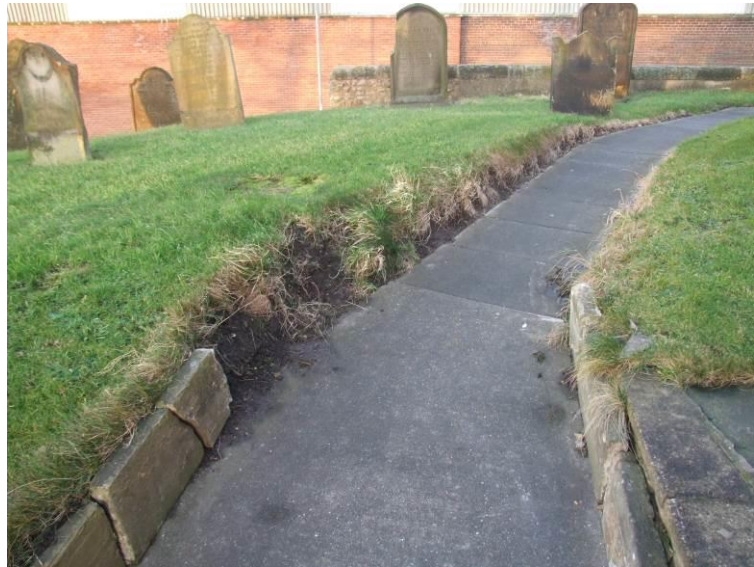
Fig 16. Missing kerb access to pathway
