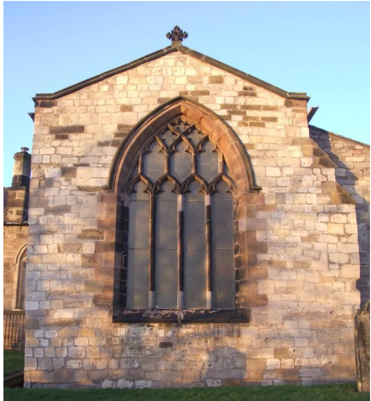
Fig 23. Central vertical cracking below east chancel window
