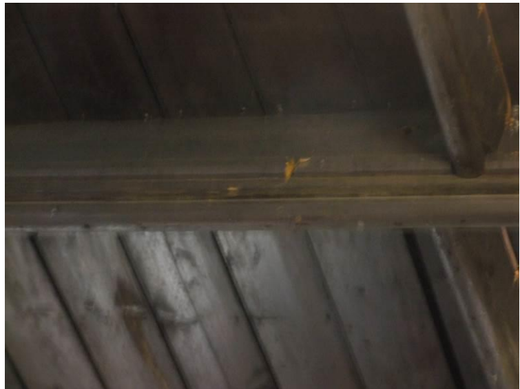
Fig 1. Evidence of woodworm, Fulthorpe Chapel ceiling
