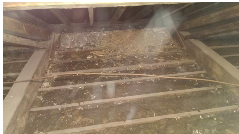
Fig 10. Evidence of woodworm, north aisle loft
