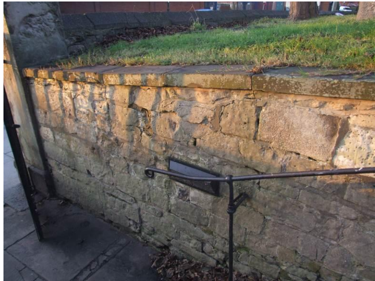
Fig 14. Small area of open joints to retaining wall
