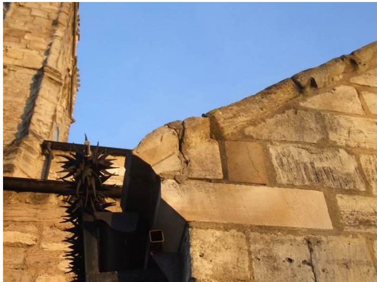
Fig 19. Repair required to termination of water tabling
