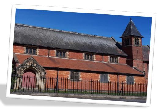
In need of some repairs, some remedial has already been undertaken to repair the Spire, (following storm damage) and to lower the roof; a small grant towards the roof repair cost was awarded by the National Churches Trust and the Durham Diocese Church Building Fund. Internally there has been some plasterwork repairs due to damage by water leaking in from the roof.
