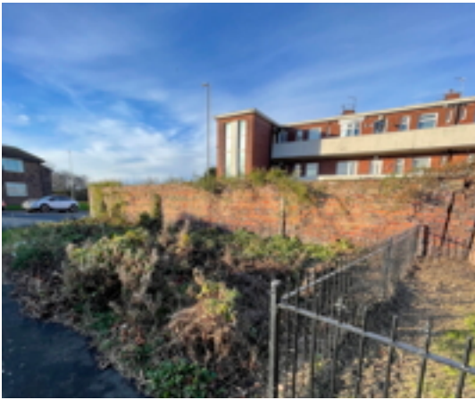
North West Corner
