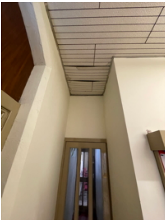
Kitchen Lobby Looking East
