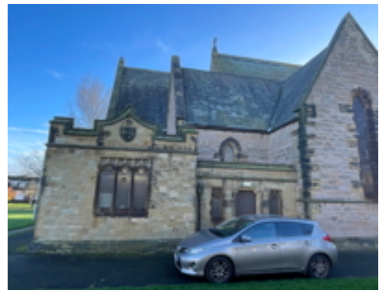
North East Corner Roofs
