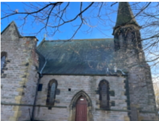
North Elevation Roof
