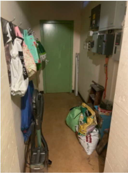
Tower Passageway Looking East
