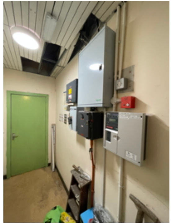
Tower Passageway Looking East
