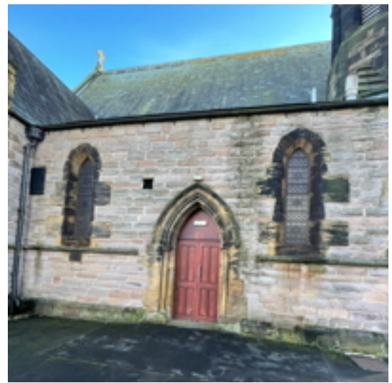
North Aisle Windows and Door
