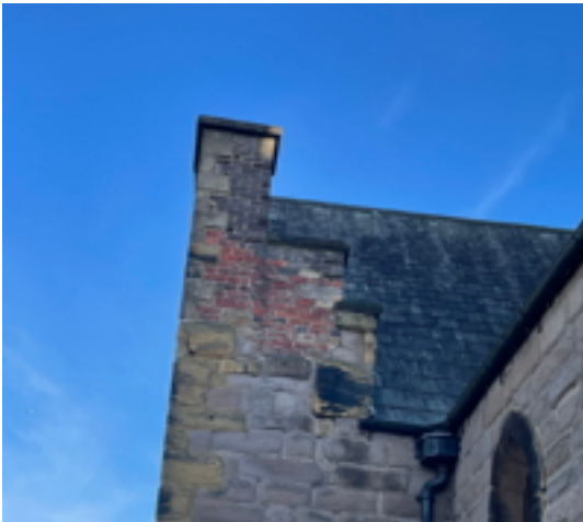
Vestry Chimney West Elevation
