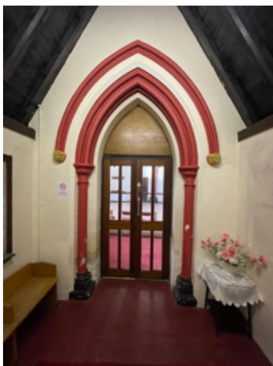
South Porch Looking North
