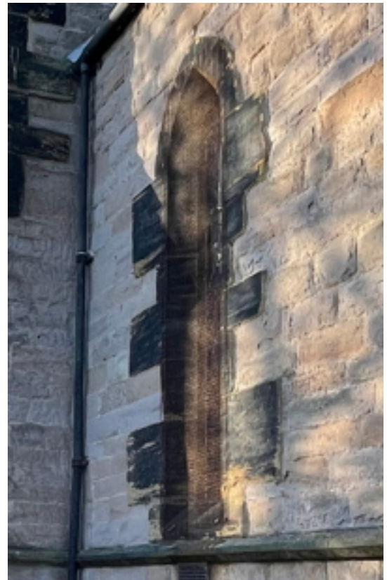
Typical Mesh Protection
