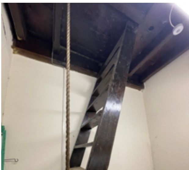
Ladder and Hatch Over
