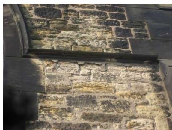
stone decay next to over-hard pointing under the window and under the string course near the N buttress
