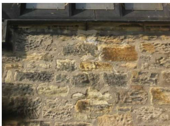
stone decay next to over-hard pointing under the window and under the string course near the N buttress
