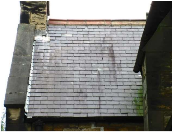
W side of Organ Chamber – lead flashings at gable pulled apart
