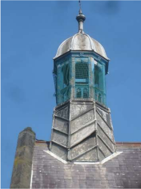
2015 lead panel coming loose 2020 lead panel missing from S side of turret and slate slipped from Nave eave
