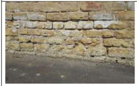
Modern cement mortar is cracking and coming away.
