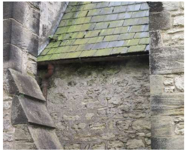
between Chancel and Choir Vestry Chimney
