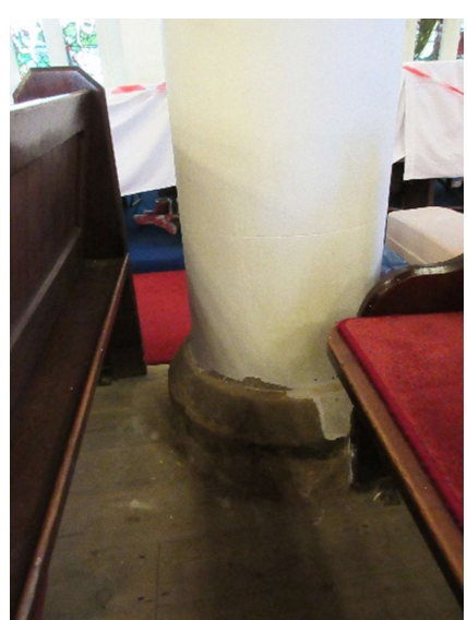
SW pier nave side 2017
