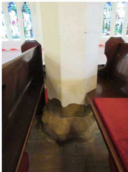
S mid pier nave side 2017
