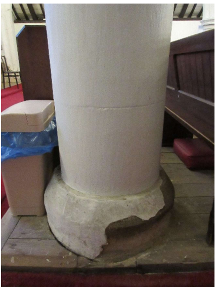
SW pier aisle side 2017
