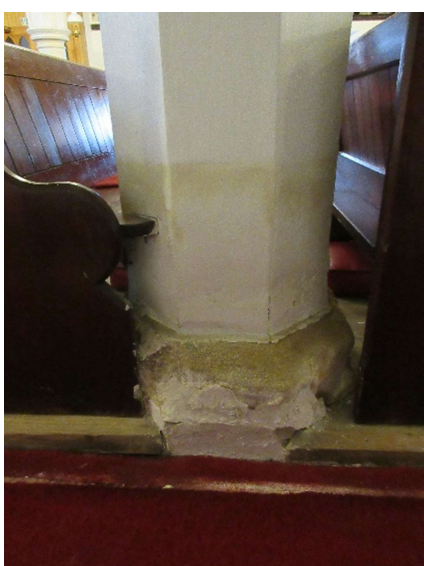
S mid pier aisle side 2017
