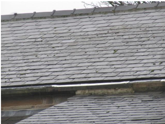
Mortar fillet over the organ Chamber roof
