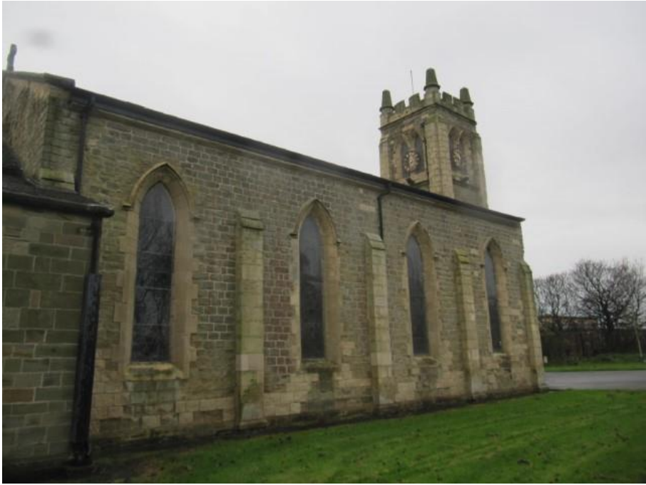
General View of the North Elevation (Nave) from the East
