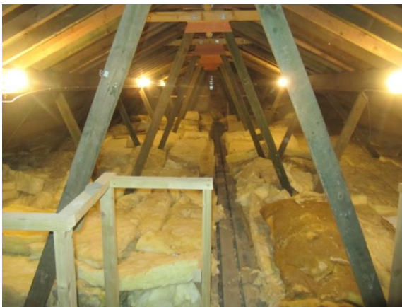
Good levels of insulation above the Nave
