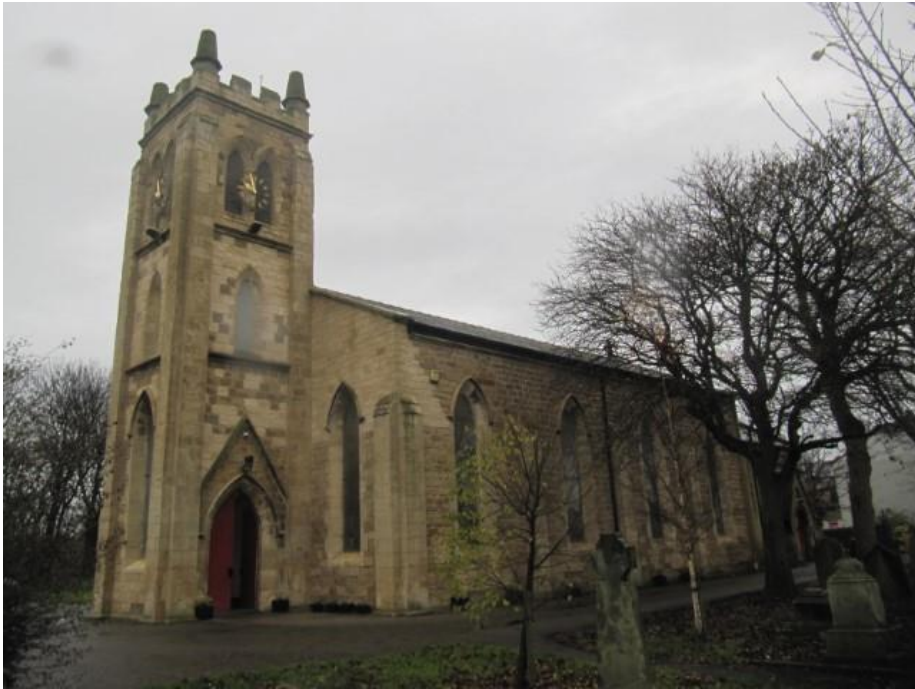
General View of the South Elevation from the West
