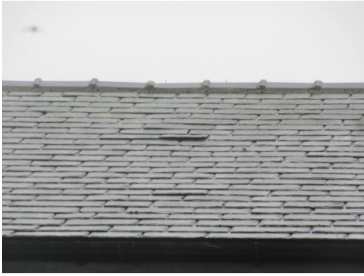
Lifting slates to the North Nave roof
