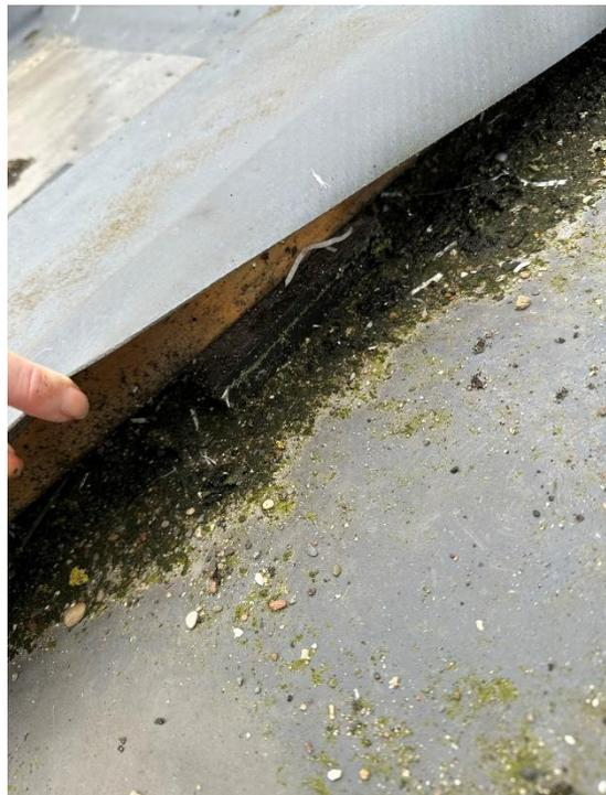
*Figure 11- underside of single ply over beam*
