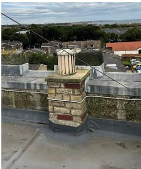
Figure 36 – Boiler flue terminal
