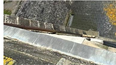
*Figure 6 – Tower downpipe*
