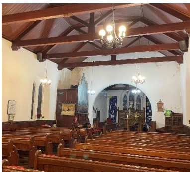
Internal View of Nave
