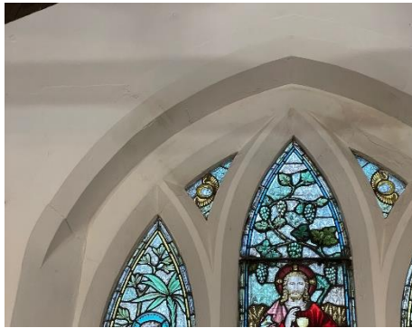
15.2.3 Cracking and discolouration to lancet
