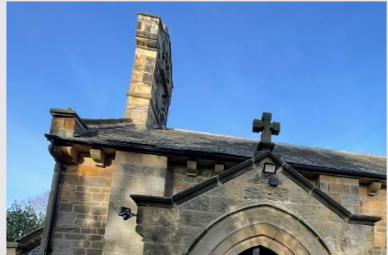
Item 7.1- Slates near south west bellcote
