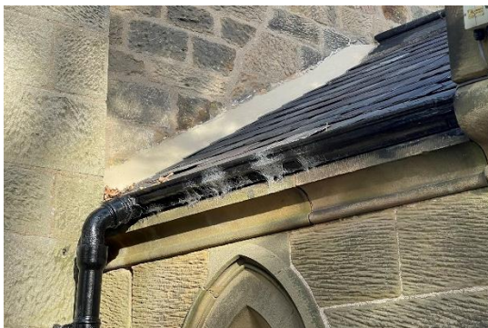
Item 7.3- New flashing to S porch / Nave abutment
