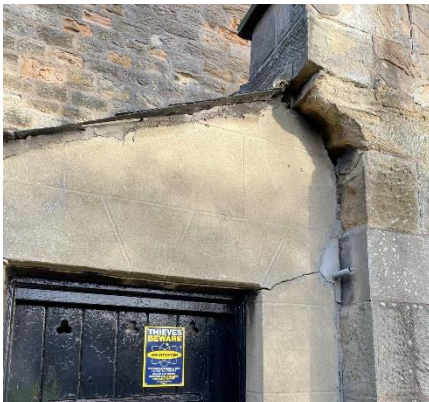
9.9 Boiler room abutment to West Porch
