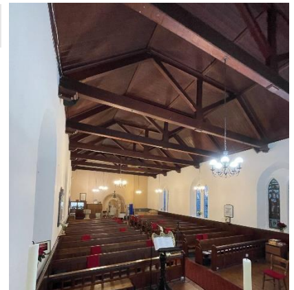
13.1 – internal view of Nave
