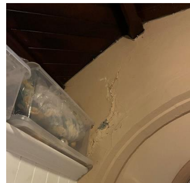
15.3.3 – crack and blistering
