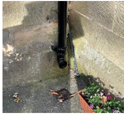
Item 8.3 – RWP outlet
