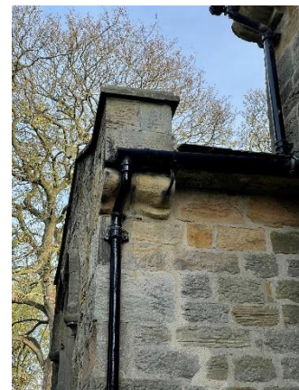
8.8 & 8.9 N Nave/ Vestry RWP
