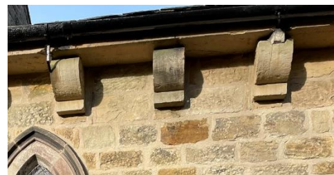
Item 8.5 – Gutter brackets
