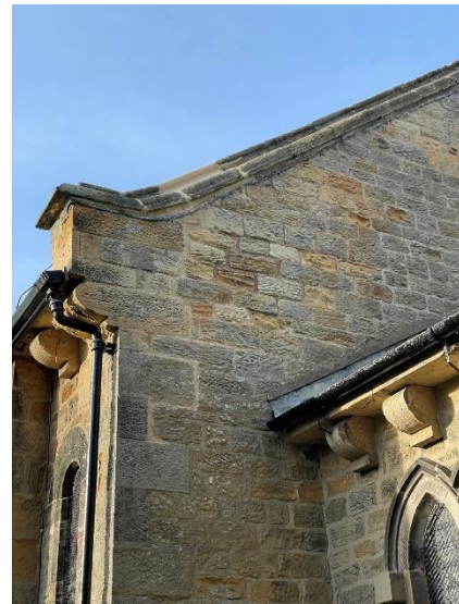
9.5.1 – Repair to S Nave
