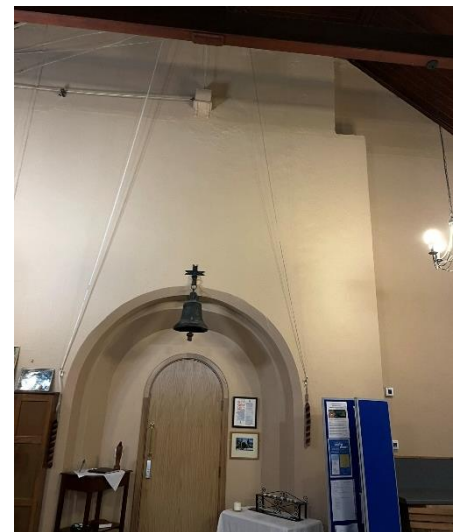
15.1.1 West end of Nave – all cracking filled
