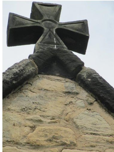
Open joints to apex on porch and gnomon weathered stonework to gable
