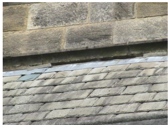
Failed mortar to South Aisle roof
