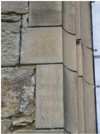
Open joints to jamb of window n(iv)
