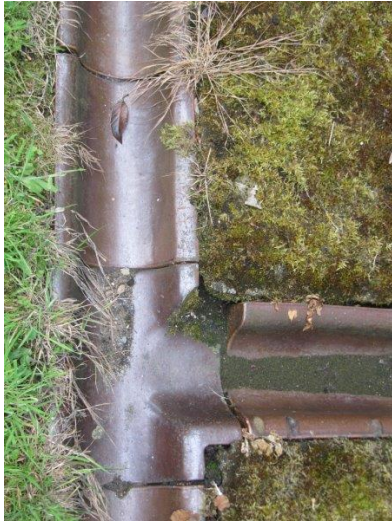
Open joints to drainage channel to North of the church and vegetation
