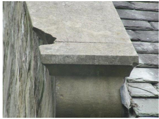
Damaged section of water table to organ chamber
