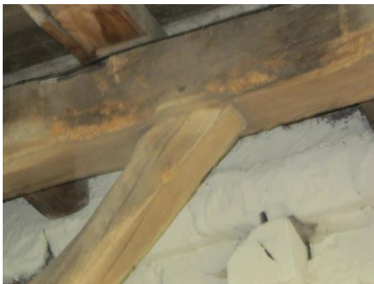
Lighter patches to timbers in Tower ringers chamber coming loose
