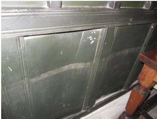
Bowed paneling to South Aisle
