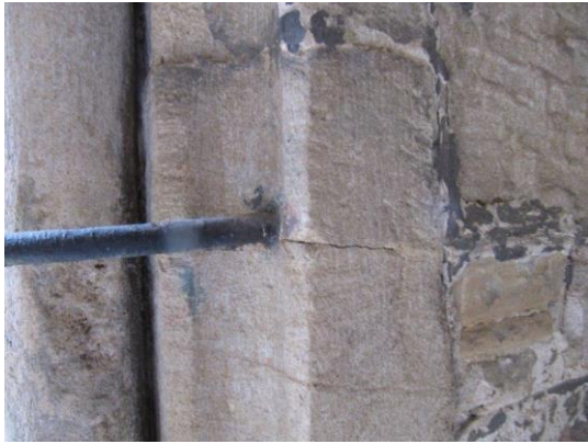
Metalwork to porch jamb with cracked stone
