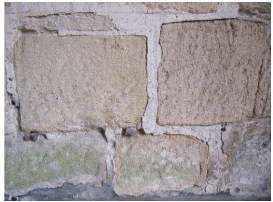
Open joints/failing mortar to porch
