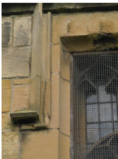
Weathered stonework to South Aisle
