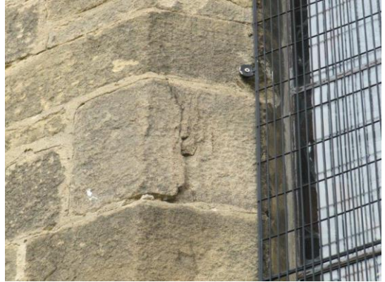
Cracked stone to jamb of S(vi)
