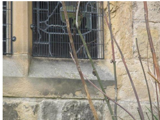
Weathered stonework to window S(viii)
