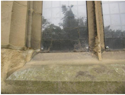
Weathered stonework to Vestry window
