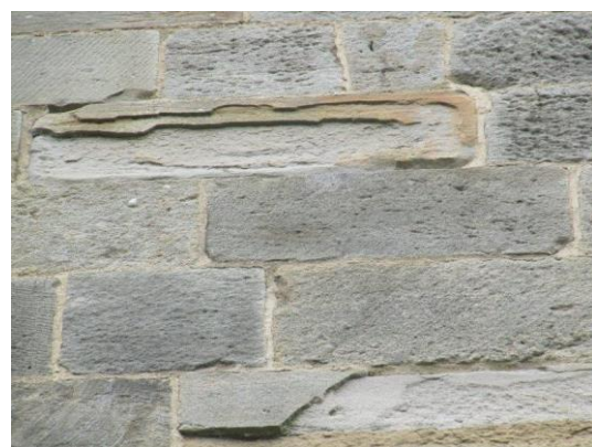
Delaminating stonework to East elevation of Chancel
