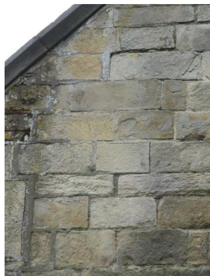
Cracking and failing mortar to North of Elevation of organ chamber
