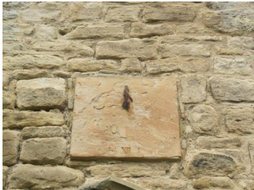
Weathered stone to sundial and bent on porch
