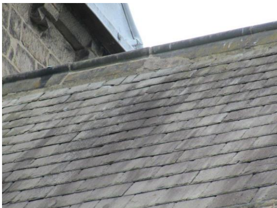
Slate starting to slip on Nave roof and repaired ridge tile
