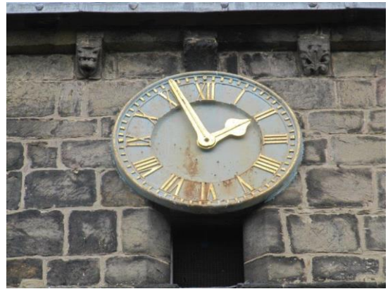
Rusting face to tower clock
