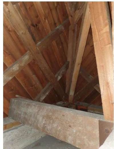
b) Diagonal boarding overlaid and cross braced.
