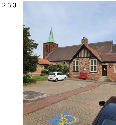
a) Main roof over the Nave abuts the Tower. The library is in the foreground with chimney at the gable end.
