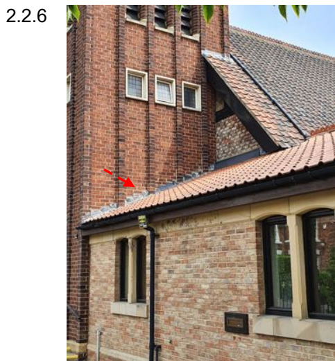
a) Abutments flashings weathered with some replacements.
