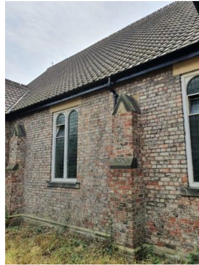
b) Nave north slope. Gutters, fascias soffits etc well decorated.
