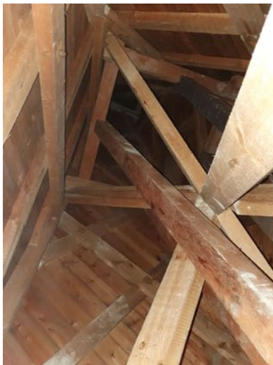
a) Loose rafters create the elongated pyramidal spire
