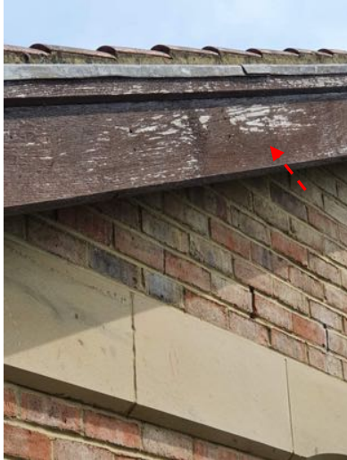
a) Bargeboard to the south gable is ready for redecoration.
