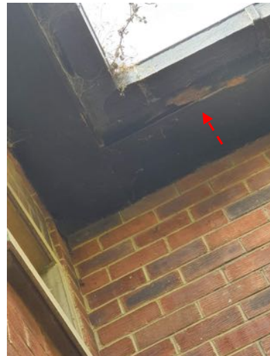
b) Minor damage to the fascia board. Probably due to the blocked gutter above. Localised redecoration required.
