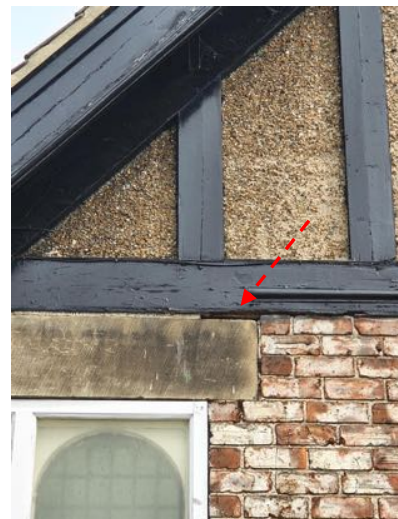
b) Mortar loss between masonry and timber beam.
