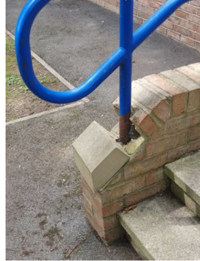
b) Loose masonry block was removed by the Architect as a precaution to avoid the risk of injury.
