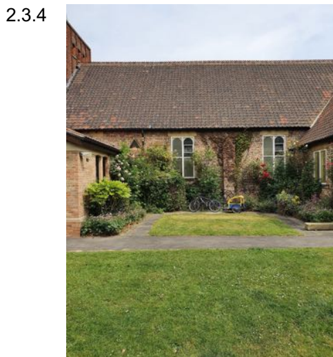
a) South facing Nave roof.
