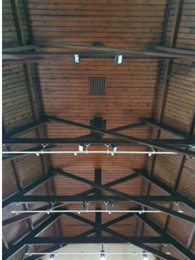
a) Exposed roof structure with ventilation and access panels in flat ceiling.
