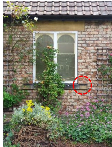
b) Cracks to cill in the west elevation
