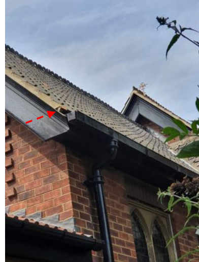
b) Small section of pointing missing from the east verge on the north side of the Chancel.
