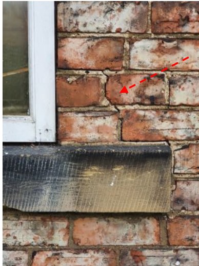
a) West elevation – crack above the cill
