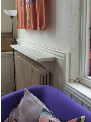
a) Cracked plaster reveals
