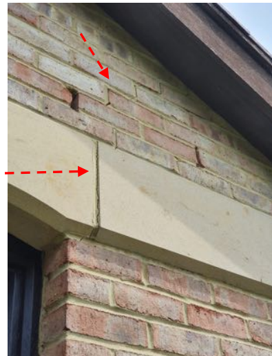
b) Stepped crack to be repointed.
