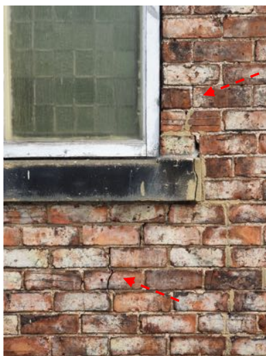
a) South elevation – cracking around the cill
