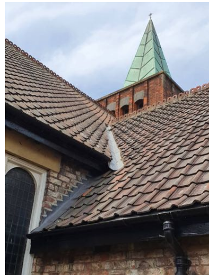
b) East face of the Tower.
