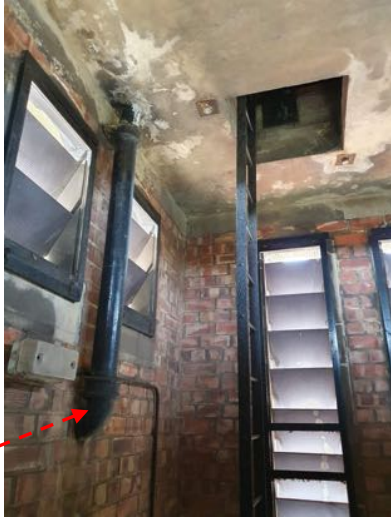
a) Cast iron downpipe drains the tower roof.
