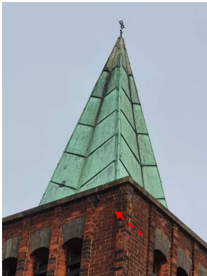
a) Overflow in the southeast corner.
