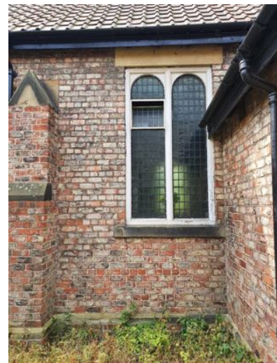
b) Buttresses between Nave windows
