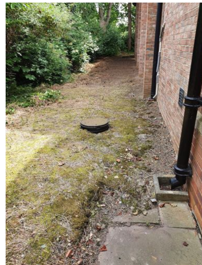
b) Manhole cover set quite high above ground level and vulnerable to damage if machinery is brought into the area.
