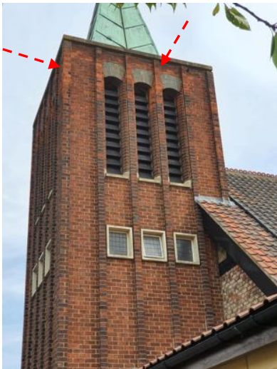
a) South elevation. Note the concentration of orange coloured bricks where surface erosion is taking place.
