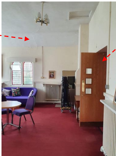
a) Entrance from the Nave on the right of picture. Plaster cracks in the west wall and ceiling are visible.
