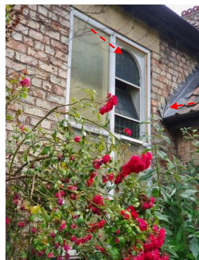
b) Panel removed to allow ventilation. Abutment flashing is working loose.
