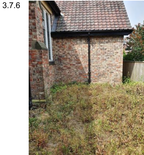
a) East elevation was underpinned
