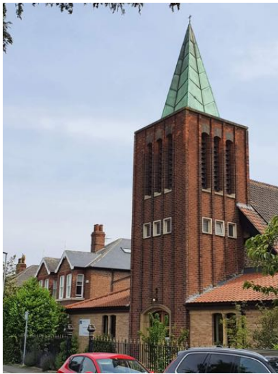
a) View from the southwest.
