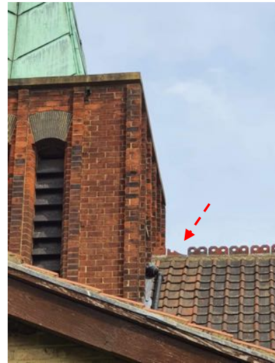
b) Broken ridge tile to Nave roof.
