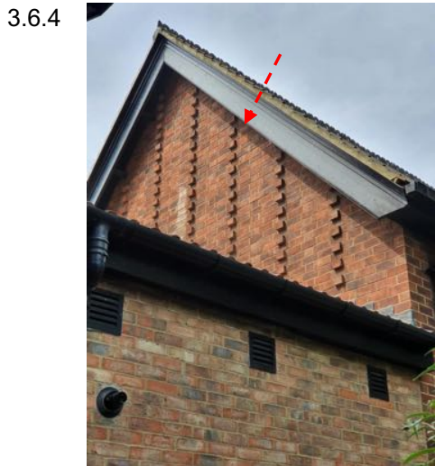
a) Projecting header brick in a Flemish bond
