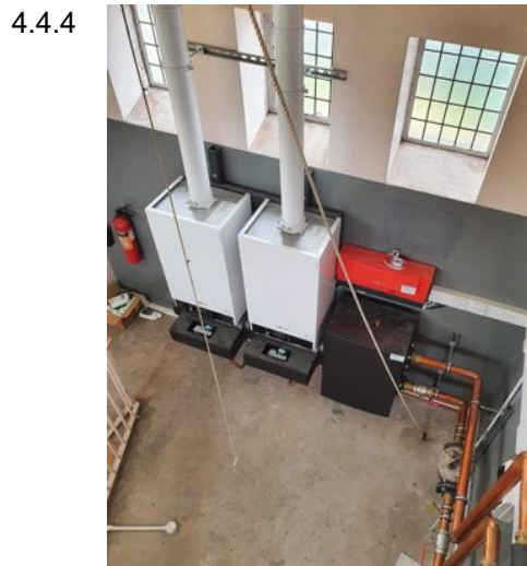
a) Boiler fixed to the north wall
