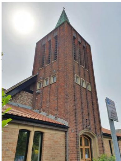
a) Boiler vents can be seen above the windows in the north elevation.
