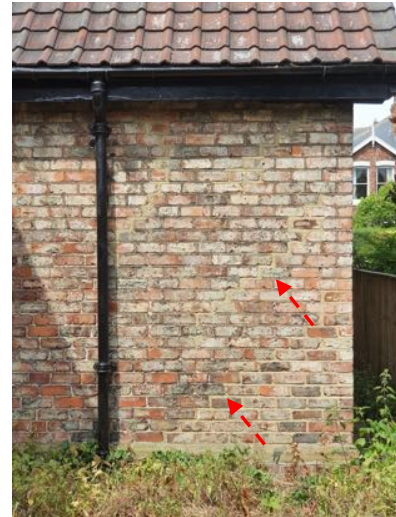
b) Stepped crack has been repointed
