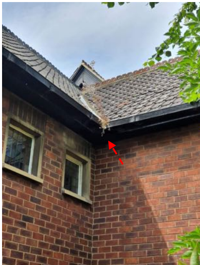
a) Remove blockage in the gutter at the valley between the Chancel and Organ Loft roofs.
