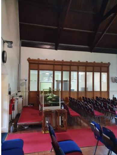
a) Timber screen infills opening in the north wall to enclose the Office.
