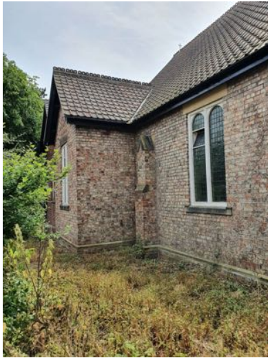
a) Former Organ Loft(?) intersects the north slope of the Nave.
