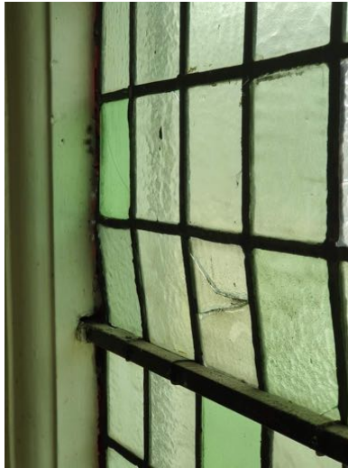
a) Buckled glazing
