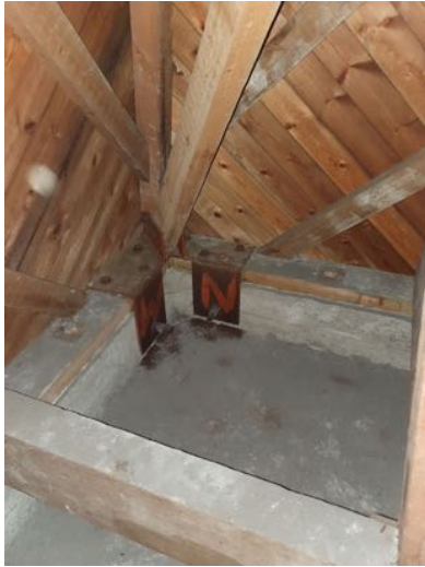
a) Holding down brackets
