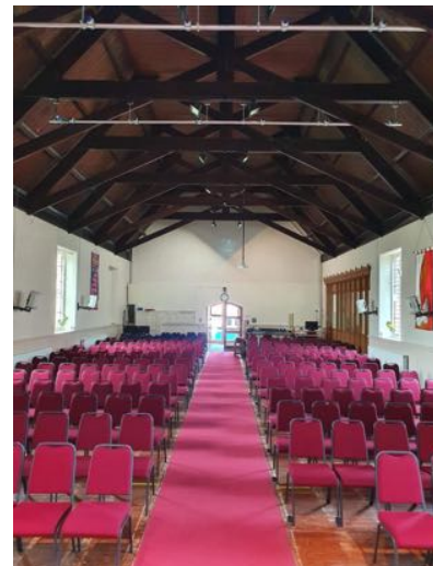
b) View from the Chancel towards the west-end entrance.
