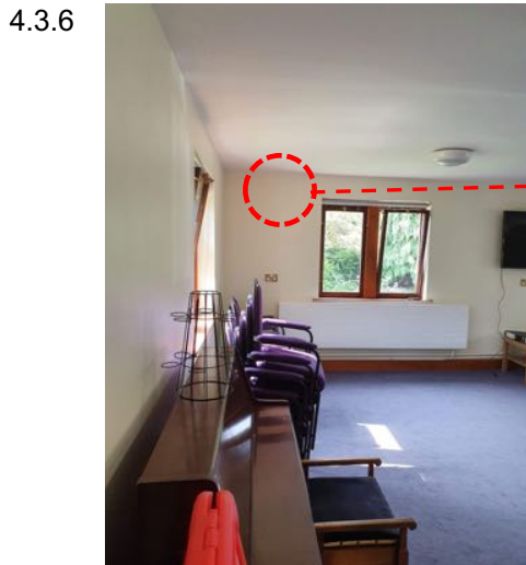
a) Cracked plaster in SW corner
