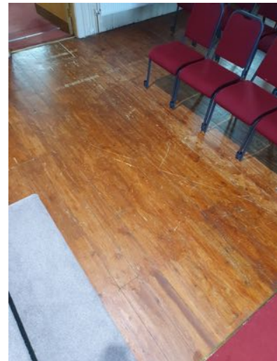
b) Pine boarding is heavily worn in places but remains serviceable.
