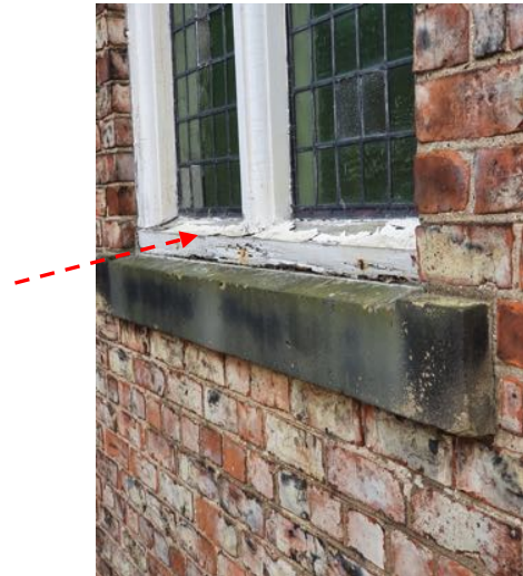
b) Replace rotten cill to window in the north gable elevation.
