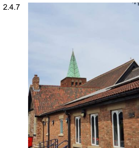
a) Shallow pitched Community Hall roof intersects with the west slope of the Library roof.
