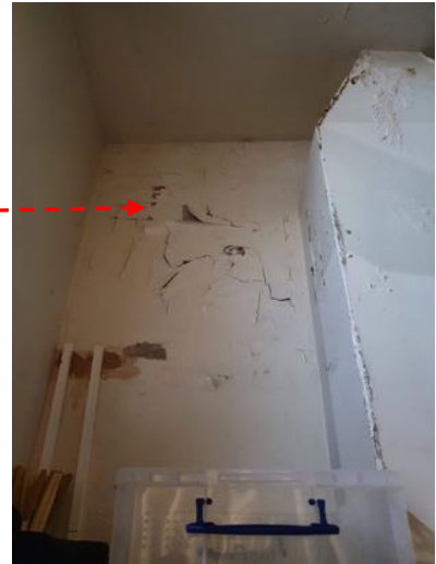
b) Corroded plaster beads and flaking paint work to be investigated.
