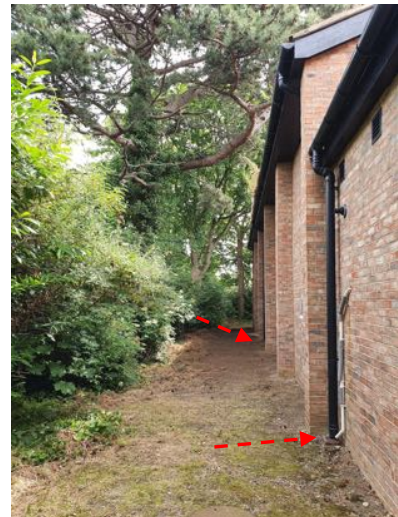
b) Check gullies capture discharge from the large north slope of the Hall roof during heavy rainfall.
