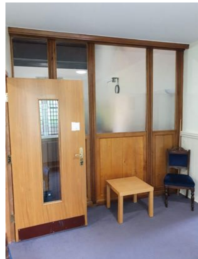
b) Glazed timber framed screen separates the Office/ lobby from the Nave.
