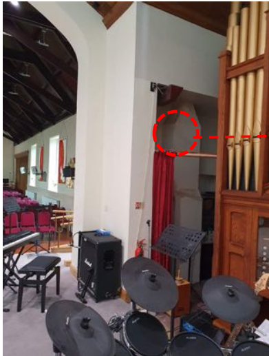
a) Plastered buttress from the original build.
