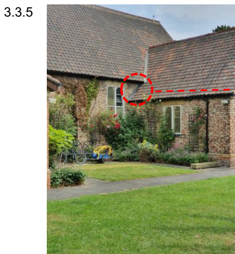
a) Library roof intersect the south slope of the Nave and forms an abutment at against the brickwork.
