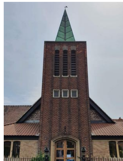
b) West elevation. The Tower is built onto the gable end of the original Church Hall/ Nave. The two roofs of the Narthex (1993) abut the Tower at low level.
