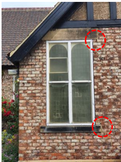
a) Mortar loss at the head and cracking around the cill
