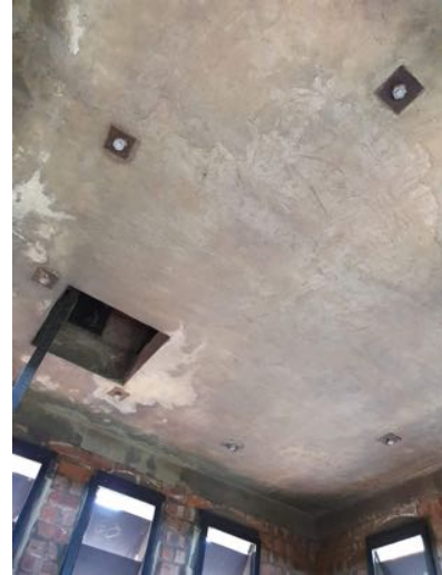
b) Bolt fixings anchor the spire structure roof.
