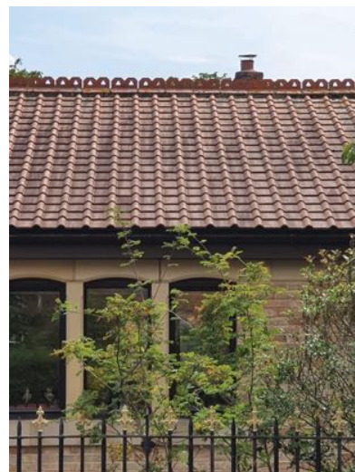
b) Single roll clay tiles with decorative ridges.
