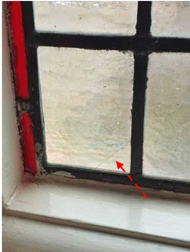
a) A minor crack to a pane in the north alcove.
