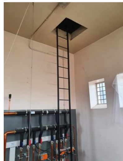
b) Ladder access to Belfry.
