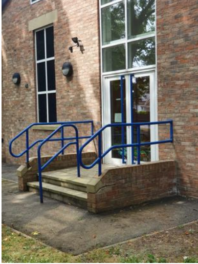
a) Cracked bed joints
