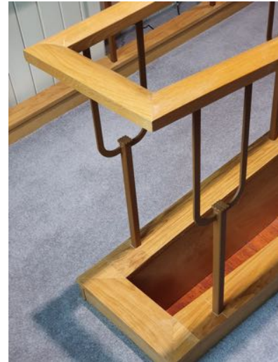
b) Ramp handrail detail
