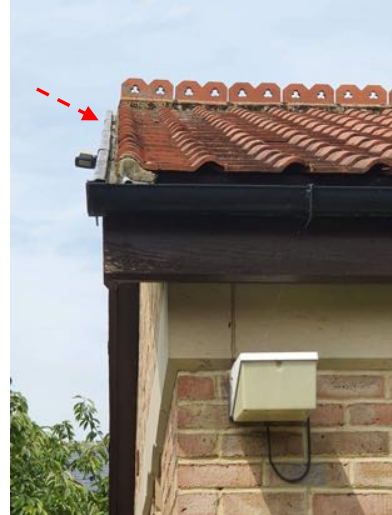
b) Lead lined secret gutter to south Gable of the Meeting Room.
