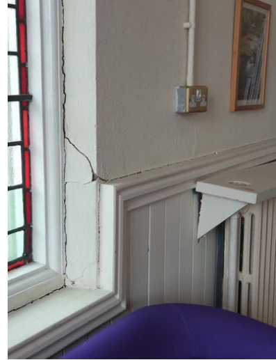
b) Cracked plaster reveals
