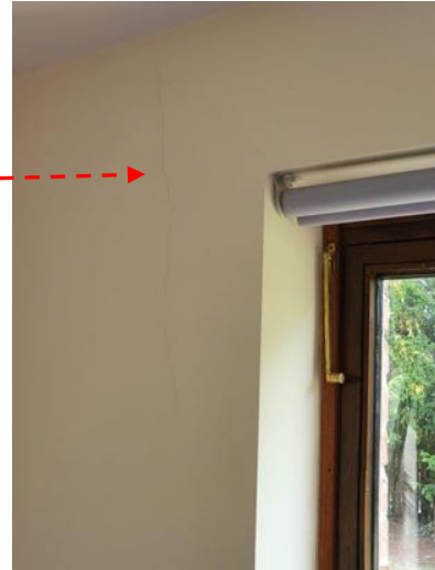
b) Crack to be monitored.
