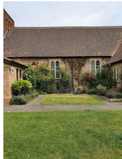
b) South elevation. Secondary glazing is unsightly.
