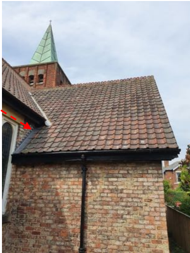
a) Replacement lead where the Office roof abuts the Nave.
