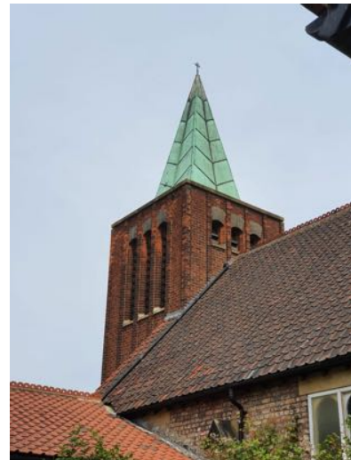
b) A rainwater pipe which drains the Tower roof penetrates the east elevation and is laid over the south slope of the Nave roof.
