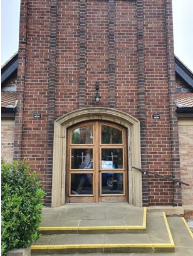
a) Oak doors to be adjusted to easy opening.
