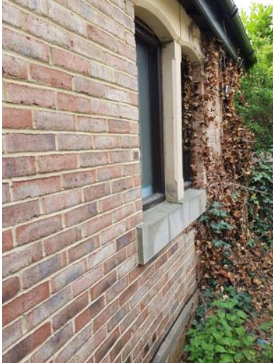
a) Cut back ivy infesting WC windows
