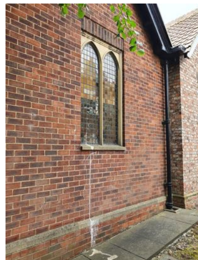
b) Organ loft gable abuts the smaller gable of the original church where a downpipe drains the valley gutter between the two.
