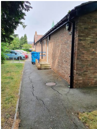
a) Tarmac has large splits, probably caused by tree roots.
