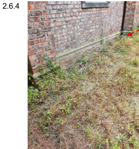
a) Gullies buried should be exposed and tested.
