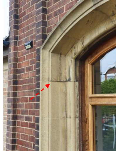
b) Washed out mortar joint and staining to the cast stone surround.
