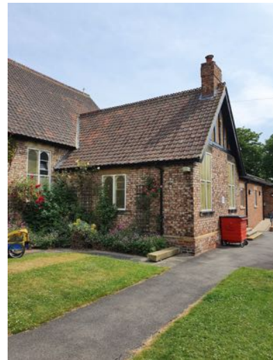
b) West slope of Library roof intersects with the Nave.
