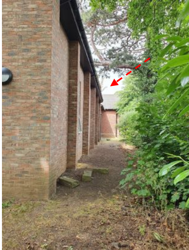
a) Vegetation growth in guttering to the north side of the Community Hall needs to be removed
