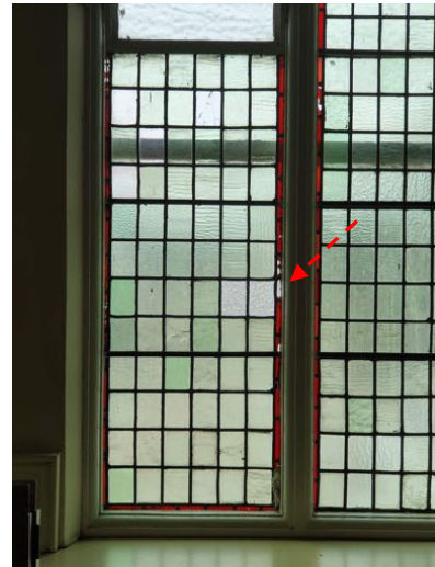
b) Numerous broken panes
