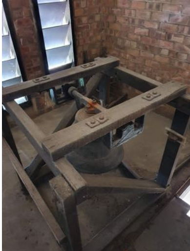
a) Bell frame and bell to be inspected by a suitable specialist.
