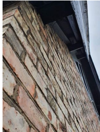
b) Bargeboard to north facing gable end.
