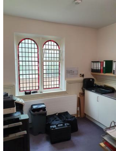
b) Leaded windows in external walls with dado panelling.
