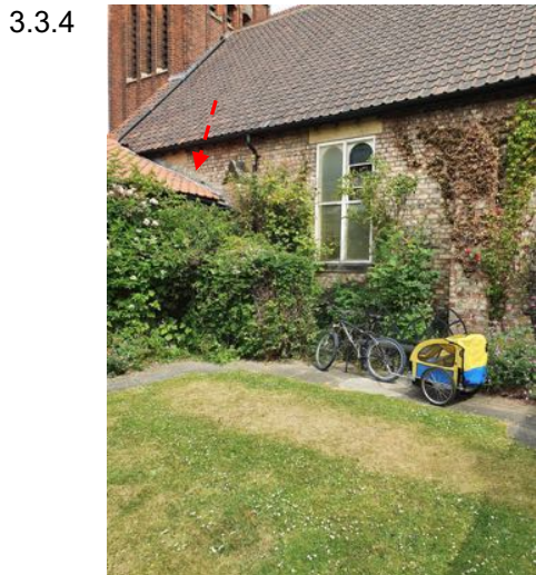
a) Lintel visible where original window was blocked
