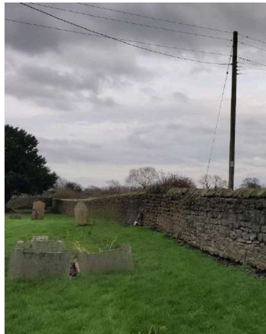
14. Sinking graves SE of Vestry reportedly due to archaeological remains, but could also indicate a localised drainage issue.
