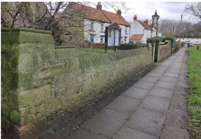
40. W boundary wall
