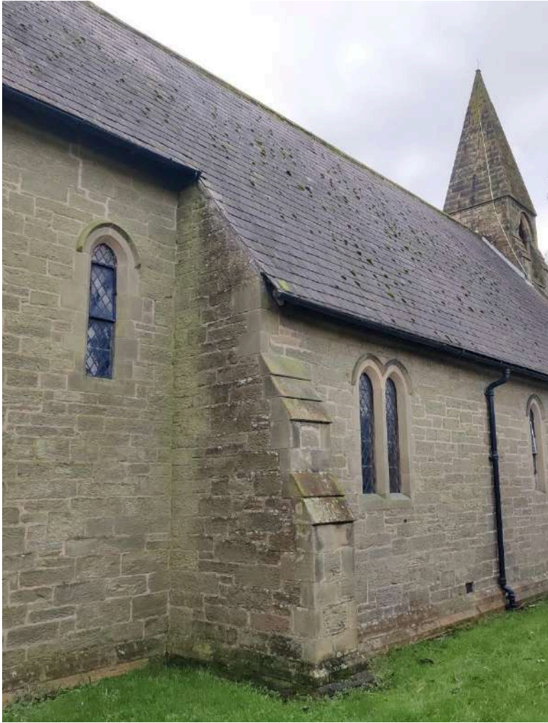
19. Chancel & Nave N roof slope.
