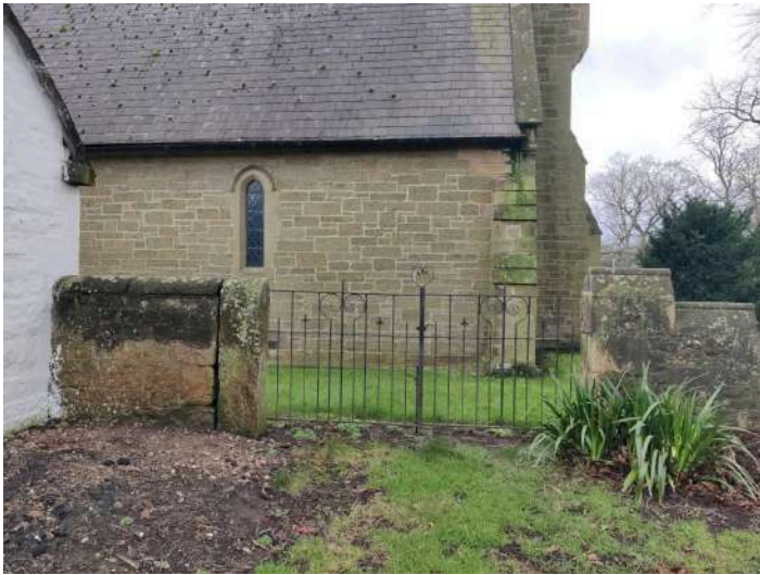
38. NW boundary wall and gate
