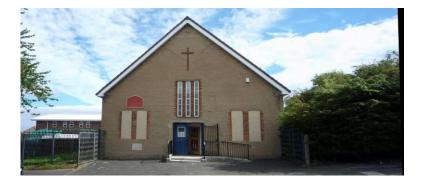
Diagonal cracking below the apex which has been botched with cement mortar. Slight cracking also above the central window and below the rendered lintel where one brick is also pushed in (odd!) and cracking to the piers either side of it.
