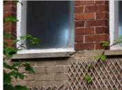
Comprises five bays. Most of the lower areas of brickwork are obscured by planting. The windows throughout are in poor condition in that their decoration has broken down. Some of them are glazed in polycarbonate and some are clear glazed. There is putty pointing missing to them and these all need a major overhaul.
