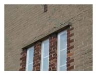
The door lintel seems to be a new replacement so perhaps we are looking at historical cracking with a touch of movement due to the new lintel settlement- so it's now settled?
