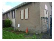
East return – damp staining on the wall as a result of blockage of the gutter above and slight open joints at previous gutter positions.
