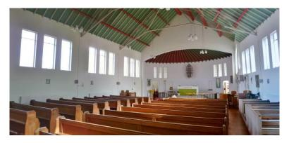
Light single open space, metal tie roof of three trusses with exposed ridge purlins and rafters with good decoration scheme to it. Boarding in between the rafters showing some slight ripple of the paper edges and one or two cracks below the upper purlin level. They are steel purlins. Walls have been redecorated and are all in fair condition and a light blue/green colour. The floor is hardwood parquet and in good condition onto solid floor. The circulation area is carpeted and in good condition.
