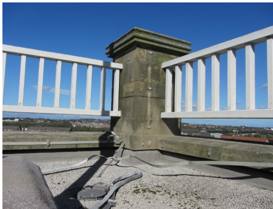
Disconnected lightning conduction tape
