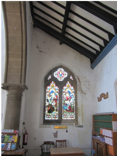
Blistering plaster and paint to North Aisle west wall
