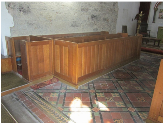
Chancel – decorative encaustic tiles
