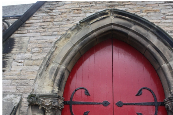
Eroded hood mould over Porch door
