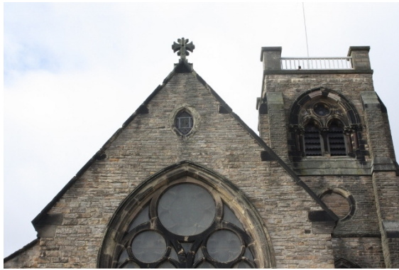
Badly eroded water tabling to Chancel gable
