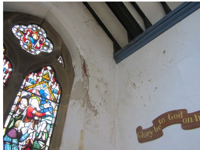
Blistering plaster and paint to North Aisle west wall
