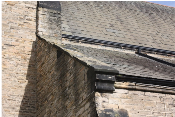
Badly eroded water tabling – Vestry/Organ Chamber
