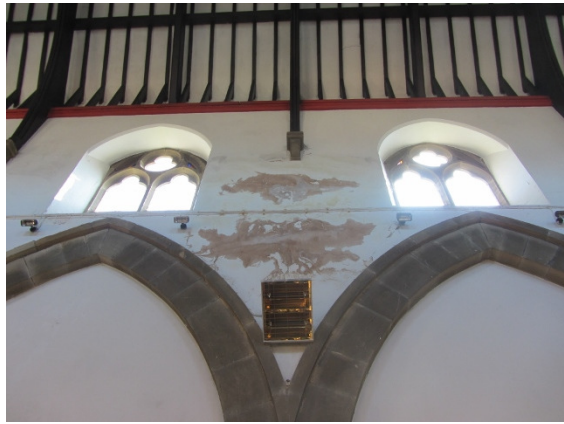
Patch of blistering plaster & paint to Nave S wall
