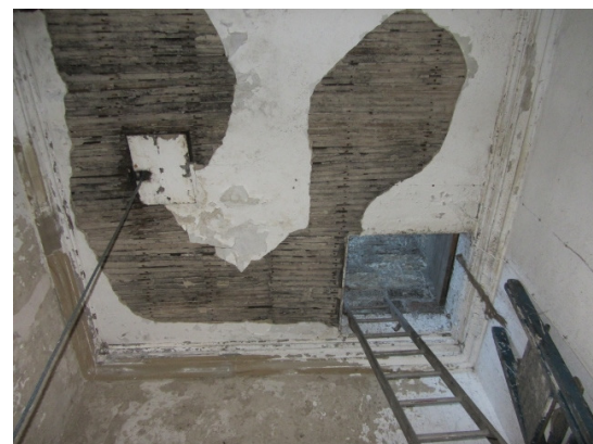
Ceiling damage at base of Tower
