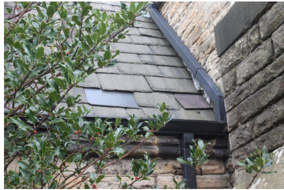
Mismatched slates to Porch roof
