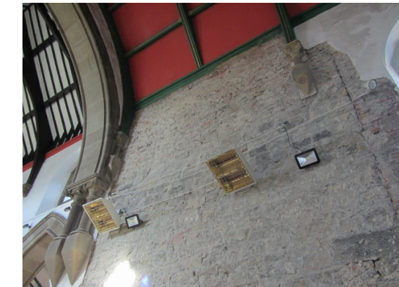
Plaster removed from Chancel north wall
