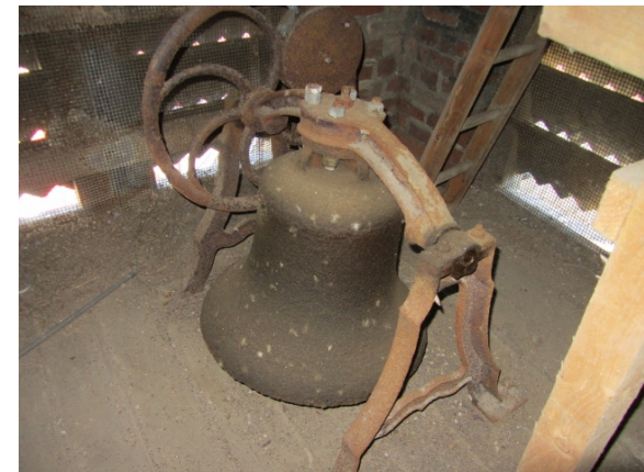
Rusting bell mechanism
