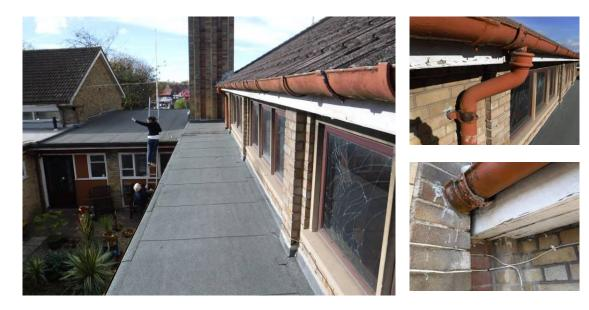
South side last looked at probably when the roof was re-covered in circa 1990's and there is a cracked downpipe and rusting gutters and fixings.
