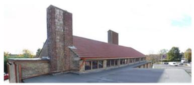
North side plastic downpipes to metal gutters, nave part restored as part of the 2016 nave roof recovering works.
