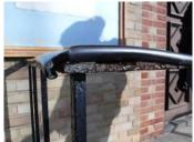
Open joints to steps and brickwork at west entrance. Handrail cover being forced off by rusting handrail.
