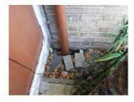
North Aisle: rusting gutters and downpipes.
