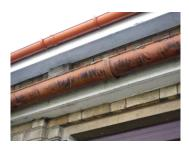
**Recommendation:** remove, renovate, repair and redecorate the rain water goods, brackets and redecorate the timber fascias. Clear out all gullies and check for free running, consider mesh covers.
