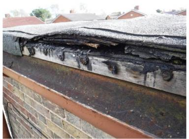
Roof is in poor condition and clearly has been over felted in the past, it is laminating at the edges, lots of hardboard showing that has expanded. The flashings to the gable are ok.
