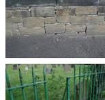
principle issue is that the two trees on the boundary are effecting it now, they are beginning to bulge the wall out and the eastern most tree is pushing it into the lamp standard that is taking the three phased power line by the bus stop.
