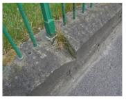
Further along the railings are decorated but rusting in places. The copings are broken due to iron rusting. Along the length of the wall there are buckles and twists to it. It is generally ok but it has had some knocks. It could really do with a repoint, the
