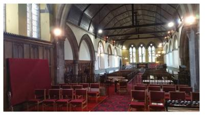
The walls are all painted apart from the stone dressings to windows and doors, the general painting scheme is good. Within the nave, the west wall at high level looks a little poor but I think what is happening is it is catching a lot of dirt that is up in the attic of the roof, so when the wind blows it dusts down the wall and there's little that can be done other than redecorate.
