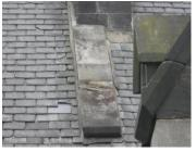
of the roofing is ok. The mortar haunching over the memorial chapel water table is ok.
