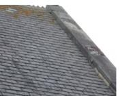
**South side** - has about three missing tiles. The water table at the west mortar pointing is breaking down, it doesn't look as if there is lead behind it, and it is breaking down at the apex.
