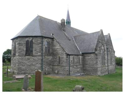
This shares a roof that sweeps over the Memorial chapel. At the junction of the nave the wall head comes through to create a coping this coping the condition of the mortar flaunching against the coping isn't great at the foot on the nave side it is coming away, this has the chimney which is redundant and can be cleared away in time, the top surface of the water table looks poor. There is damp inside at this point.
