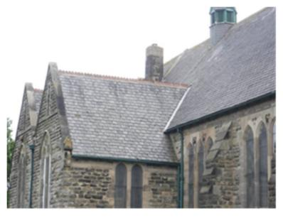
The western most transept has an ill matching ridge at the apex of the valley flashing and a collection of debris at the foot of it.
