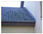
**W.C.** – Has a lean-to slate roof, this is a little bit scruffy with arisings off the main roof works and just needs to be tidied up, has mineral felt flashings elsewhere the flashings are in lead.
