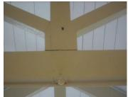
Five trusses form the main nave space, supporting purlins onto ceiling boarding. Every second truss has a projecting supporting member going down into the wall head and the truss condition looks fine. There is some slight possible deflection to the penultimate s beam as the gap has opened up on the truss postbut looks historic. Is there rot at the purlins at the n end? Or is this decoration marks?
