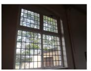
**Vestry** – Metal single glazed windows with obscure glazing apart from one in clear, possibly as a result of a break-in in the past. These also have top vents but they are none operating. Slight marking of rust coming through but no attention required.
