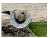
Soil pipe to northeast appears to have most clamp fixings missing, and is in a dangerous condition.
