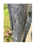
2. Lead-lined stone chute blocked on south side of Nave.
