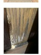
Vestry door D5 has cracked outer plank adjacent cylinder lock, otherwise in good condition.
