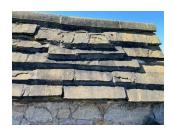
Porches have stone slates, water ingress and daylight visible through southwest roof. Investigate and repair as necessary.
