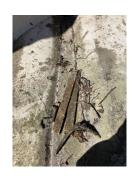
2. Bird netting has fallen off southeast turret. Also, fixings are into asphalt.
