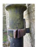
Blocked and loose asbestos shoe from Priestman Hall roof discharge into north Porch gutter.
