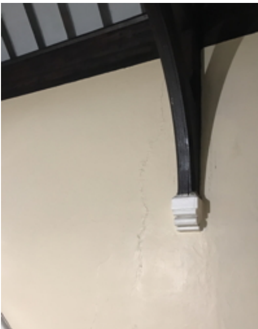
Crack to South Wall
