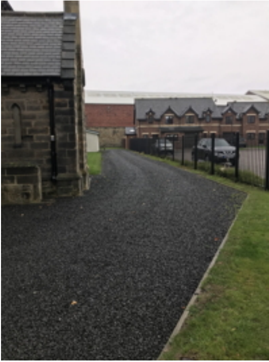
Gravel Driveway to North Elevation
