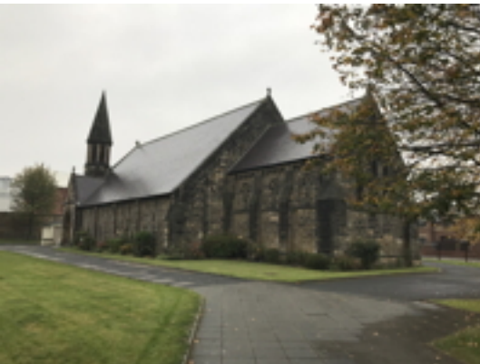
Paving to South East Corner and Planting Bed to South Elevation
