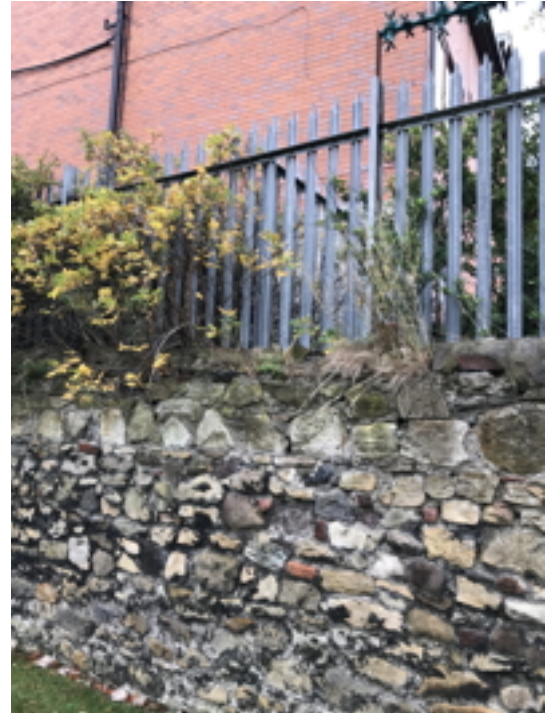
Vegetation to South Wall Copings
