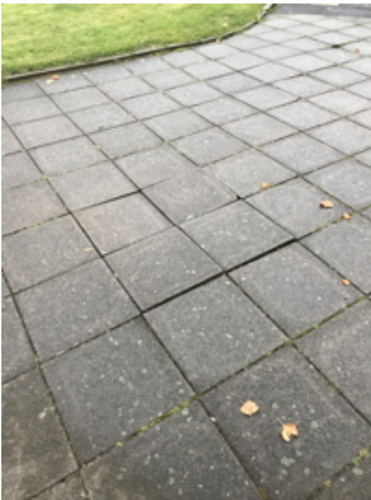
Area of Loose Paving on Driveway to South East Corner
