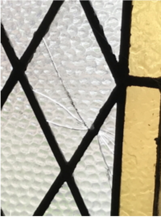
Cracked glass panes visible from organ loft
