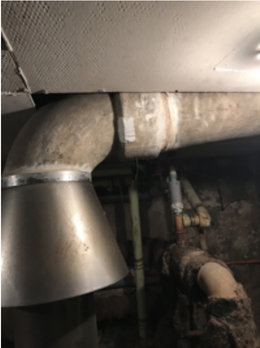
Boiler Flue and Boiler Chamber Ceiling
