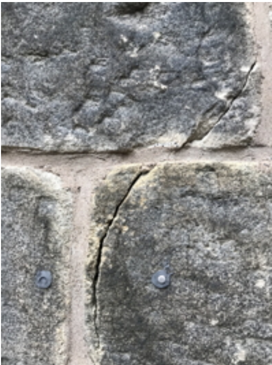
Crack to North Chancel Wall
