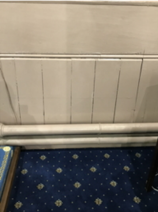
South Aisle Panelling that extends throughout the Nave
