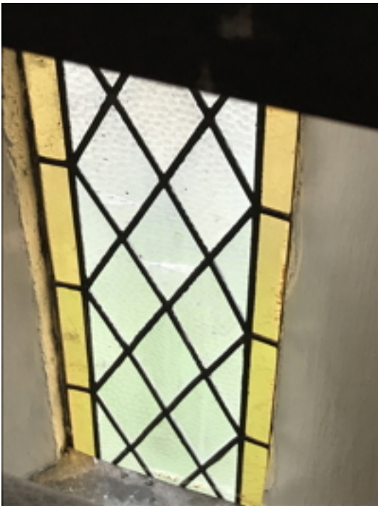
Cracked glass panes visible from organ loft
