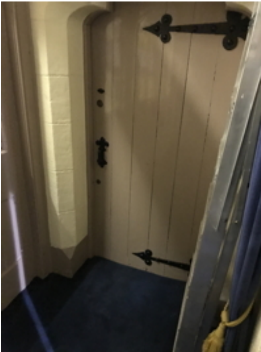
Porch/Tower Staircase Door
