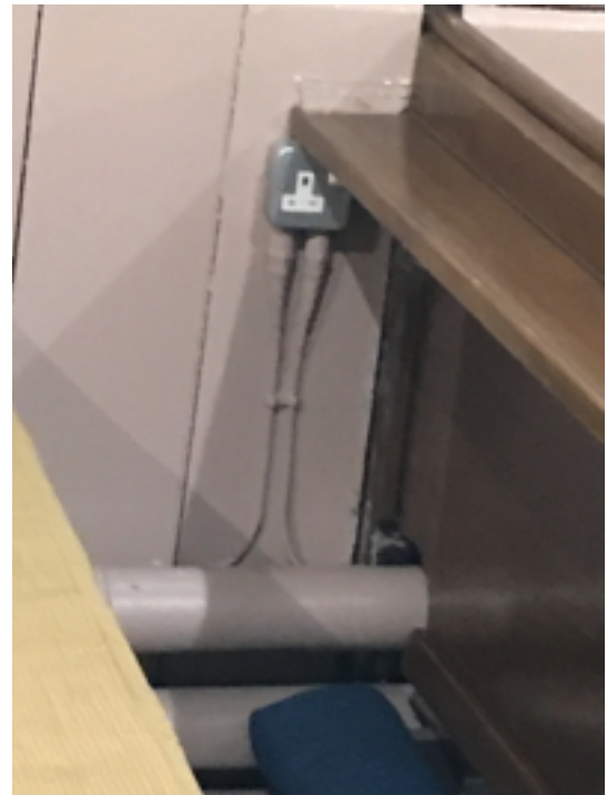
Perimeter Heating Pipework
