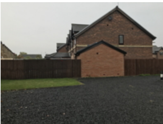
North Boundary Fencing and Garage
