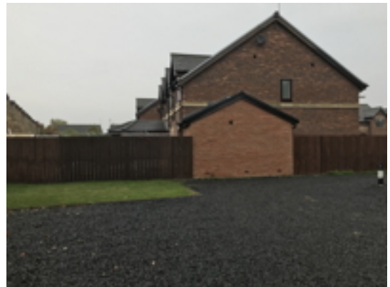
Gravel Driveway to North West Corner
