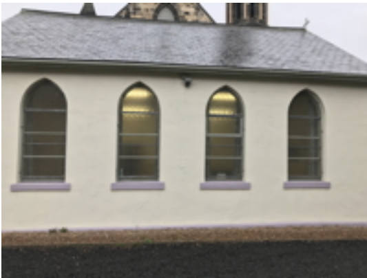
Meeting Room West Elevation Windows
