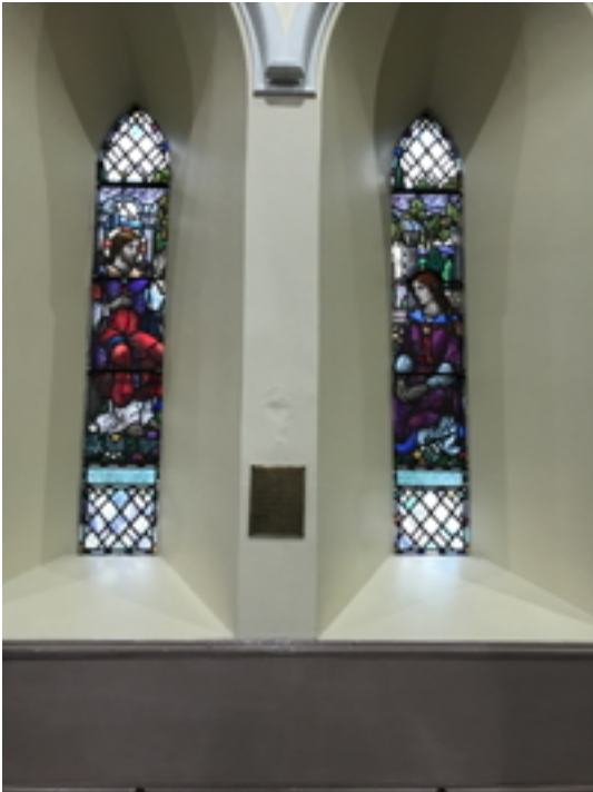
Typical South Aisle South Elevation Windows
