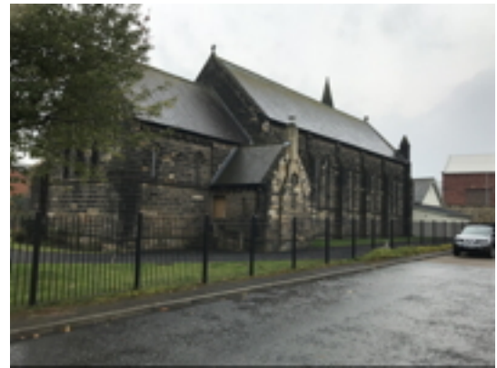
North Boundary Railings
