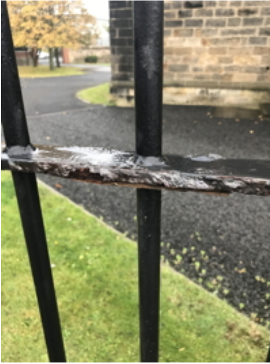
Rust to North Boundary Railings
