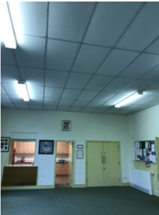
Meeting Room looking towards Kitchen and Large Store
