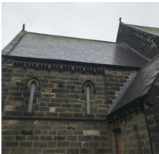
Chancel and Vestry Roofs
