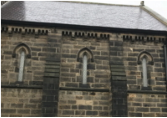
Chancel South Elevation Windows
