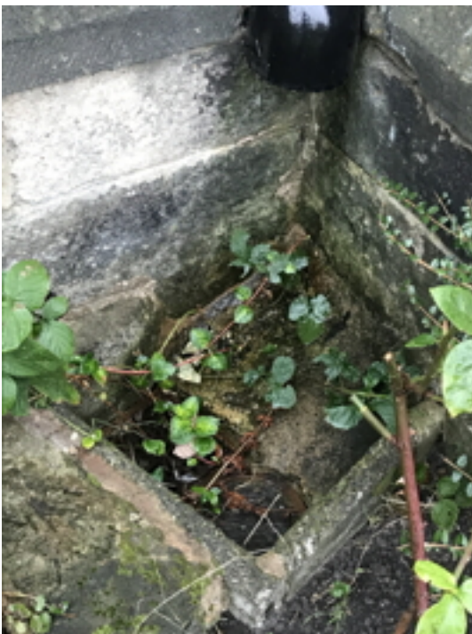
Vegetation starting to grow around gully
