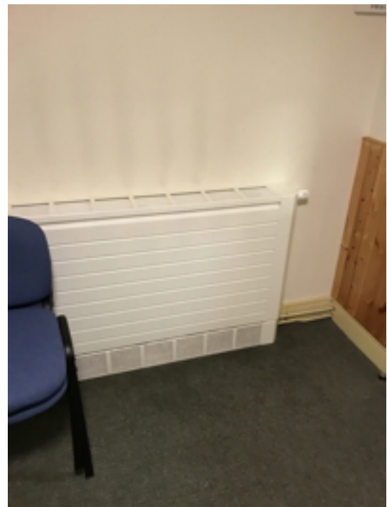
Typical Hall Radiator
