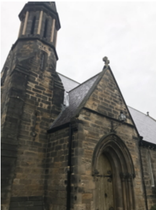
Vestry Water Tabling
