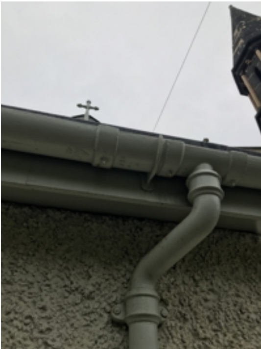
Rust spots to Hall Gutters and Rainwater Pipes
