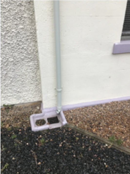
Hall West Wall UPVC Rainwater Pipe
