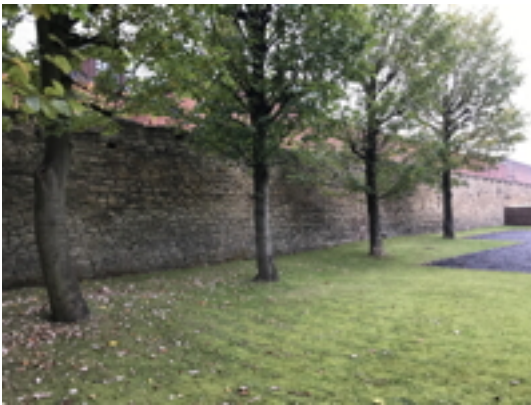
West Boundary Wall
