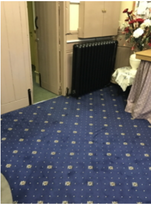
West End Nave Radiator
