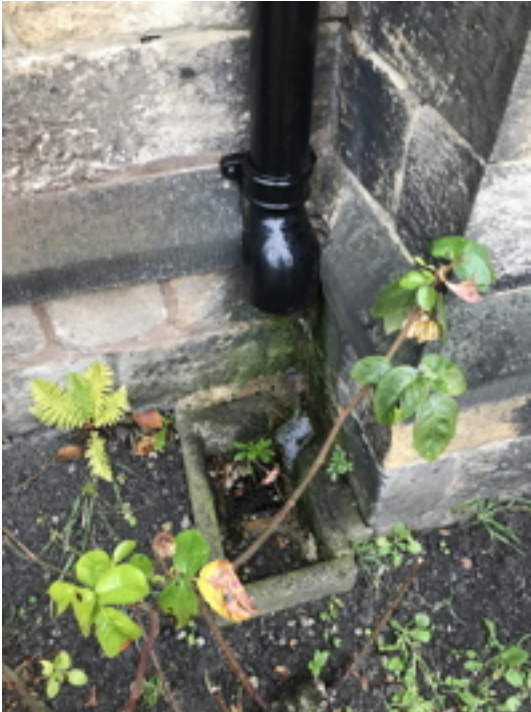
Vegetation starting to grow around gully
