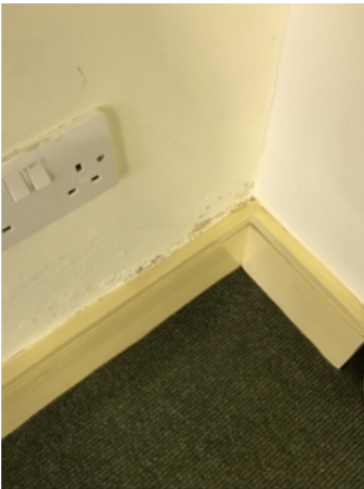
Typical Hall Damp
