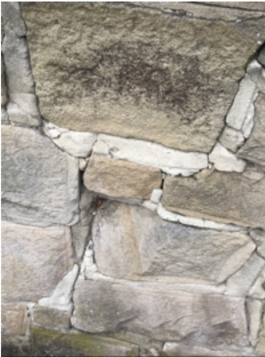
Loose Pointing to East Wall Stonework
