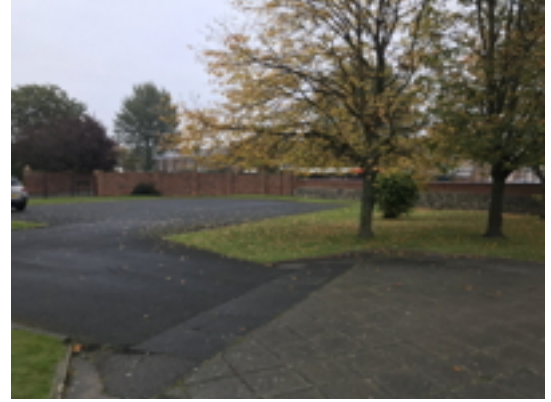
Tarmaced Parking Area to North East Corner
