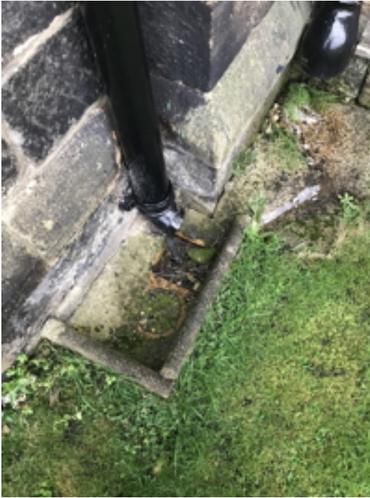
Debris around gully and rainwater pipe discharging over concrete.
