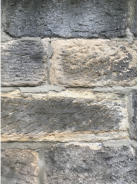
Possible cement Mortar pointing to Nave North Wall
