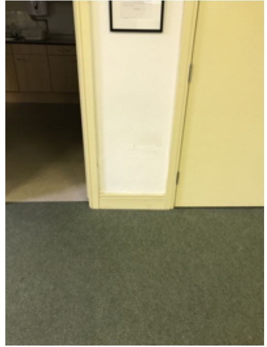
Hall carpeting and sheet vinyl flooring
