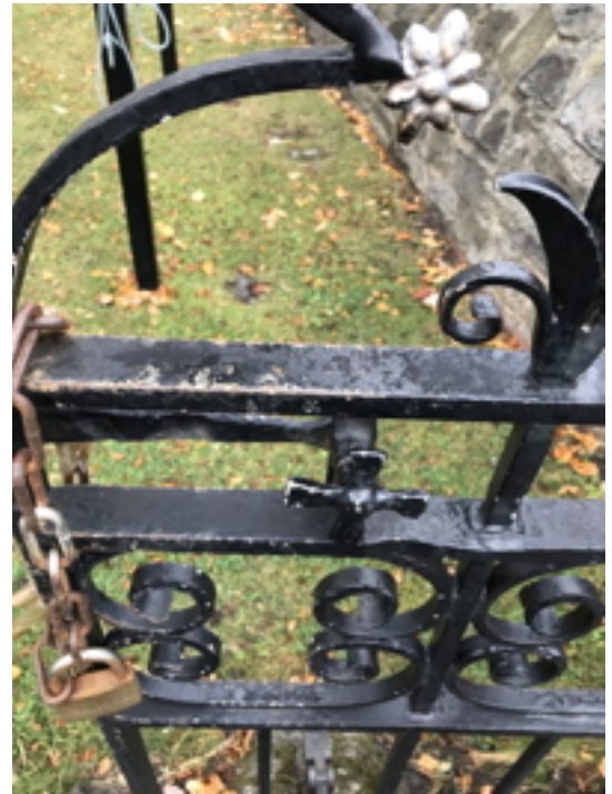
Gates Requiring Redecoration
