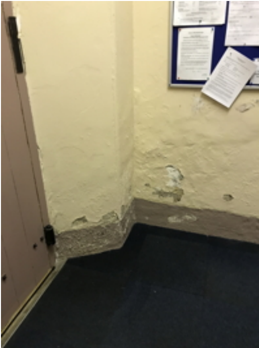
Porch West Wall Damp
