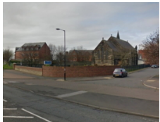
North East Corner Brickwork Wall and Stone and Brickwork East Boundary Wall
