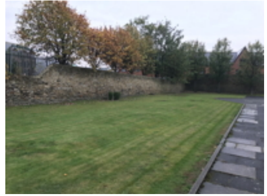
South Boundary Wall West End
