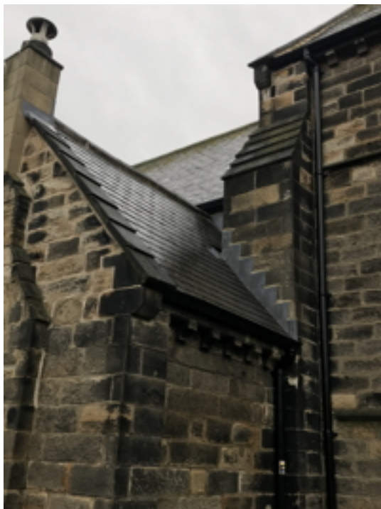
Vestry and Nave Rainwater Pipes and Gutters
