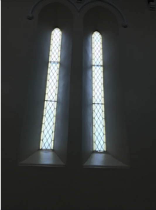
Typical Nave North Elevation Windows
