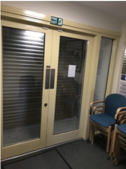
Hall Glazed Doorway and Shutter
