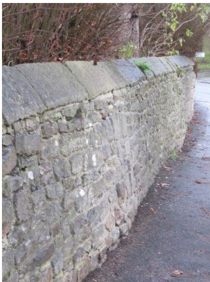
Bowing wall around tree to Southern boundary
