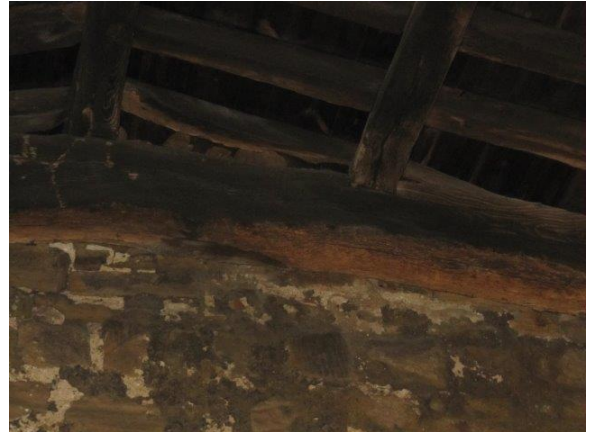
Roof trusses and rafter to tower roof
