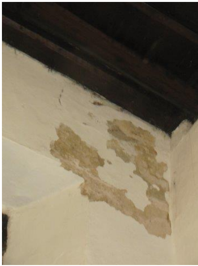
Loss of limewash to West wall of North Aisle
