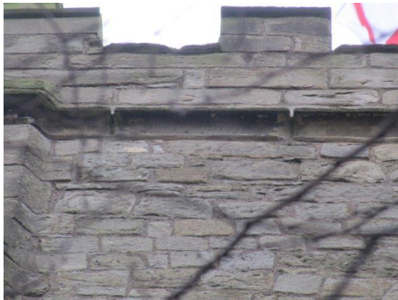
Open joints to tower string course
