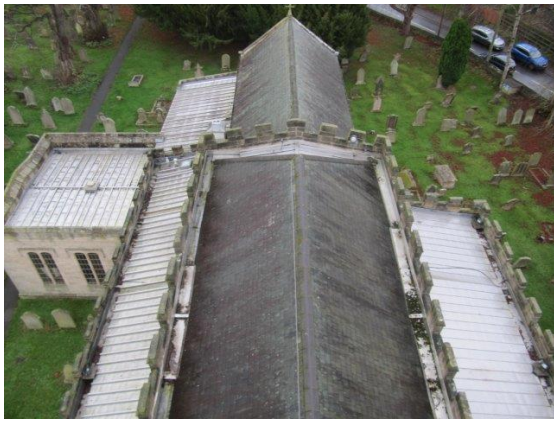
General view of main roofs from tower
