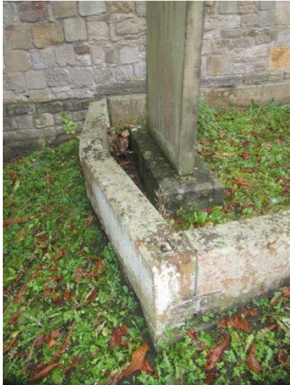
Unstable grave edging to the East of the steps/entrance South Aisle
