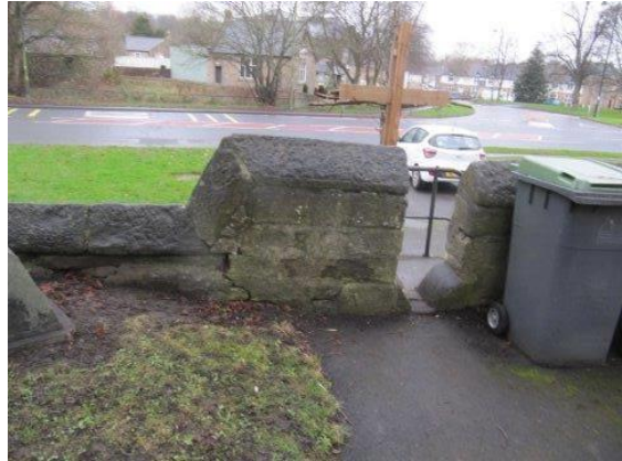
Cracking wall to the South of the main
