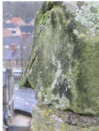
Cracking to tower parapet to be repointed or grouted
