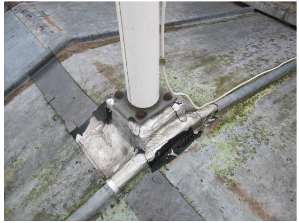
Failing modern flashings to base of flagpole
