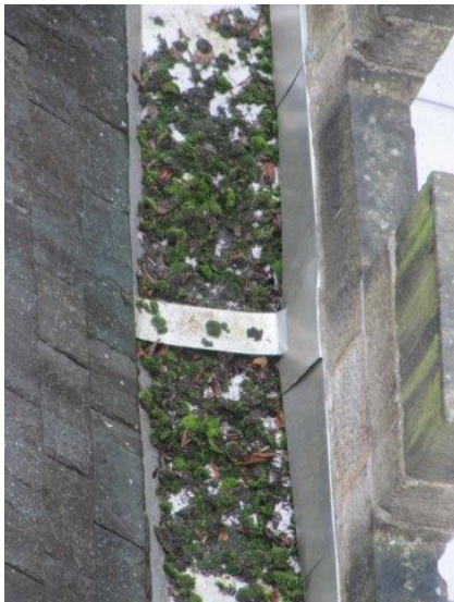
Buildup of debris in aisle gutter
