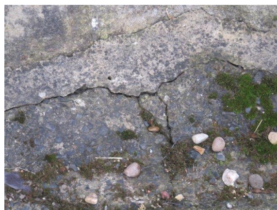
Cracking to concrete skirt at the base of the tower
