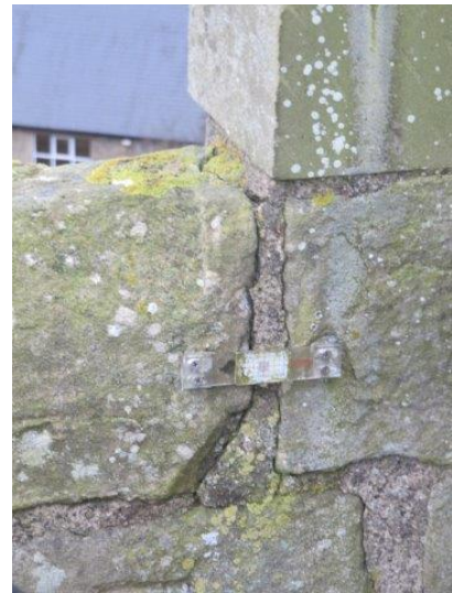
Cracking to tower parapet to be repointed or grouted
