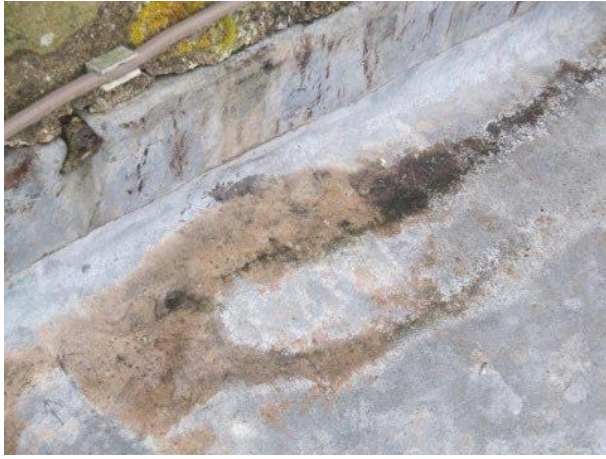
Raised leadwork to tower roof
