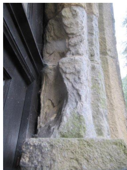
Weathered stonework to main porch
