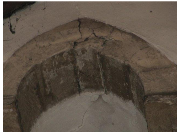
Cracking of arch over left light to East Chancel
