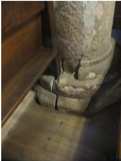
Open joints to column in North Aisle Window
