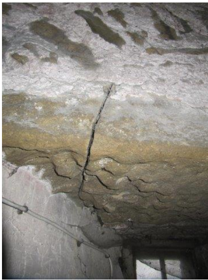
Crack to clock chamber lintel is understood to have been repaired but not repointed
