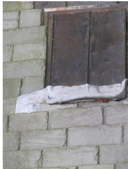
Deformed lead over hatch/old skylight
