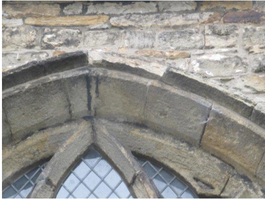
Hood moulding to window 16
