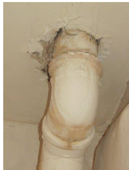
Staining around SVOP in forts floor WC
