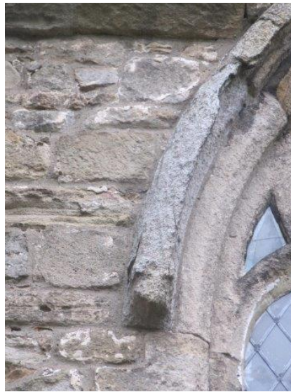
Hood moulding to window 15
