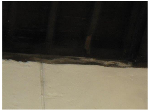
White staining to wall plate in North Aisle
