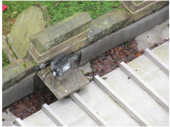
Build up of leaves in Aisle gutter
