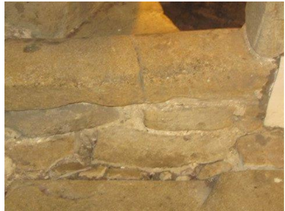
Step into clock chamber is awkward
