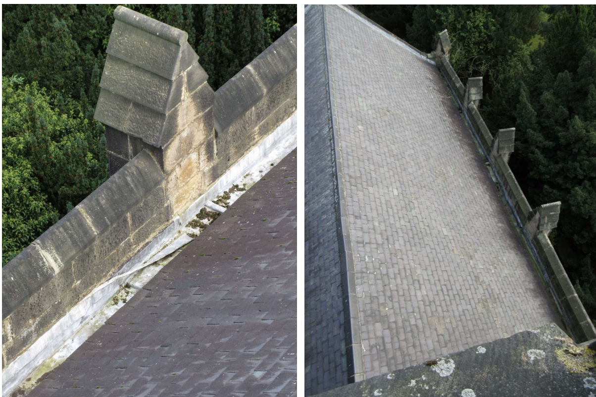
Cover flashing at centre of N Nave fallen out
