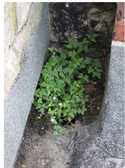
Outlet from Tower roof, before plants removed at inspection
