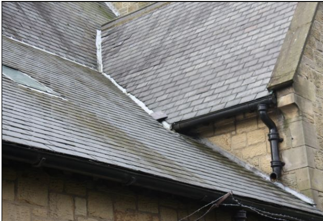
Missing slates by Organ Chamber valley gutter
