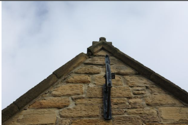
Porch gable - hard cement pointing, open joints to gable copings etc.
