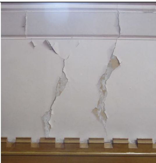
Nave walls – unsightly blistering paint
