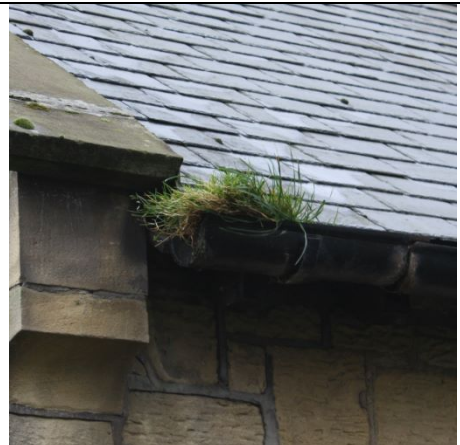
Blocked and leaking Vestry gutter
