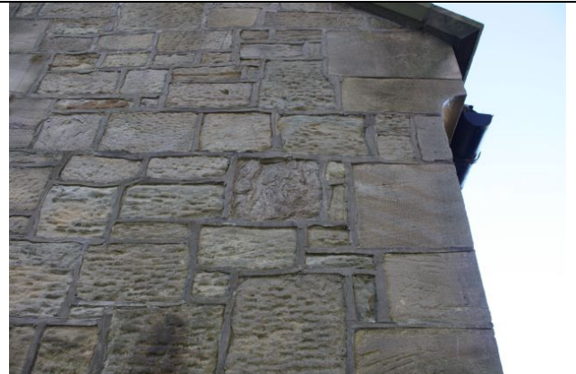
Vestry east gable – hard cement ribbon pointing
