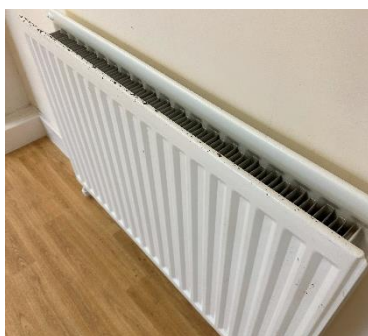
Figure 14 – Radiator Rust
