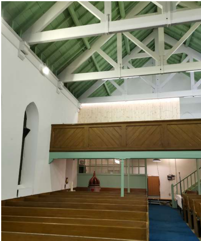
Newly painted ceiling boards and trusses - removal of fibreboard allows leaks to be noted immediately and monitored
