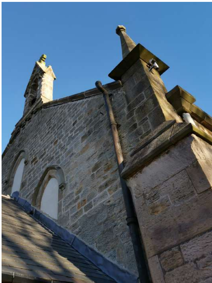
Western gable - watertabling re-bedded, gable re-pointed.
