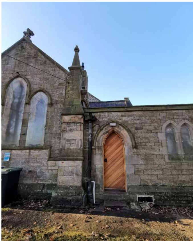
Vestry copings open, but felt over prevents water ingress
