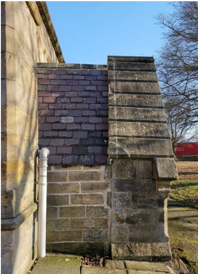
Porch re-pointed and re-roofed - grey plastic soil pipe taking rainwater from nave roof still not been resolved
