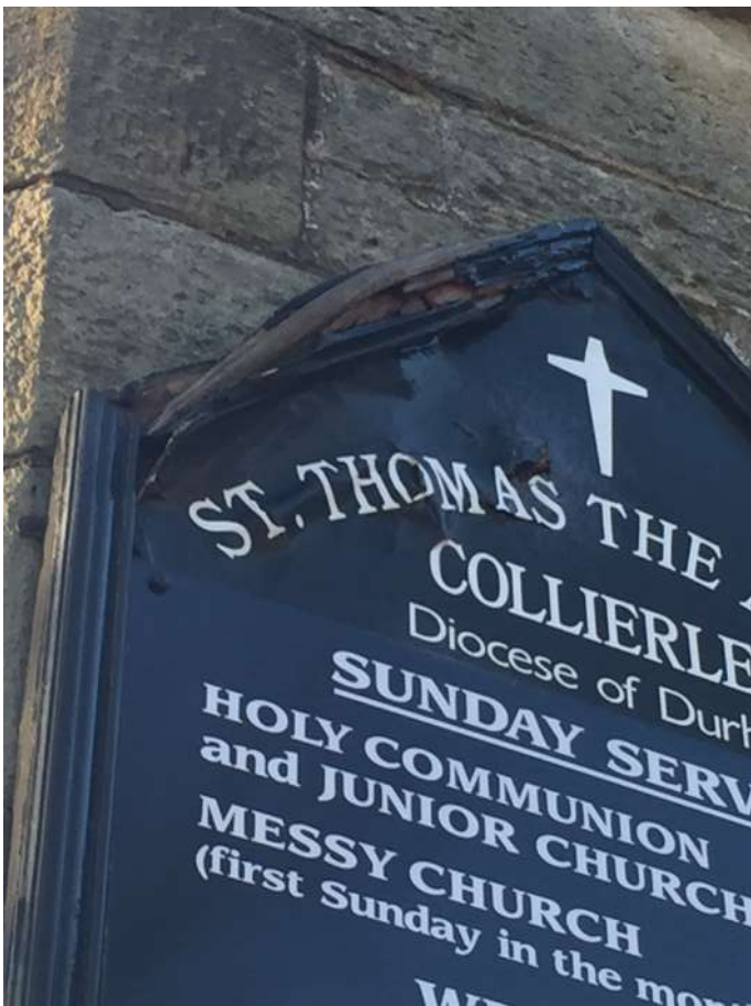
Damaged noticeboard, now required replacement, or repair
