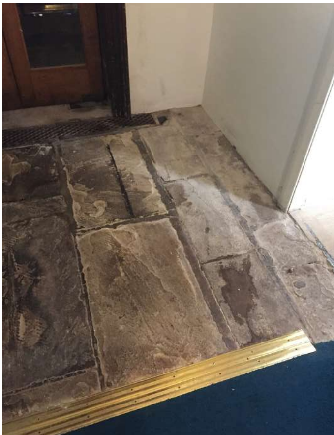
Stone flags still visible at south west entrance, before blue carpet begins
