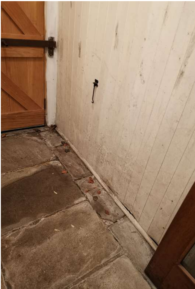
Timber panelling inside porch hiding damp masonry, restricting drying out. Damp seen on flags to floor
