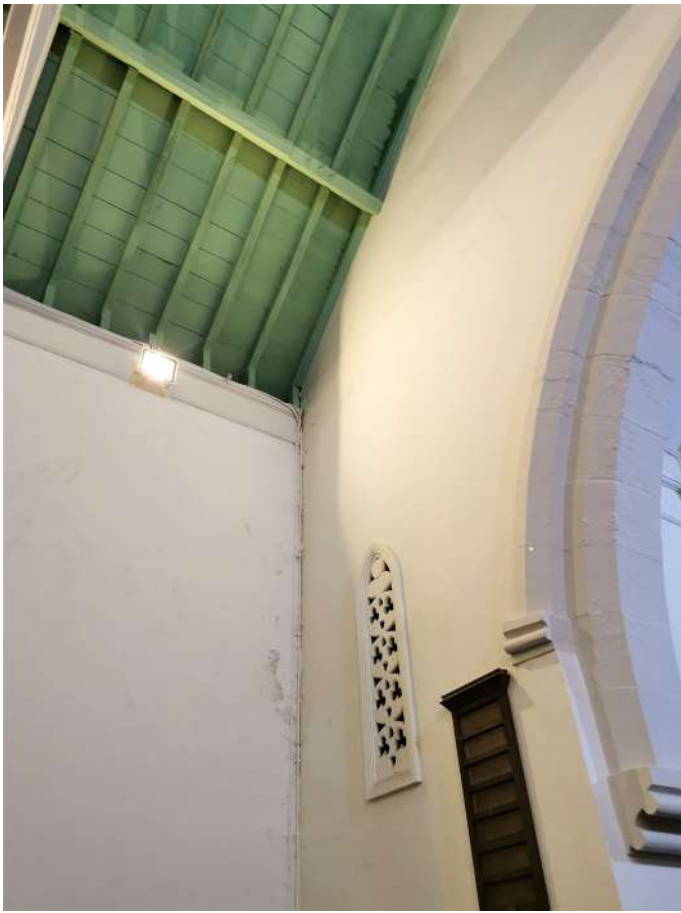
Blistering and damp in corner of north east nave - wall drying out from major long-standing water ingress, but also still signs of leaking at roof level following driving rain (above bottom purlin) despite major works to watertabling. See notes about slating in roof section
