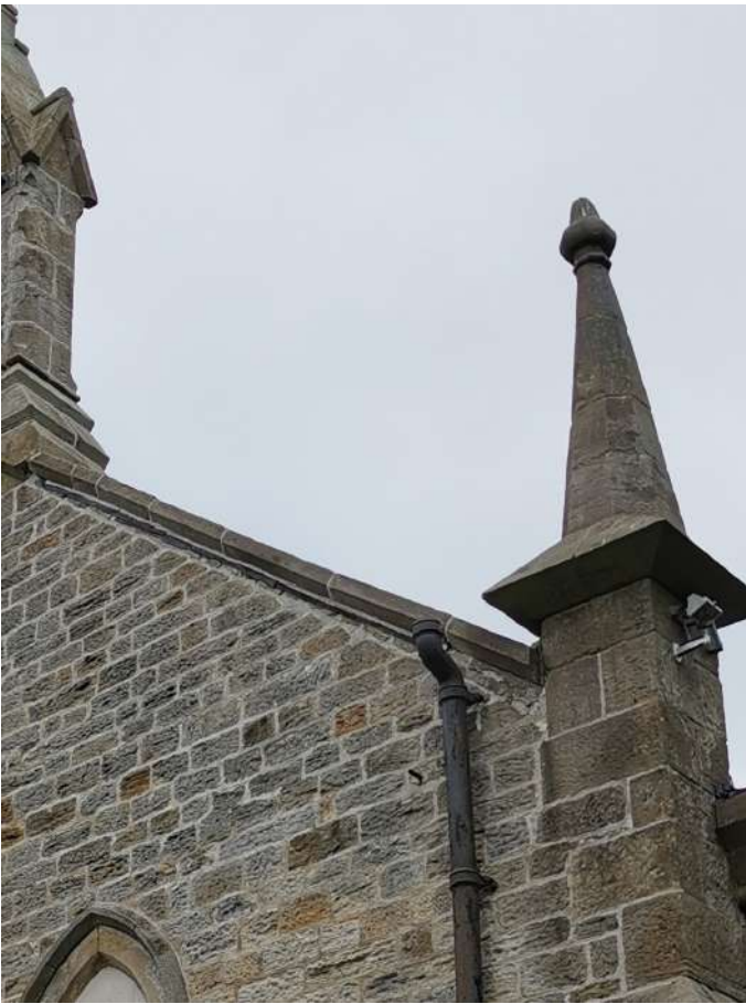
Pinnacles checked for stability, movement is notable - unknown whether there are dowels or lead joggles locating the stones - would benefit from re-building with stainless steel dowels
