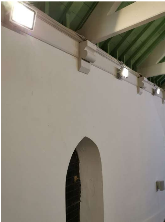
Full redecoration of plasterwork and timber roof structure
