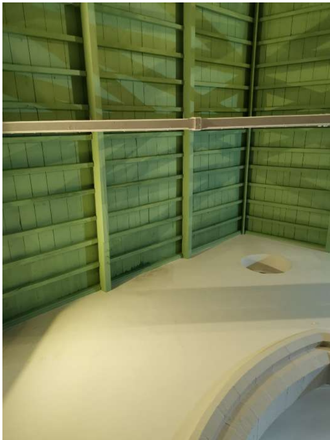
Purlin in east gable, north pitch repaired and area of sarking boards replaced where rotten
