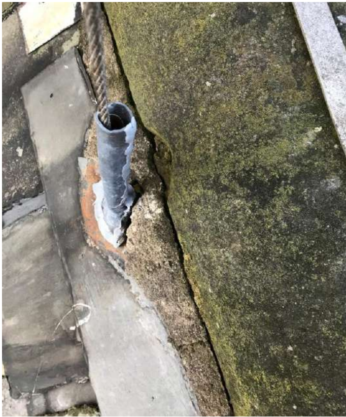
Lead sleeve taking bellrope through roof covering is inadequate - requires completely renewing during re-roofing
