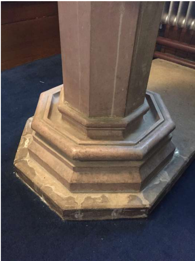
Base of font suffering from salts - surrounded by carpet, which will be having a detrimental affect
