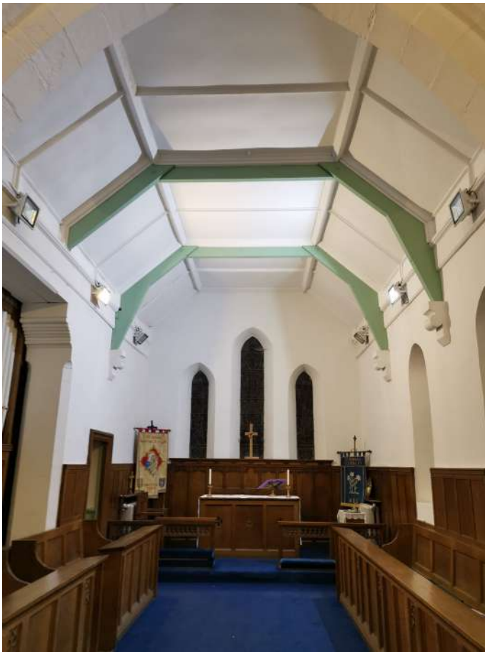
Furniture and panelling to chancel in good condition - ceiling also re-painted. Fibreboards left in situ
