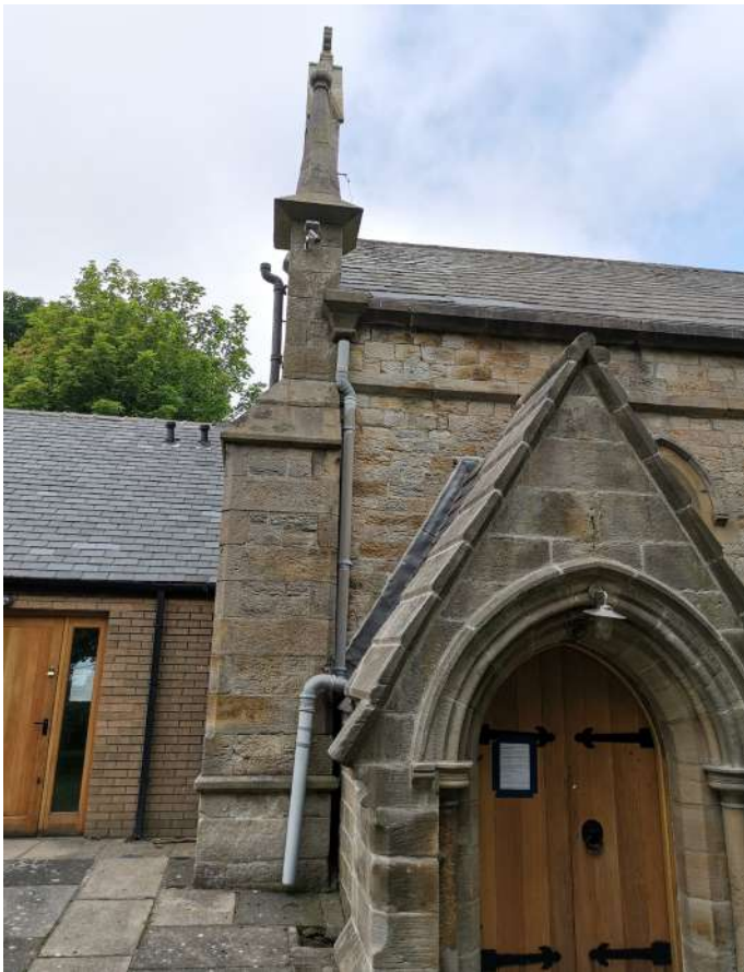
Contrived grey plastic SVP taking water from nave down and around porch and buttress - requires improvement
