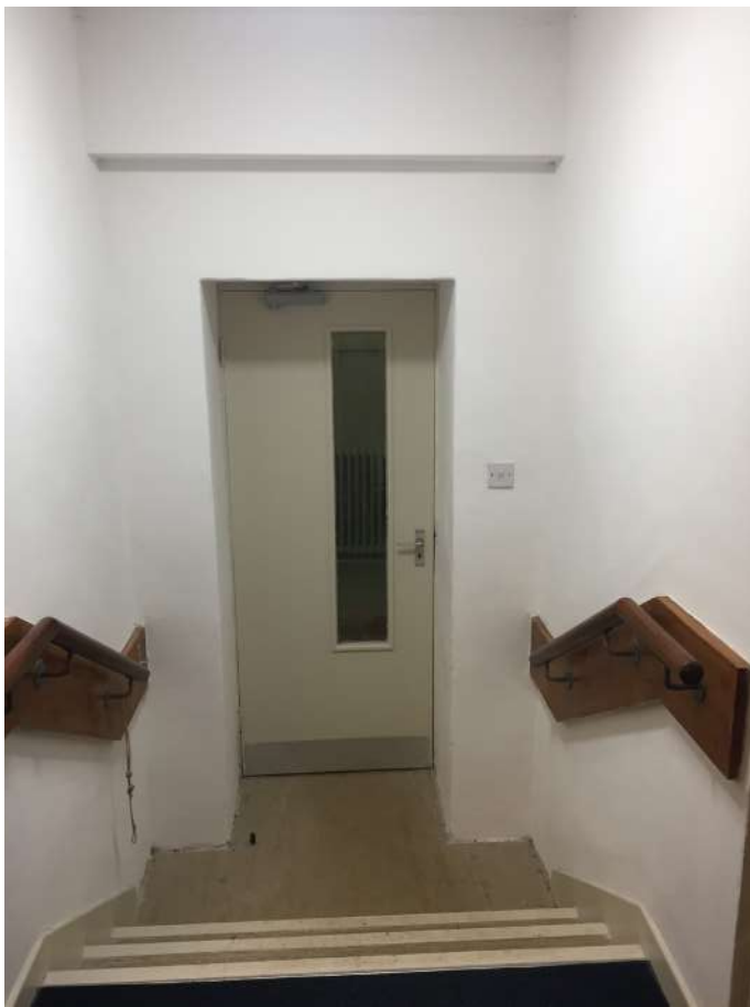
External wall to right hand side of link has been replastered in lime plaster to help deal with damp
