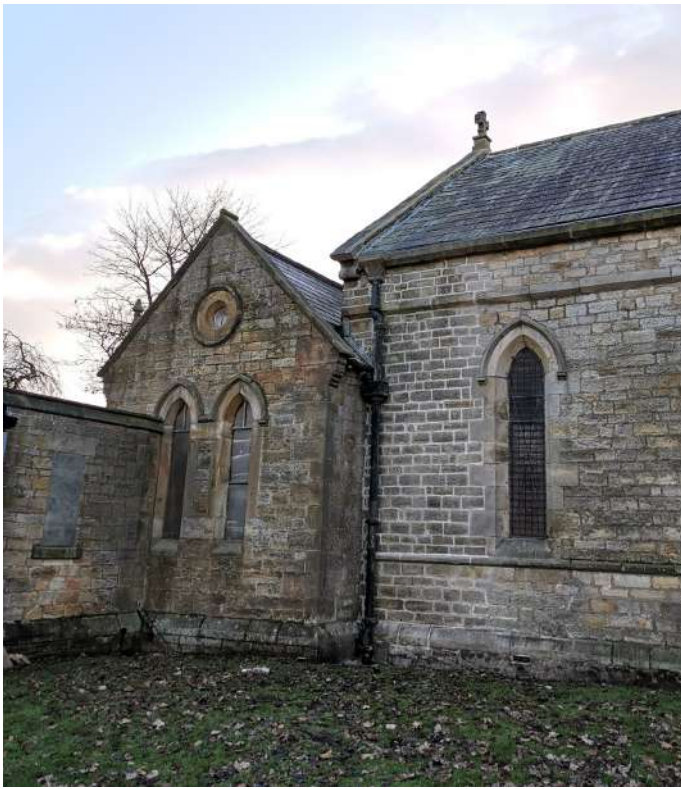
North elevation generally damp - area to east of nave repointed
