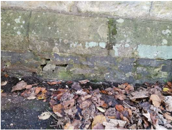
Hardstanding against base of wall is causing damp at low level, and mortar breaking up
