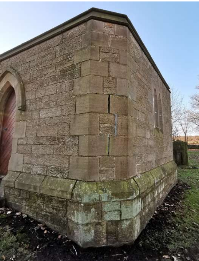
Cracking in north east vestry walling is substantial - point in lime mortar and monitor
