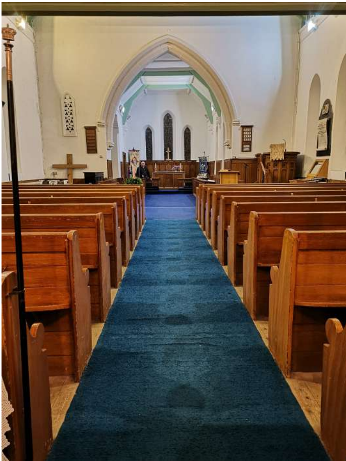
Carpet throughout, will be causing dampness within the original stone flags below
