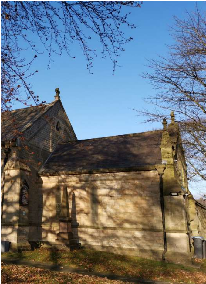
Chancel roof requires major repair, and likely re-roof
