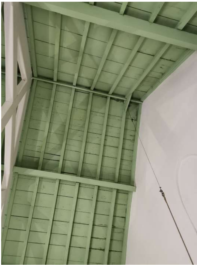
Newly plastered west gable. Extent of storage area, between gable and first truss.
