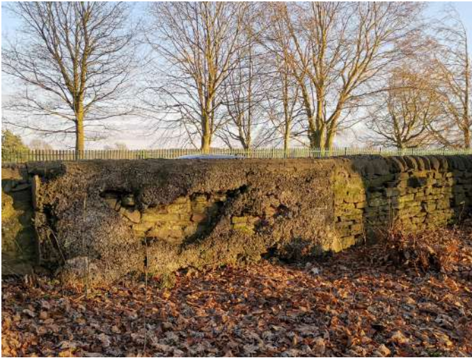
Cement render to be removed
