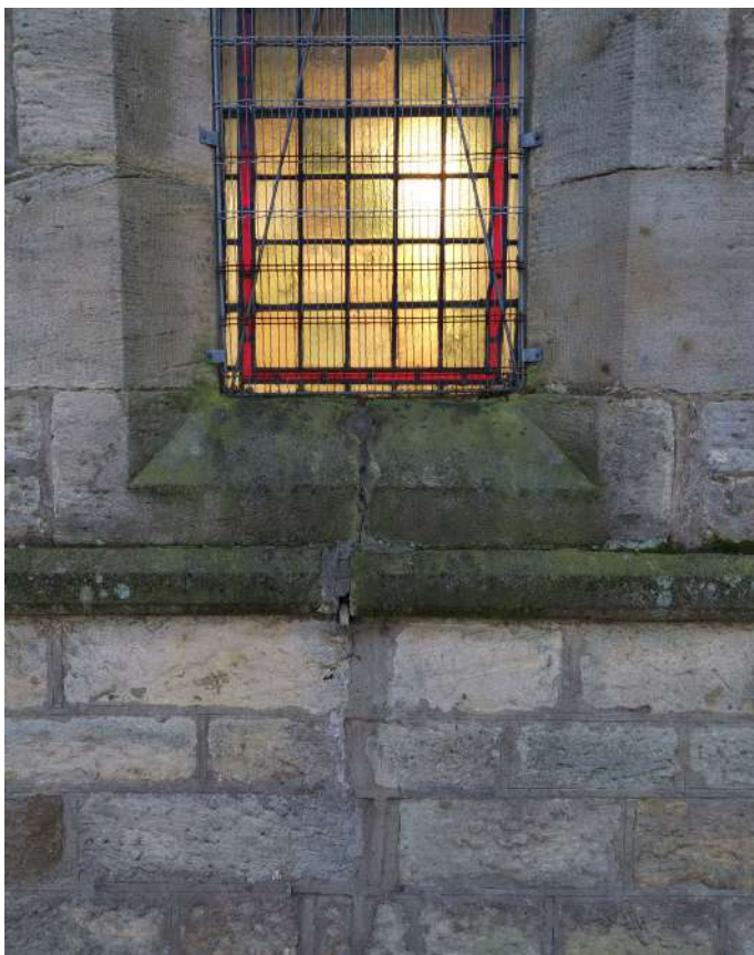
Crack through cill of middle window on north elevation of nave
