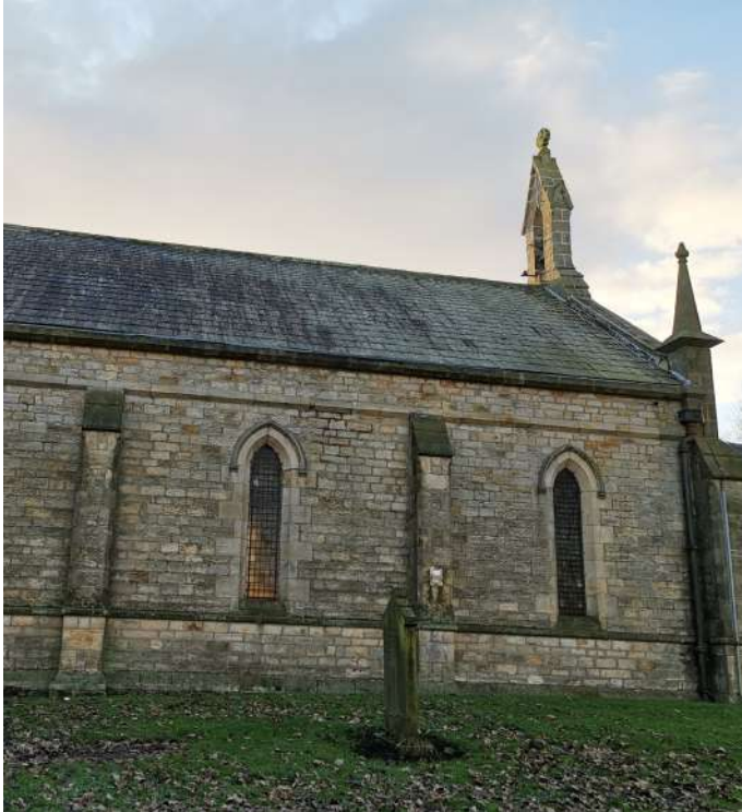
North roof pitch - repaired but still allowing water through during driving rain - headlaps only 50mm in general.
