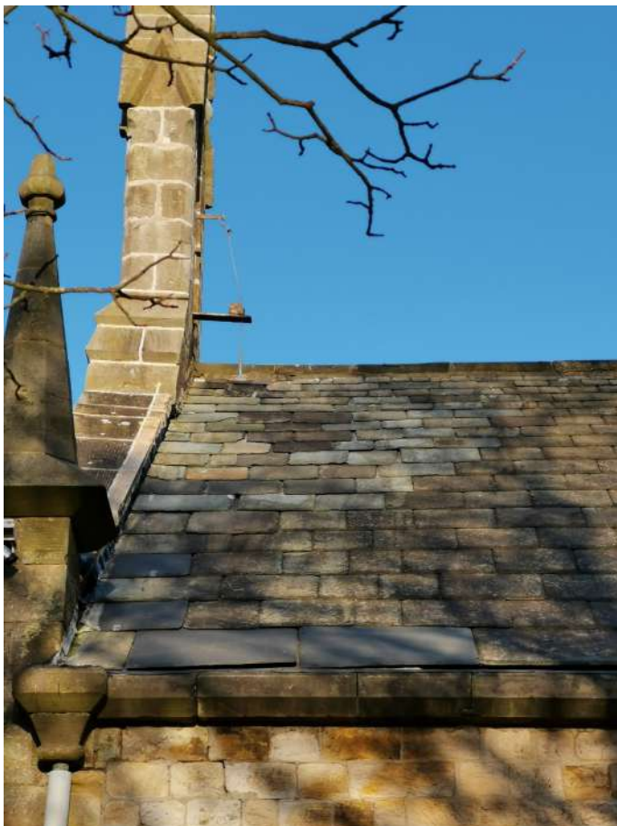
Newly patched slates to south-west nave
