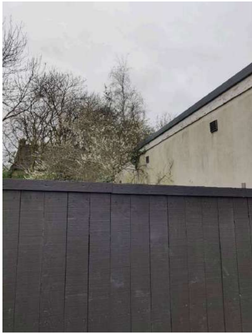
11. Redecorate timber eaves boards to E side of kitchen extension (rec. 2.04)
