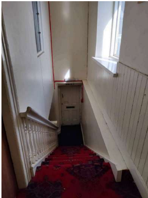
36. North end fire exit, looking down
