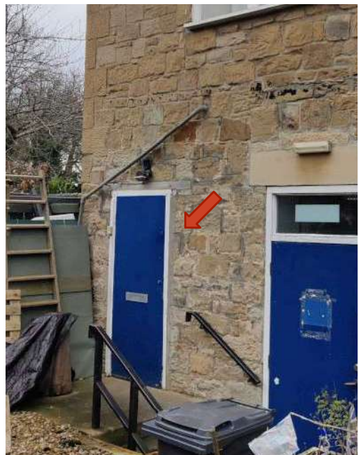
39. External view of north fire exit door
