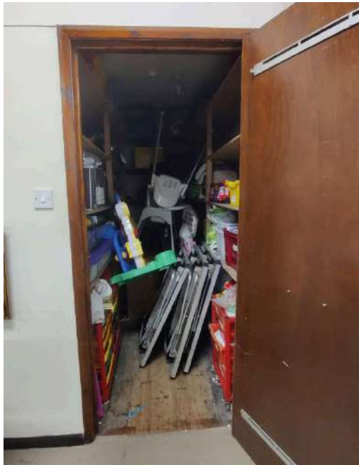
21. Storage room off the Community Room - reduce excess storage (rec 4.04)
