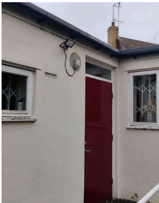
13. Redecorate kitchen windows and frames (rec. 3.01)
