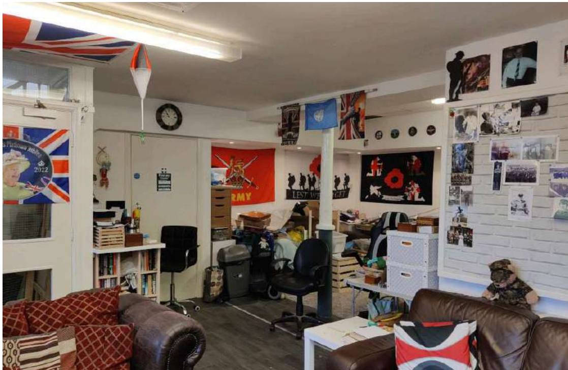
40. Lower ground floor main room seen from NW. Reduce excess storage (rec 4.04)
