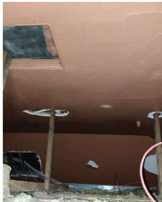
35. Void between St Hild and attic room
