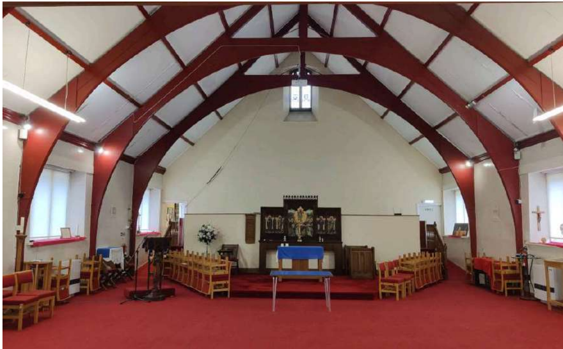
15. View of Nave. Consider replacing failing ceiling tape if funds allow (rec. 4.01)
