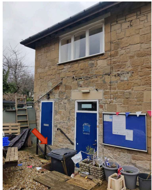
50. Remove the wheelie bin blocking the wheelchair access (rec 8.04)
