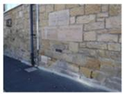
M Stonework is the same as the east though it is a little more worn at the footpath level. There are some open joints mostly in the middle below the memorial signs. There is a fillet of cement against the footpath and damp is clearly coming up, though there is little to be done here other than replace it in lime mortar if funds allow. There are some cement patches that look pretty poor.
