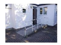
North side: Ramped and stepped area, the ramp provides disabled access down to the ground floor. Drainage grille at the bottom looks silted up and could do with being cleared out. Short brick retaining wall holding back a gravelled area.
