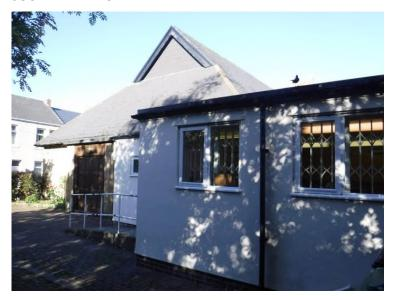
M Mixture of original building plus plastered rendered kitchen block, this has a Sarnafil type roof on, the middle section lobby has an old felt roof with some stone on the top of it.
