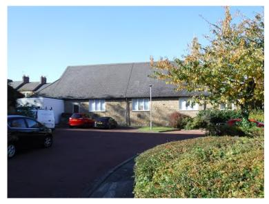
Rendered block extension to the south east corner, looks ok apart from the fascia board which needs decorating. The render has been brought right down to the ground and is staying put, it has been repaired in the past.
