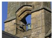
Stone belicote in good condition (probable repairs in c. 2010). Formed at the apex of the roof and creating a west window feature. The stonework is in good condition, some remedial pointing that doesn't quite match but no work to be done here. The window below it looks in good condition and the glass is clean, interestingly there is no protection on the glazing.
