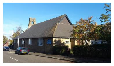
Gablet hipped roof formed of a ridge and four hips and these appear in good condition. The slating is in Eternit type fibre cement and these seem sound though there is moss collecting at the bottom edge of the slates that should be removed.
