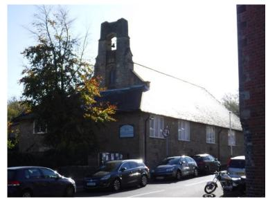
C Upper level is the apex of the Nave below the Bellcote that seems in fair condition. Lower level is the handcrafted operation, walls seem to be in fair condition, there has been some cement pointing. There is a crack to one of the lintels but this looks very old and it doesn't seem to be loading onto the window at all.
