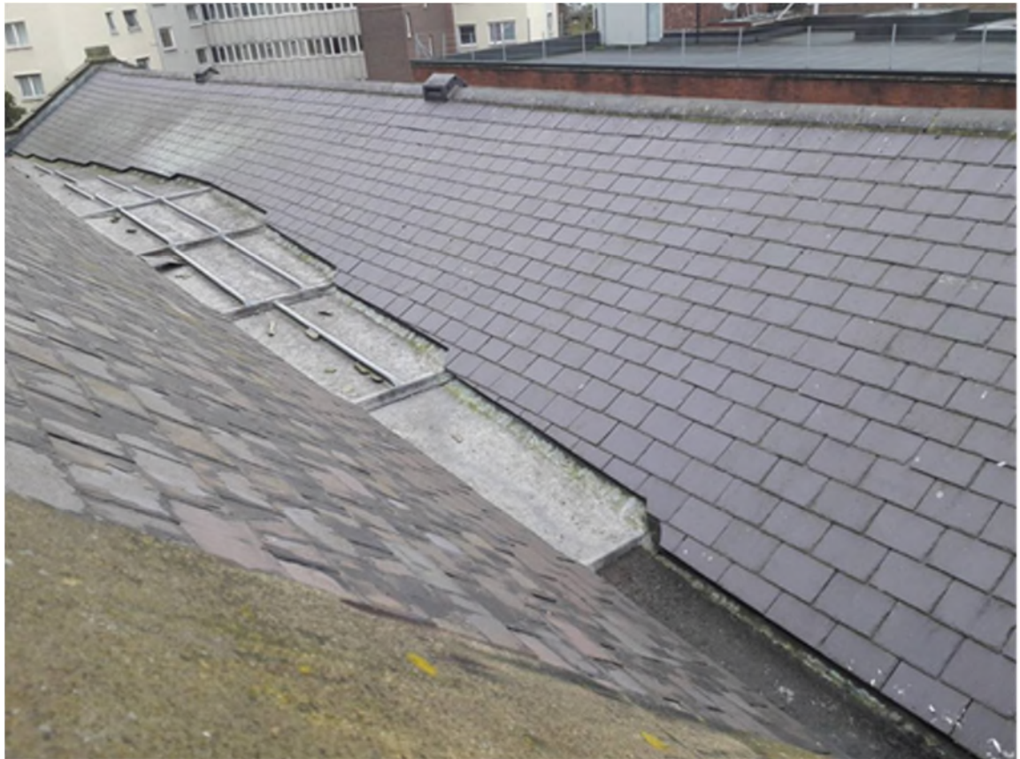
View towards Edmund. Note bits in the gutter
