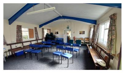
Open trussed roof with board panels with cover strips, slight rippling to one of the boards over the doorway.
