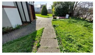
Within the boundary walls the area is mostly laid to grass with the principal path in concrete, in good condition. There is a secondary path to the hall in concrete paving slabs, slightly undulating and leading to a stone step up into the hall.
