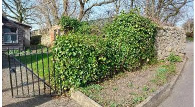
Holly tree is causing cracking to the wall and will only get worse and so it needs removal or the wall rebuilding to suit the tree growth.
