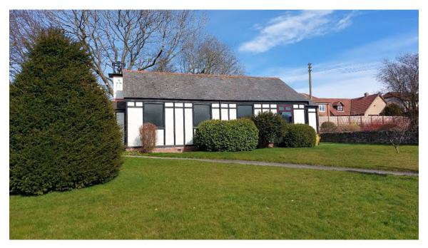
The church is an elementary prefabricated timber building dated from 1922 and originally intended as a temporary building. It has a four-bay nave with a smaller single bay chancel, a small vestry at the north side and a west porch. Cement tiles to the roof, and walls are clad in cement sheeting with timber cover strips. Inside the walls and ceiling are lined with soft wood tongue and groove boarding. Suspended timber floor.
