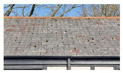
Red socketed clay dropping at the east end with the bedding generally sound, fibre board Eternit type slates in fair condition with some moss to it, significant amount on the north side.
