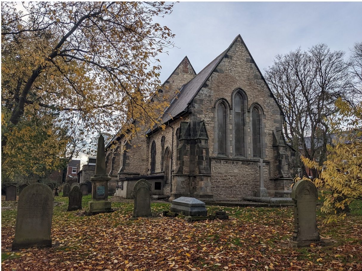
Fig. 3 | Church Photographs (3.1 + 3.2 Exterior)
