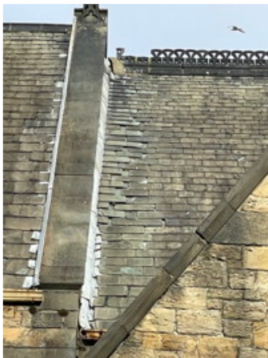
Chancel Roof South Elevation
