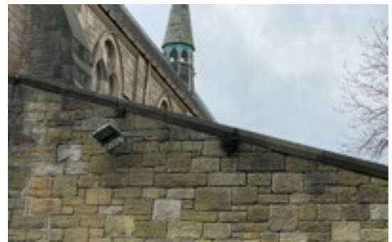
Plant growth at Vestry East Elevation
