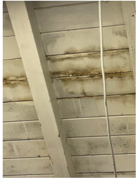
Vestry Store Ceiling
