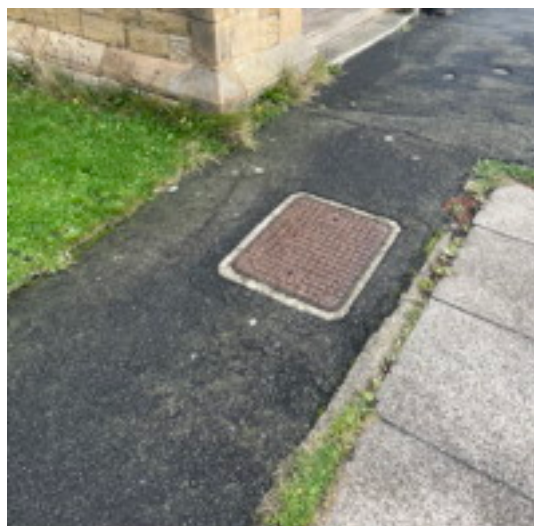
South Elevation Inspection Chamber
