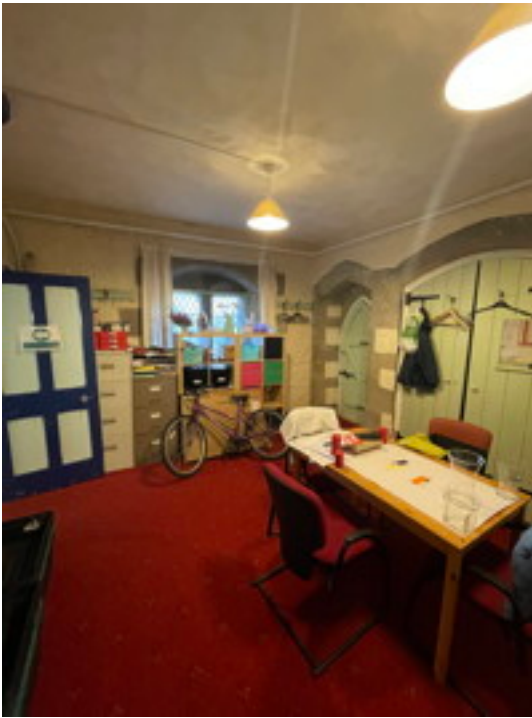
Vestry Looking East
