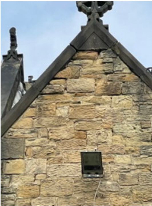
Eroding Stone to Organ Chamber Gable
