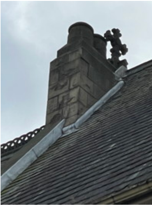
Chimney Nave East End
