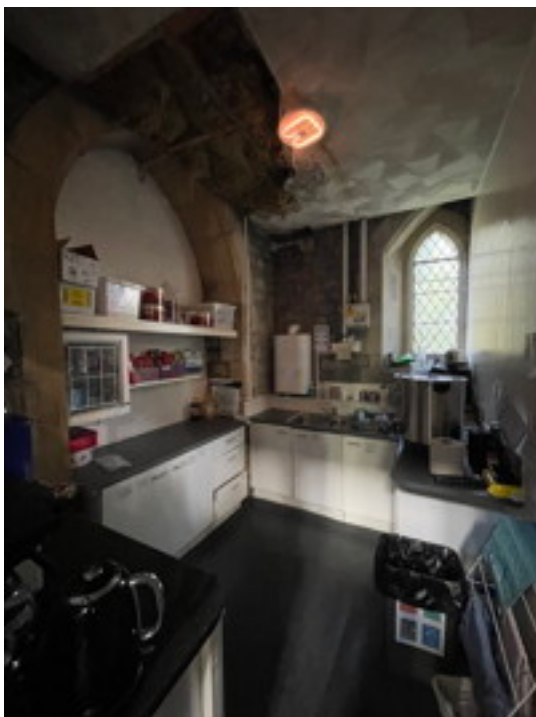
Kitchen Looking North
