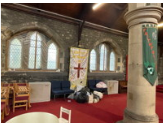
Plastic Sheeting to North Elevation Glazing Internally
