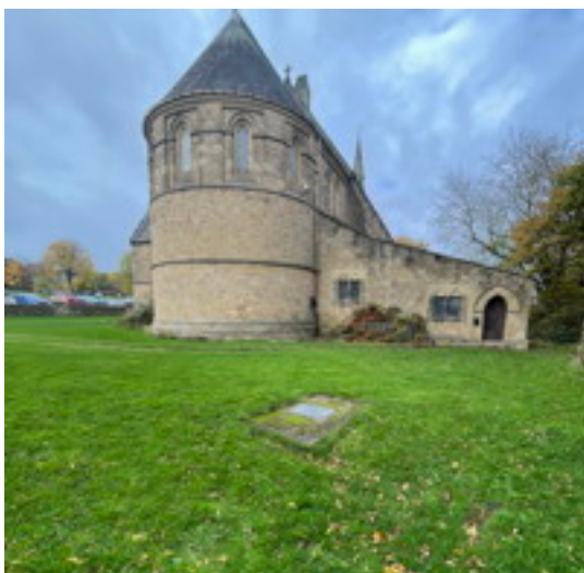
East Elevation Inspection Chamber
