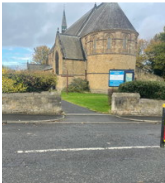
East Boundary Wall Entrance
