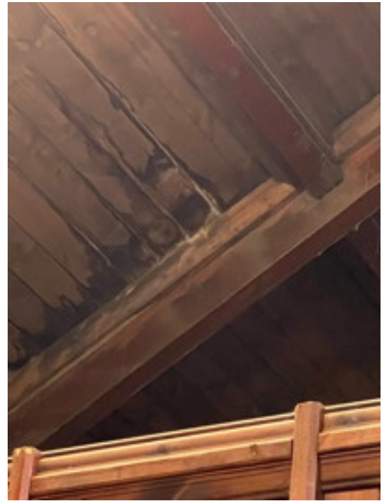
South Aisle Ceiling
