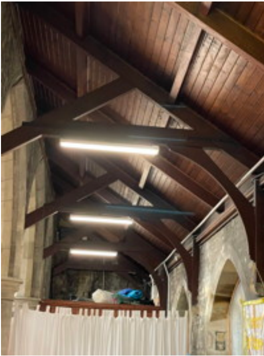
South Aisle Ceiling
