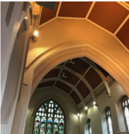
East End Ceiling
