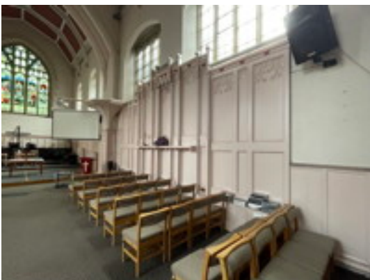
South Wall Panelling
