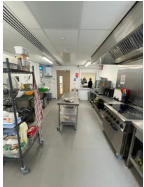
Multi-Purpose Room Kitchen Looking West
