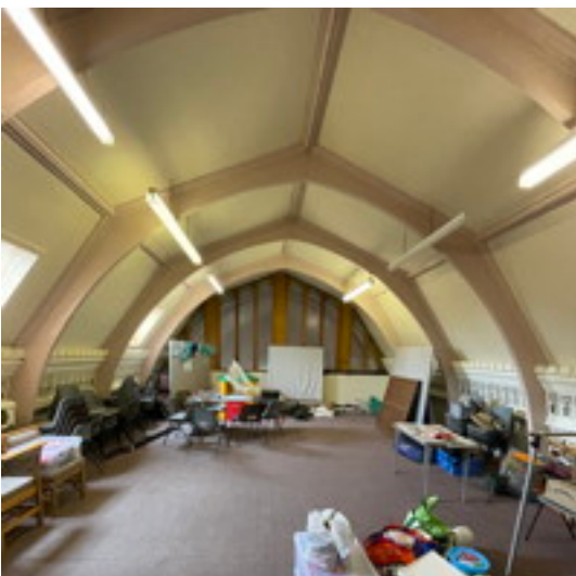
Second Floor Store Looking East
