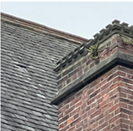
North Elevation Chimney
