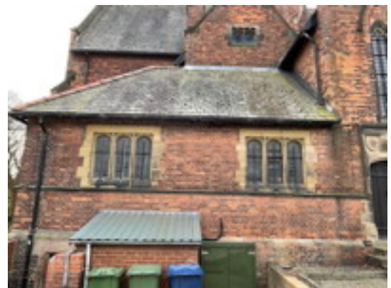
Vestry and Vestry Corridor Windows
