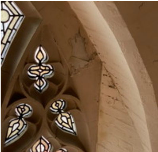
Second Floor Landing West Window
