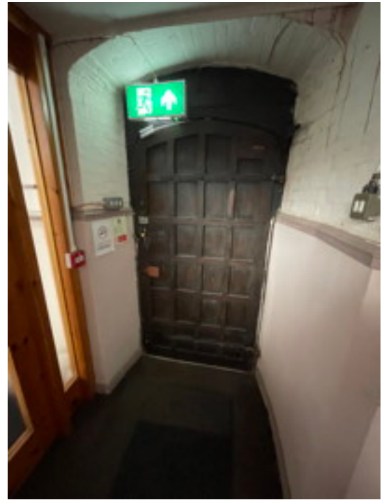
Vestry Lobby North Door
