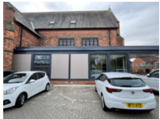
Cladding to New Extension
