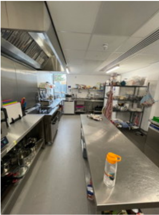
Multi-Purpose Room Kitchen Looking East
