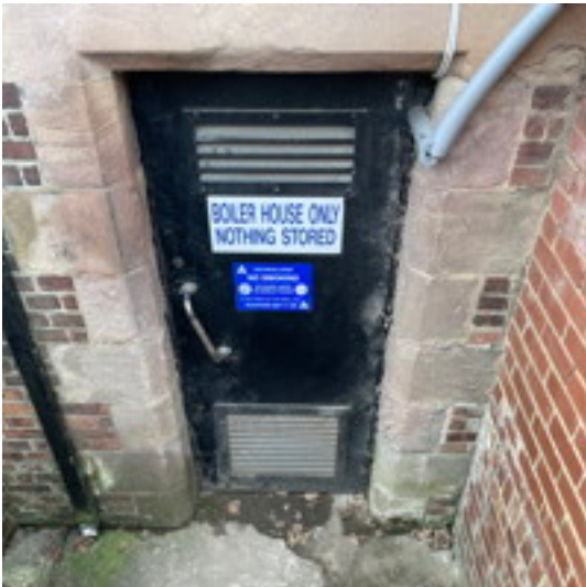
Boiler House Door
