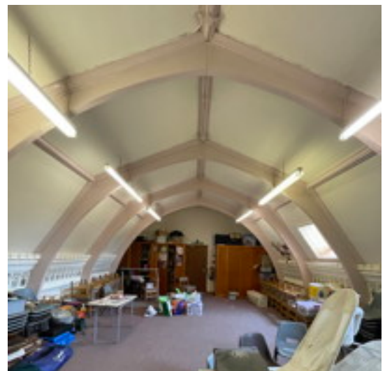
Second Floor Store Looking West
