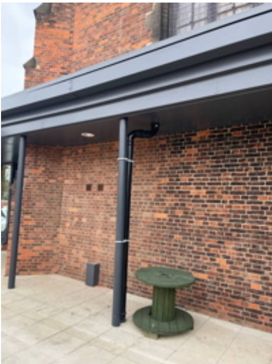
New Extension Roof Rainwater Pipe
