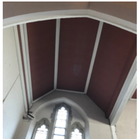
North Aisle Ceiling
