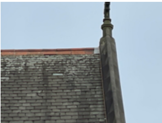
Slipped Slate South Elevation East End
