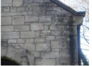
there is a crack running from the N kneeler down to the door head probably dropping in the corner, historical differential settlement, nothing too troublesome, a slight open joint at the bottom by the gulley and the arch has dropped fractionally in the past but is ok. Door within it is timber boarded locked shut not in use and the decoration is ok.
