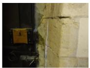
Poorly heated and rather forgotten area with not much in the way of appropriate shelving and fittings. It has a basic sink and hot water supply, electric heater and is carpeted over timber board with a bit of a floor vent showing. The bottom of the walls by the E end doorway salting rather, the E door is rather forgotten it is behind curtains and not used, it is draughty and it could do with improving if it means squeezing something into the gaps.
