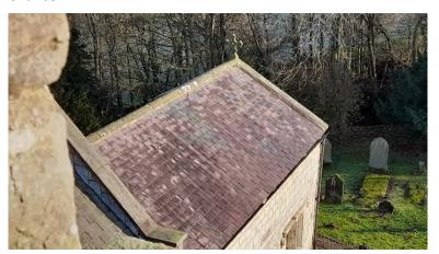
**South side** – Stone angled ridges laminating in places, ridge bedding looks just about ok, it might need a bit of a patch towards the E end. Welsh slate has been patched quite a bit in the past, it is fair condition.
