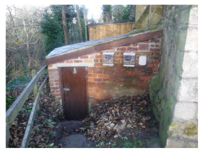
Elementary lean to brick structure to provide a boiler room. The steps down are coming apart and need repair.
