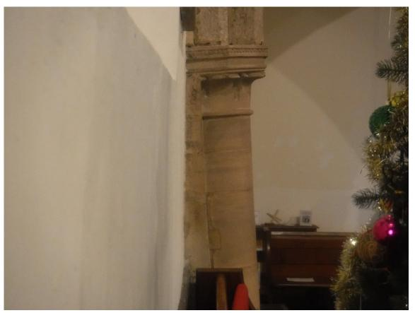
There is some distortion to the final arch at the W side on both arcades, however this is all historical. The plaster above the arcades at the W end on the N side shows that there is a shear crack up there but again this is just a minor problem probably superficial hairline crack. All of the arcades are sound as is the chancel arch, there is no cracking there. The tower is solid and in good condition.
