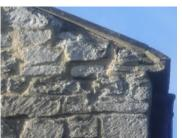
**East side** – Walling is ok apart from a few open joints at the bottom. Large three light tracery window, pictorial glass, historic crack at the apex and slight open joint which should be filled and mullions are generally ok. Above that is a small square hole in the gable apex, is that a perch has it got protection behind?
