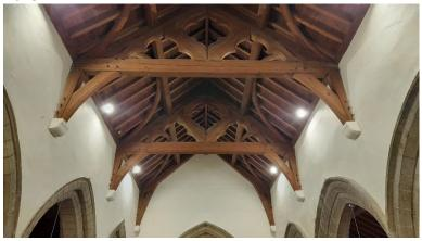
Three large sized decorative softwood trusses with cusping to struts, curved wind braces to purlins, rafters and horizontal sarking boards. All exposed and attractive but hard to see details against the downlights. No obvious defects.
