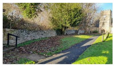
Southern end – Some rudimentary timber fencing leading down to the boiler room and as we head S it is beginning to go over where there is some older and close to the cottage wall which is made up of random stonework with terracotta round coping that has all been patched up in cement in the past, not brilliant condition. Is this the cottages or the churches responsibility? This then terminates by the cottage where there is a small timber w.c. which doesn't have a light inside it.
