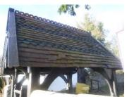
Timber lych gate which is in fairly good condition though there are some slipped slates.
