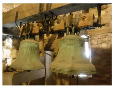
Two bells in the tower, dated 1664- 'Sol Deo Gloria' (Glory to God alone) and 1694- 'Deo Gloria', these bells are tolled. They are hung from timber headstocks with painted metalwork suspended from a large E to W beam. Bells are chimed by rope and leavers stapled to the headstocks and there is also a hand chimed hammer. The clappers are eroding the sound bow and it might be wise to have these turned if funds allowed, or checked over by the DAC bells advisor.
