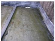
Loose slab tops to the murlons. Pointing to the flashing out in places but it is firm, hatch could do with a hinge on it, better grabrailing, another two in fact as you exit is required. Lightning conductor has four terminals just made of the straps and one downtape. Render inside on the masonry is all sound, dirt in the top of the parapet gutter.
