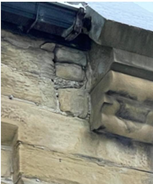
**South elevation east end open joints**
