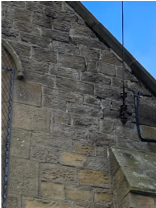
**Chancel east elevation north side open joints**
