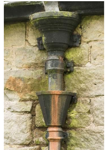
1.4 Stains indicate pipe is blocked
