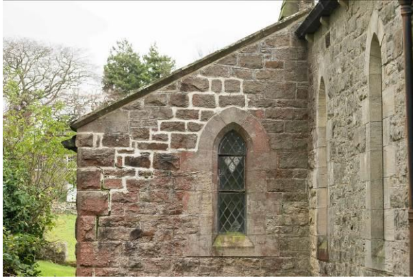
4.1 Recent repointing to Vestry west wall
