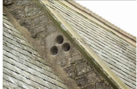
1.2 Nave roof void vent
