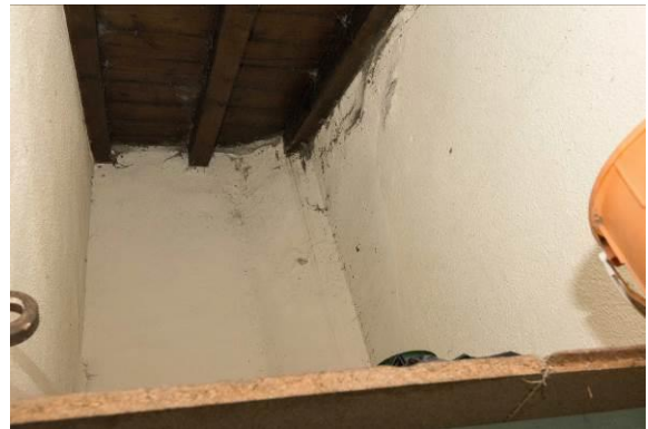
5.10 Roof structure above vestry lobby
