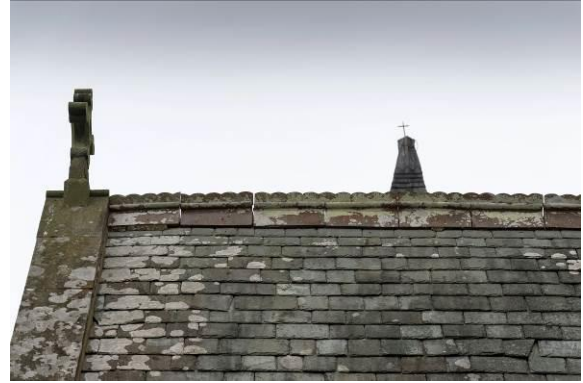
3.4 Ridge tiles have lost their mortar
