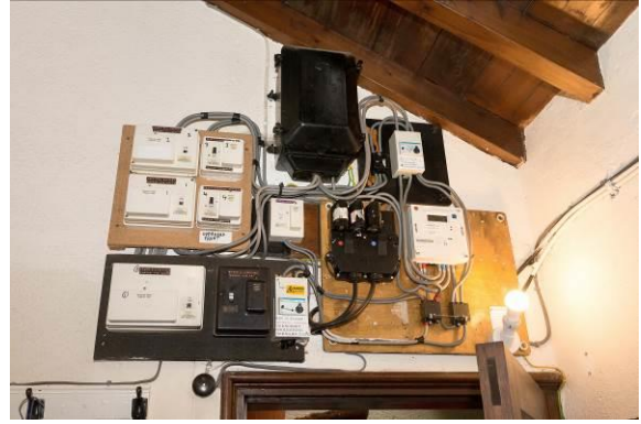
5.8 Electric meter panels
