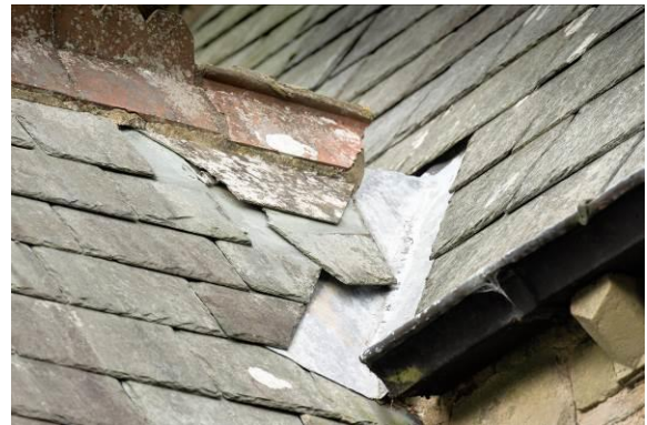
3.5 Slipped slates at valley gutter
