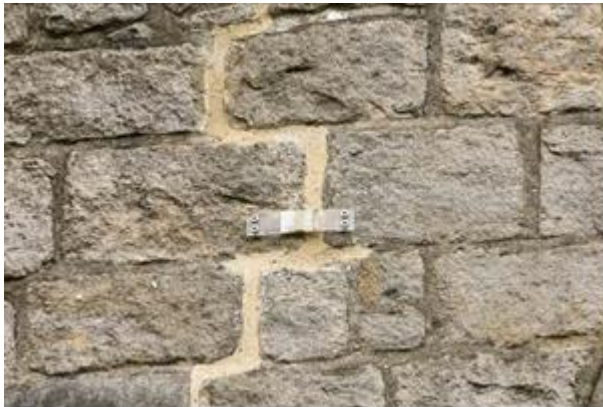
4.2 Vertical crack in the west gable
