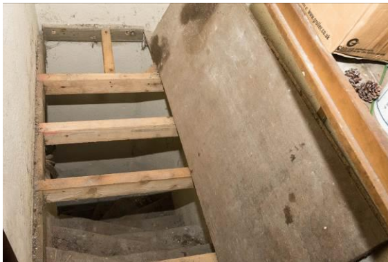
5.9 Infill to basement stair
