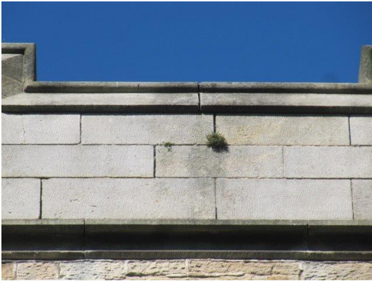
Open joints, cracking and vegetation growth to Tower parapet
