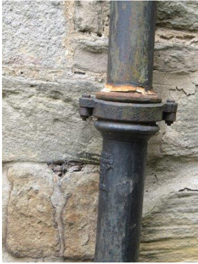
Rusty downpipe with damaged sealant to joint
