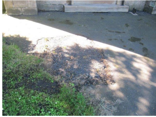
Failed patch to main tarmac path
