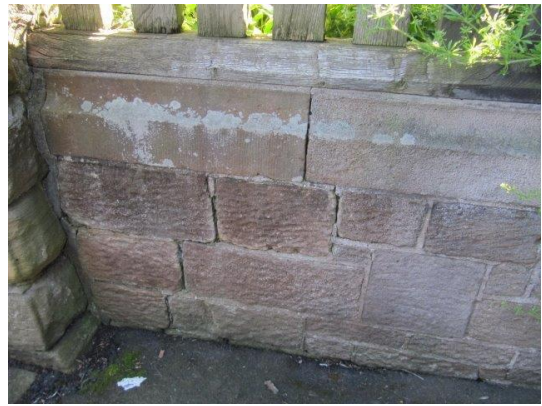
Cracking to wall of lych gate
