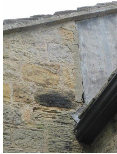
Failing mortar to side of lead on East gable of the Organ Chamber
