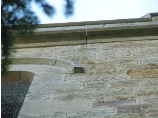
Open joints to string course and in section of wall below the parapet on the tower
