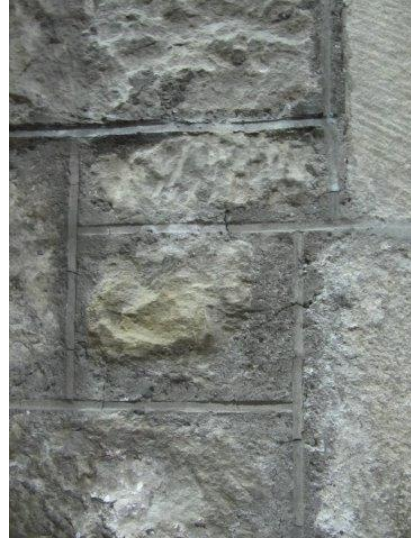
Hairline cracking through mortar to West Wall of Nave
