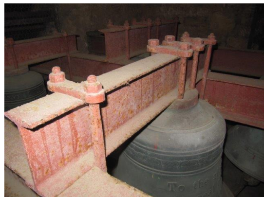
Rust to metalwork supporting bells
