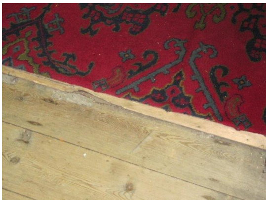
Loose and damaged timber edging near font and cut/damaged boards to East of Nave
