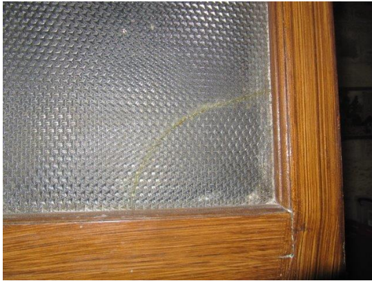
Repair to cracked glazing of vestry door
