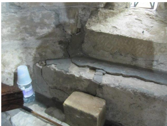
Cracking and failed mortar repair to W9 on South wall of Chancel
