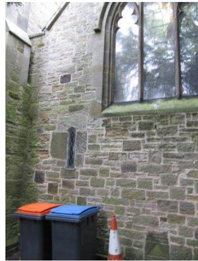
Green algae to corner between tower and West wall of the Nave
