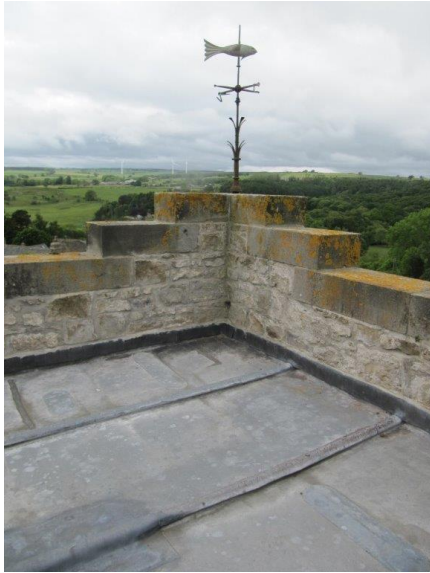
Previous patching to lead of tower roof
