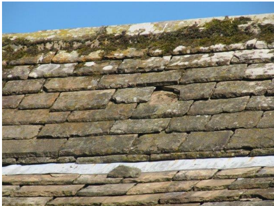
Cracked slates on Nave and vestry roofs
