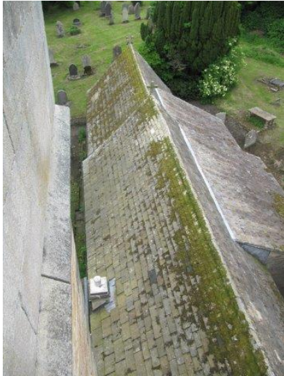
Views of the Nave roof from the tower
