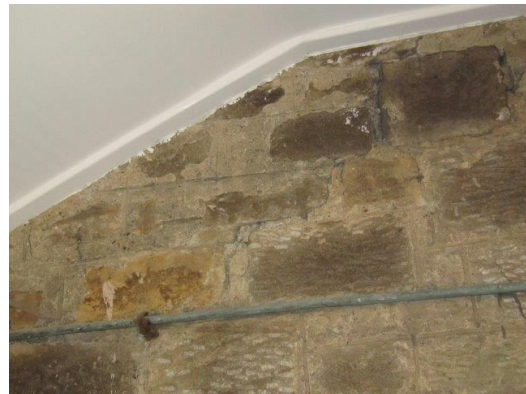
Cracking to East wall of boiler house
