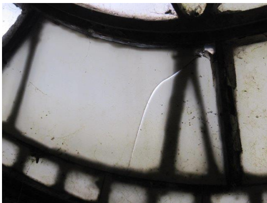
Cracked glazing to clock face
