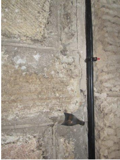
Cracking to North West corner of Nave
