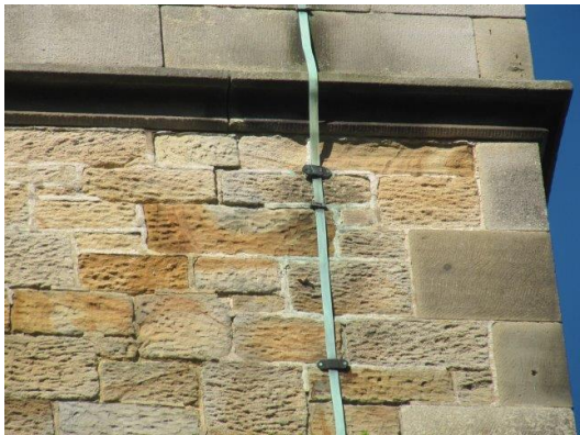
Open joints to string course and in section of wall below the parapet on the tower
