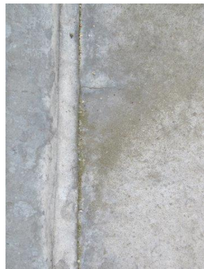
Deformed lead to rolls and cracking to lead bay on tower roof
