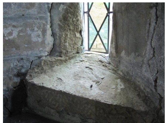
Cracking and failed mortar repair to W9 on South wall of Chancel
