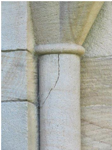
Cracking to pilaster of East Chancel window
