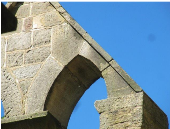
Open joint on east side of Bellcote
