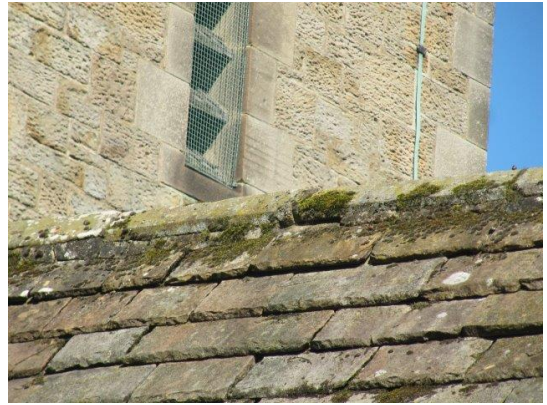
Missing bedding to ridge on Nave roof
