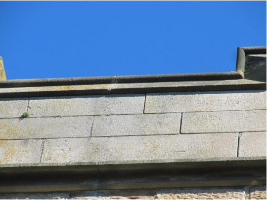
Open joints, cracking and vegetation growth to Tower parapet
