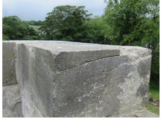
Cracked and loose stone to tower parapet
