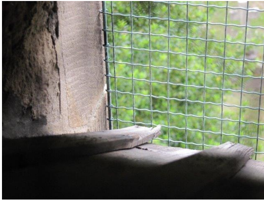
Damage to louvres/cover strips
