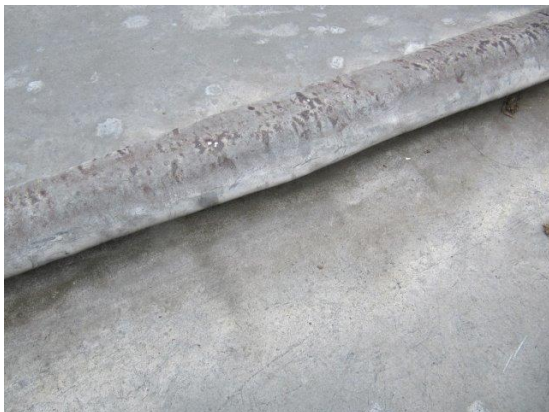
Deformed lead to rolls and cracking to lead bay on tower roof
