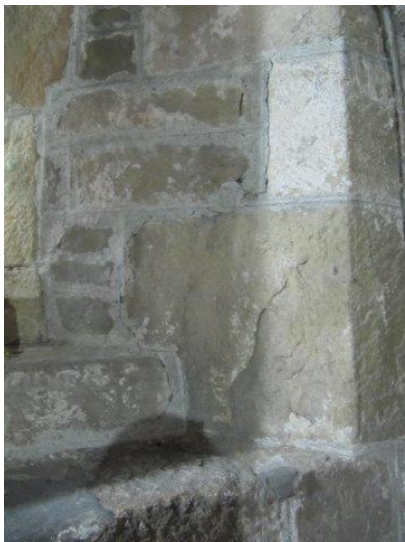
Cracking to window on North wall of Chancel
