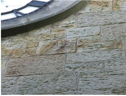
Cracking below the West (left) and North (right) clock faces
