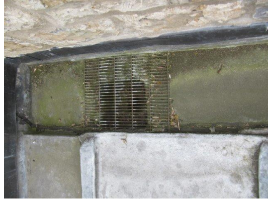
Gutter guard traps debris
