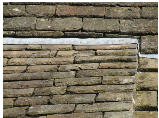
Missing bedding to ridge on Nave roof
