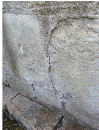
Cracking to mortar between larger stones on East wall of the Chancel
