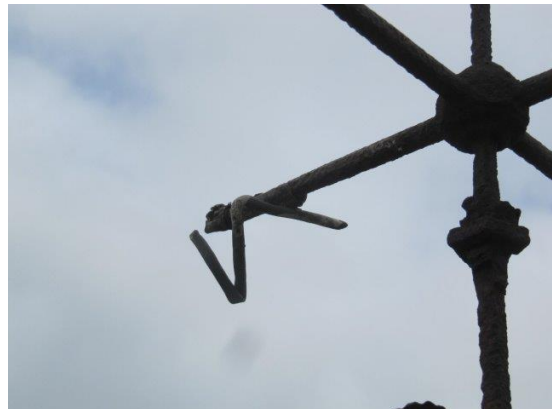
Rusting metalwork and damaged and loose compass point to weathervane
