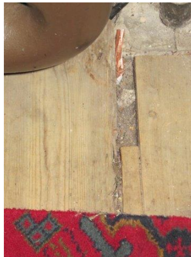
Loose and damaged timber edging near font and cut/damaged boards to East of Nave
