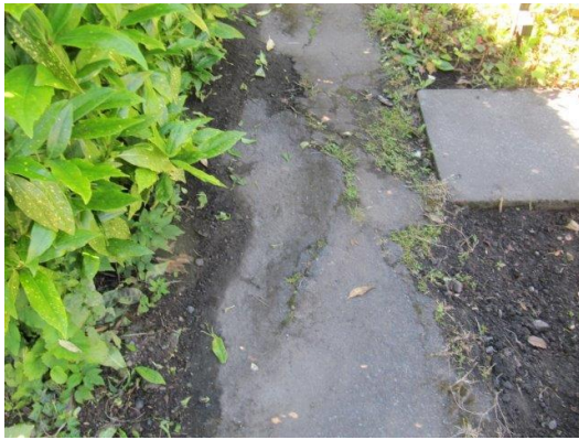
Uneven and damaged tarmac path To Garden of Remembrance
