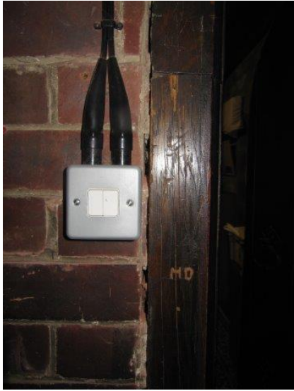
Cracking around door frame to organ chamber
