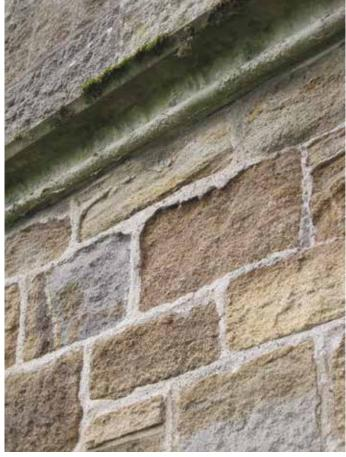
Hard and impermeable cement pointing causes accelerated decay of adjacent soft sandstone
