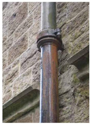
Rusting and algae on downpipes is sign of leakage from joints, suggesting that the pipe is blocked with debris.
