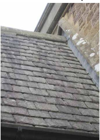
The Porch roof is in good condition. The ridge requires re-pointing in lime mortar
