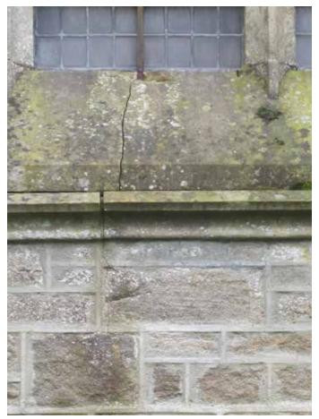
West window: cill split by corroding ferrementa, harmful and ugly cement pointing below
