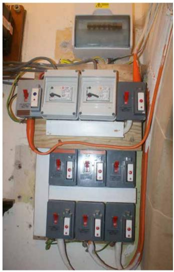
The electrical installation is tidy and appears to be in good order. Test and inspection is overdue, but in hand
