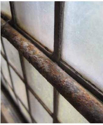
Steel saddle bars are corroding and should be cleaned off, rust-treated, and painted
