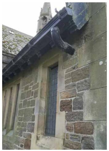
The Vestry east gutter return into the building - a poor detail. Fit a new downpipe and gully below
