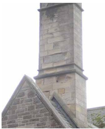
Some of the chimney stones are heavily eroded, and cement repairs are hastening the stone decay
