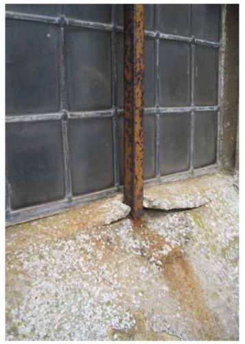
The corroding external ferrementa has split many of the window cills
