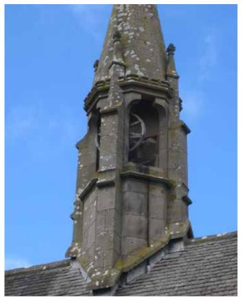
The fleche is very well constructed. The bell mechanisms have suffered from weathering and timber decay
