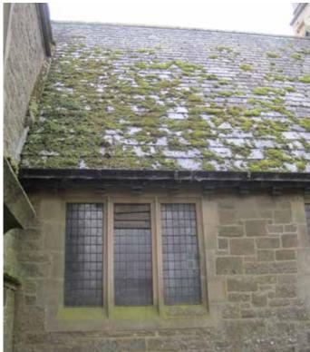
Moss build up on all roofs should be carefully cleared off. Moss prevents the slates from drying out, encouraging frost damage. It also blocks gutters and downpipes.
