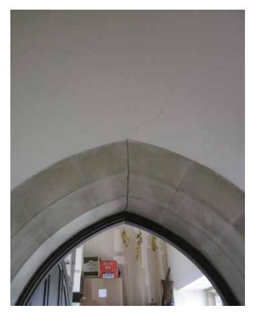
Cracking to the head of the Vestry door
