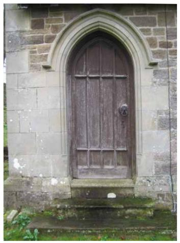
The Vestry door - the step is saturated due to a gutter leak above
