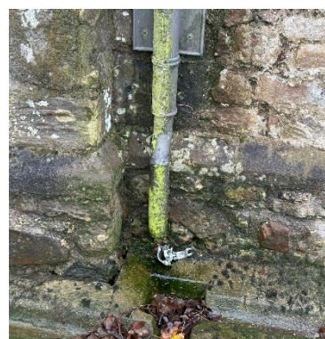
Figure 6 – downpipe short of gulley
