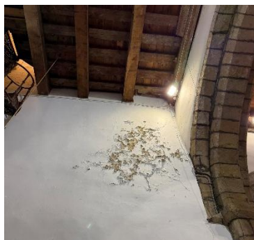
Figure 19 – damp patch to tower
