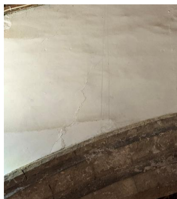
Figure 34- historic cracking at arch
