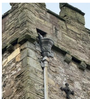
Figure 13 – Tower hopper outlet
