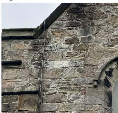
Figure 8 – Cracking at kneeler
