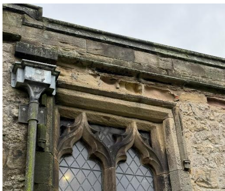
Figure 10 – N Aisle stone decay
