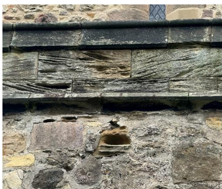
Figure 9 – S Aisle stone decay
