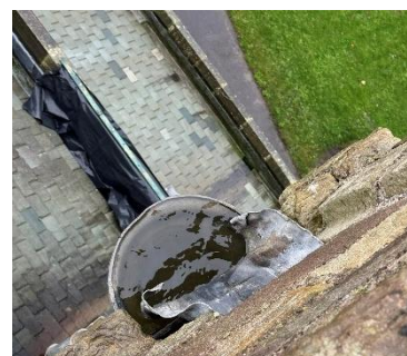
Figure 5 – Overflowing hopper at Tower
