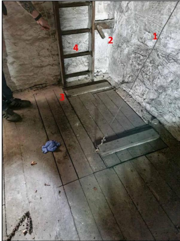
**MUFFLING CHAMBER COUNTER BALANCED HATCH**
