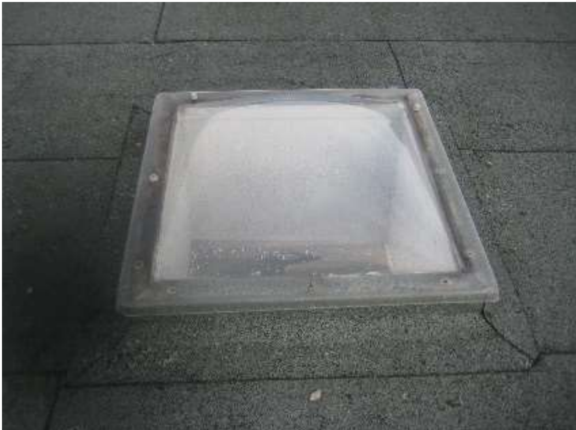
typical rooflight – missing fixings
