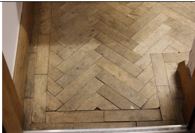
Loose wood block flooring
