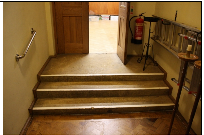
Bare & deteriorating concrete floor finish
