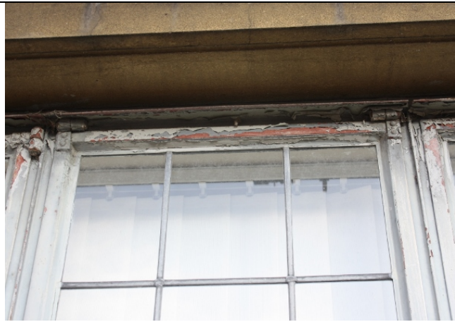
Flaking paint to metal windows
