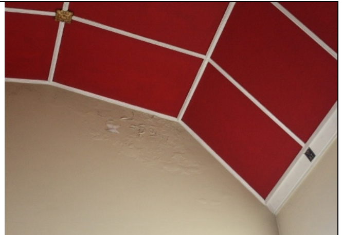
Chancel East wall – flaking paint through leak
