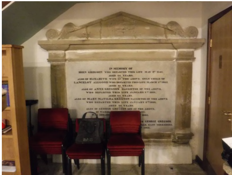
Below gallery, relocated Gregson memorial tablet which is a pedimented rectangular frame, this was in a previous position, there is some damp showing to it around its perimeter.
