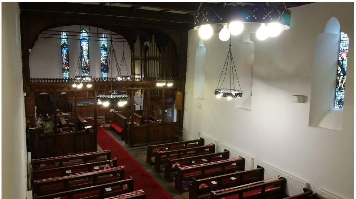
Interior: gutted and plastered. Panelled nave ceiling, shallow wagon roof to chancel; minimal wooden chancel screen.
