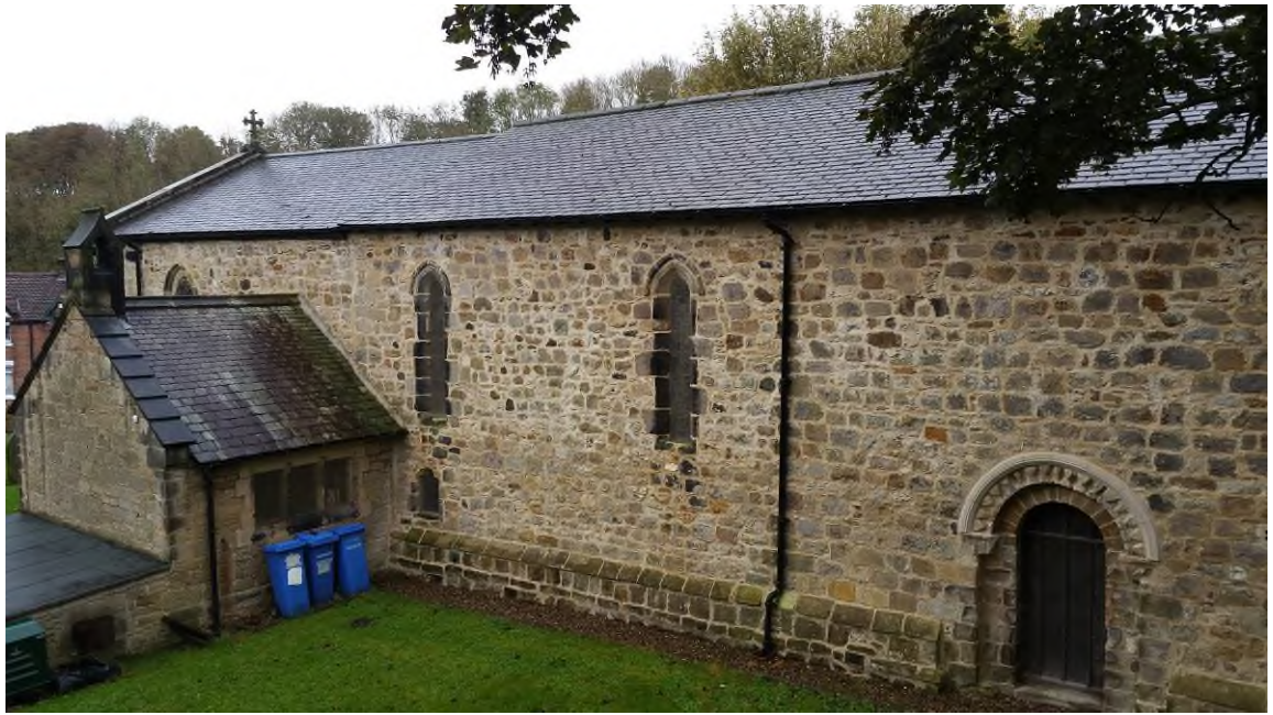
North wall has chamfered plinth and a late Romanesque doorway of 3 orders with chevron and worn scalloped capitals, shafts missing. Single tall lancet in west end and bellcote above.
