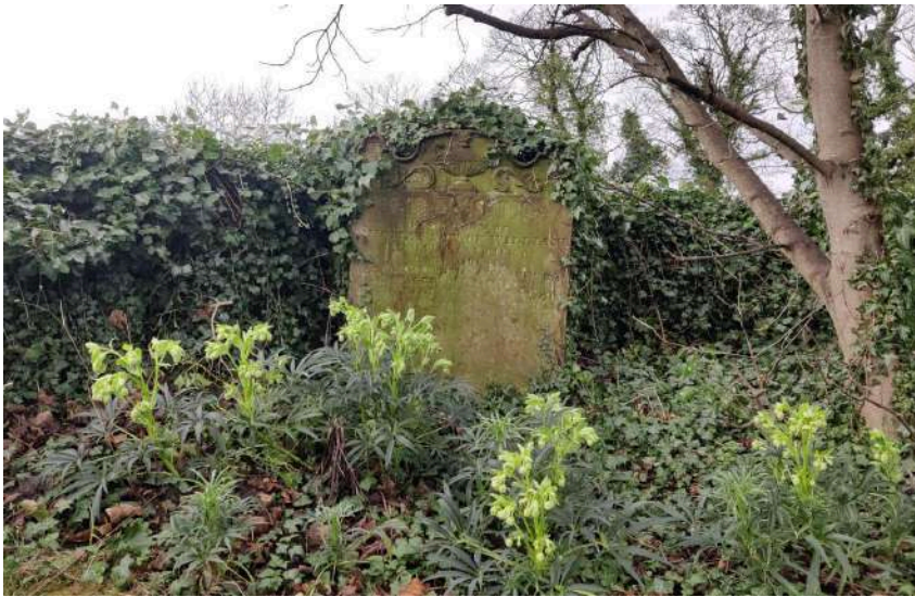
73. Corner of W and S boundary wall is overgrown
