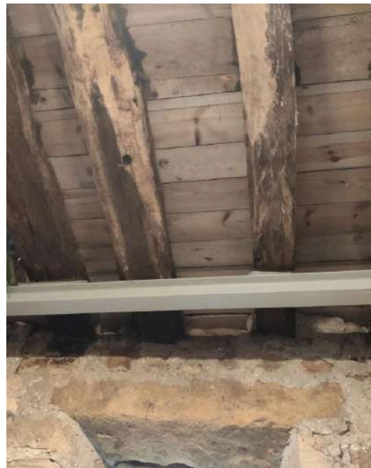
60. Tower first floor - new steel beam supporting decayed beam ends
