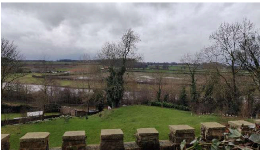
75. View over S boundary wall. The crenellated wall at the bottom of the photo is a separate retaining wall beyond the boundary wall.
