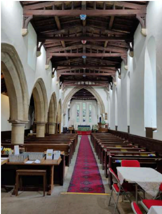
13. Nave looking East
