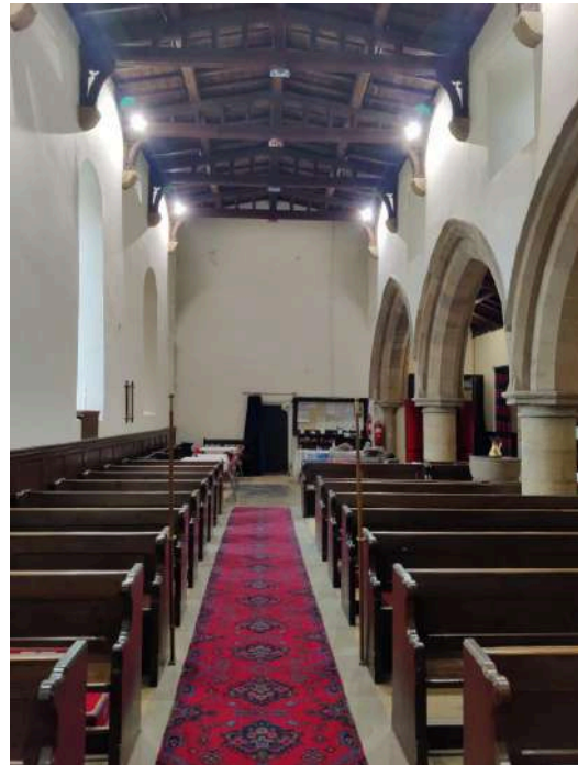
14. Nave looking West
