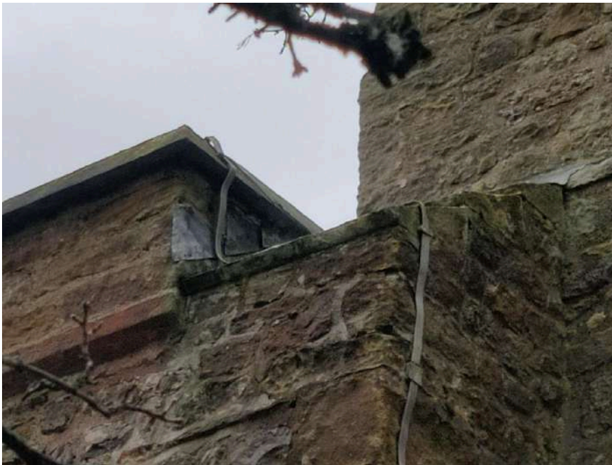
55. Close-up of exposed wall head at NW end of Nave.
