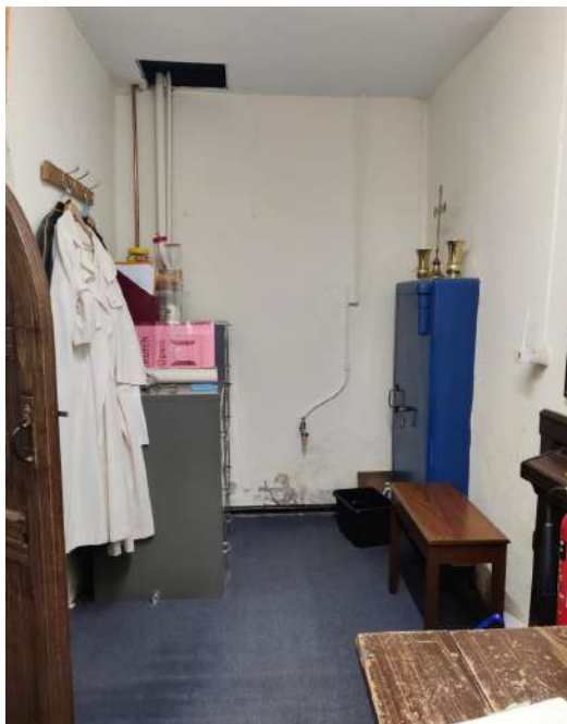
32. Vestry looking West and loft hatch
