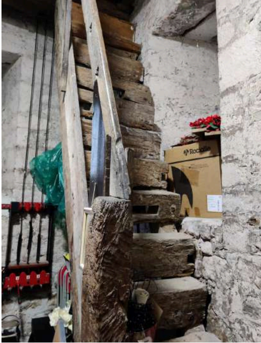
57. Tower ground floor, stair leading upwards
