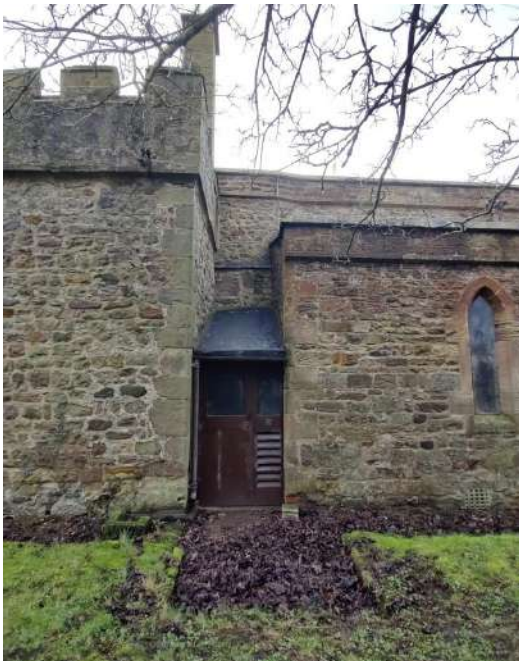
49. Boiler House between Vestry and North Aisle
