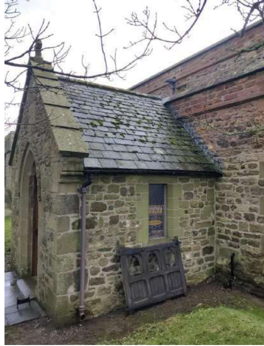
54. W elevation of North Porch, with temporarily stored gate from the Lychgate
