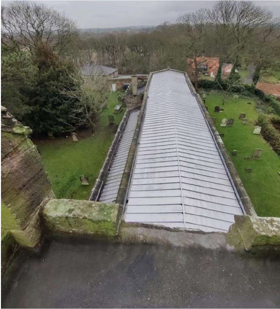
56. View onto Nave and Chancel roofs
