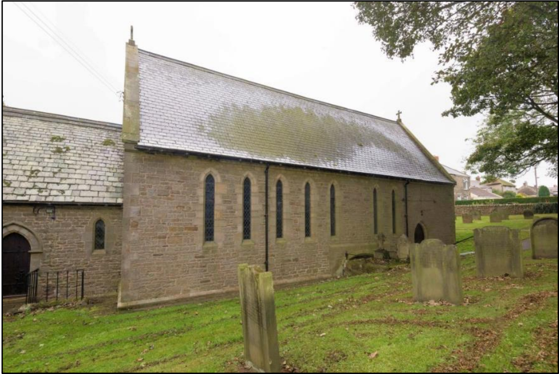
North Elevation: North Aisle
