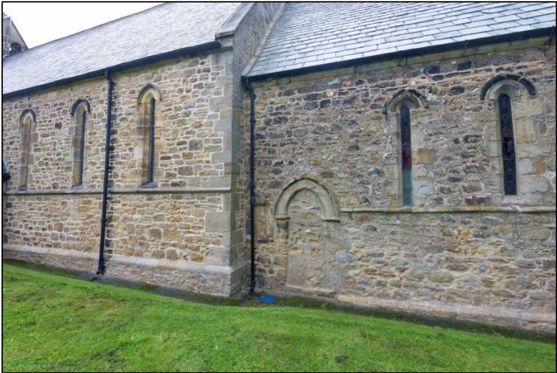
South Elevation: junction of nave and chancel, showing an infilled very early doorway
