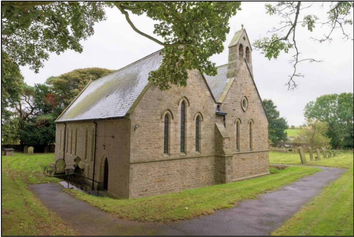
View from the northwest
